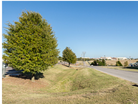
Landscaped Drainage Area
