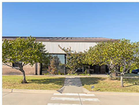
Sidewalk Accommodating Grade
