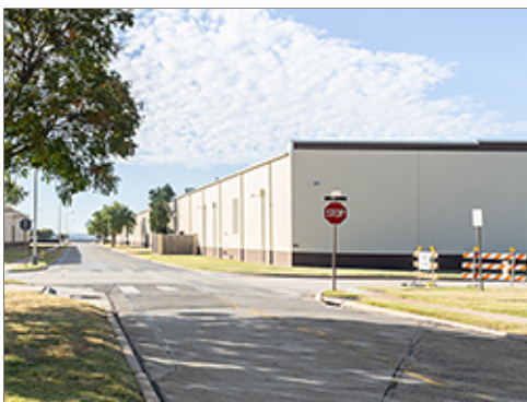
Local Street Adjacent to Group 3
