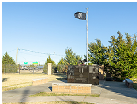
Concrete Paving at Memorial Plaza
