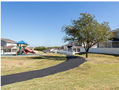
Asphalt Paving at Trail
