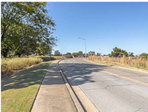
Attached Concrete Sidewalk
