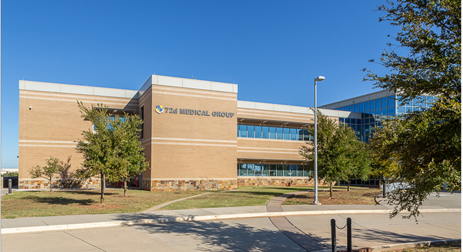
Stand-out Letters on Group 1 Facility
