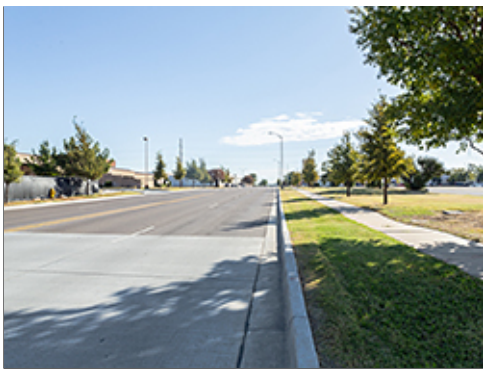
Concrete Paving at Intersection
