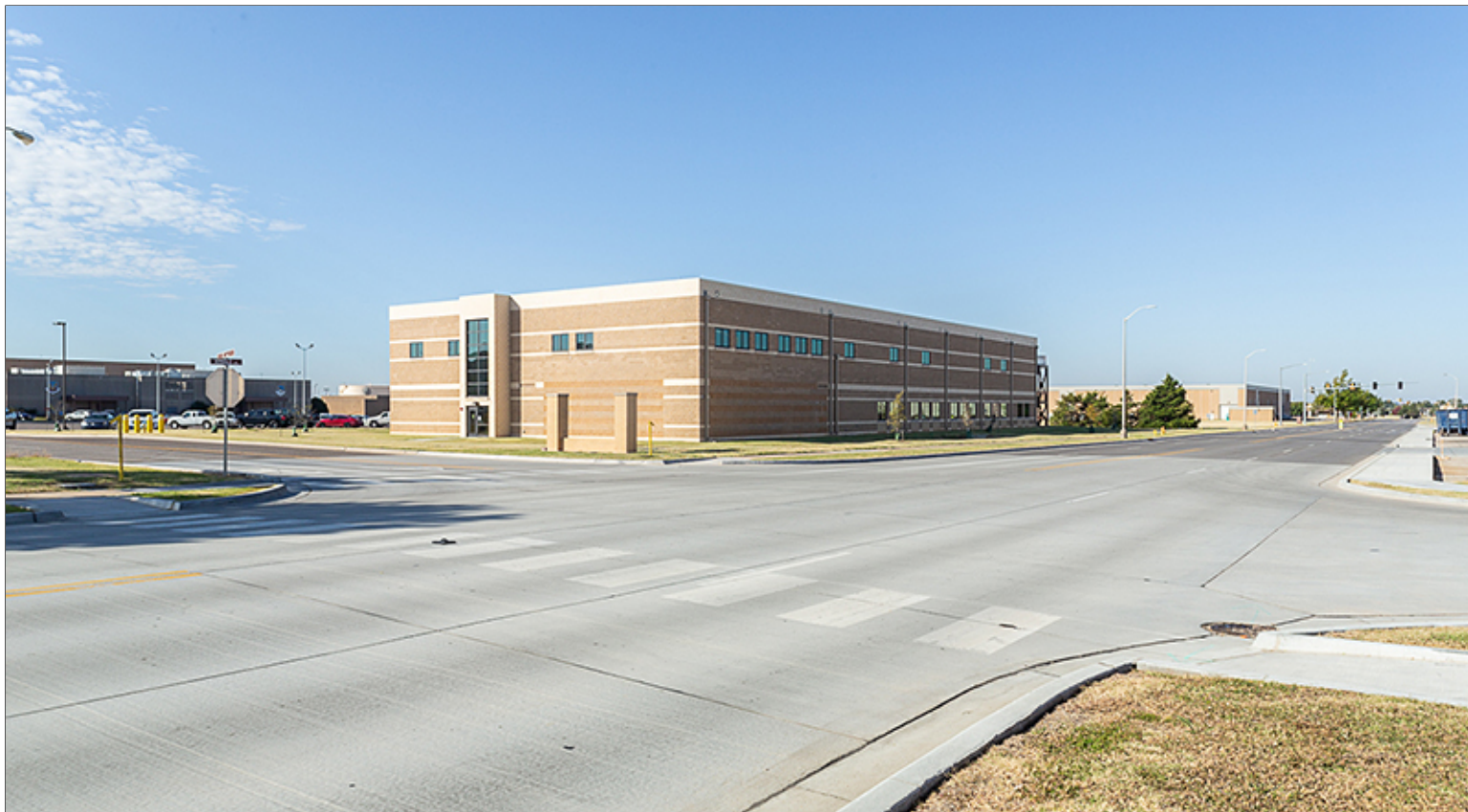
Intersection at Headquarters
