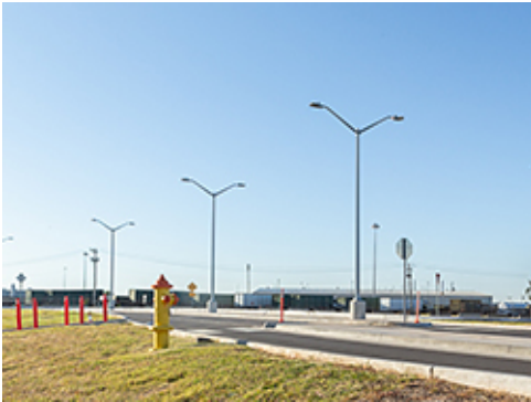
Dual Arm Cobra Head Fixtures
