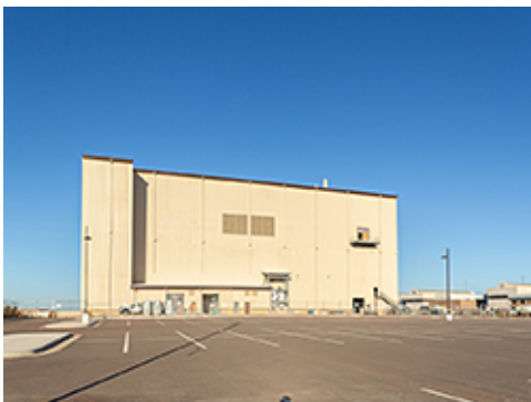
Buried Utility Lines in Group 3
