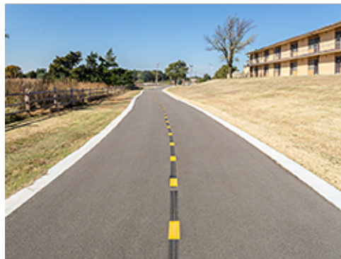
Asphalt Paving with Header Curb
