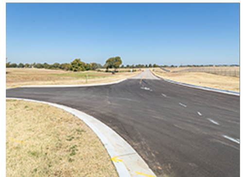
Asphalt Paving with Integral Curb and Gutter
