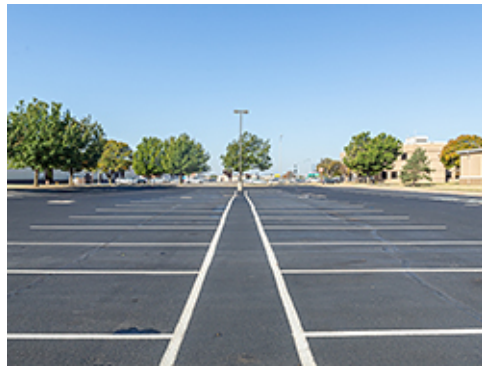
Asphalt Paving with White Striping
