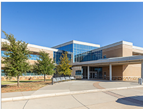
Decorative Concrete Entrance Plaza at Group 1
