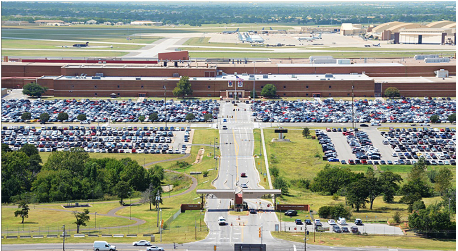
Installation Elements: Base-wide Infrastructure
