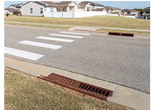
Coordinated Storm Drain Inlets
