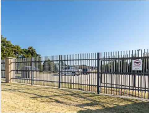
Brick and Metal Fencing at Group 1
