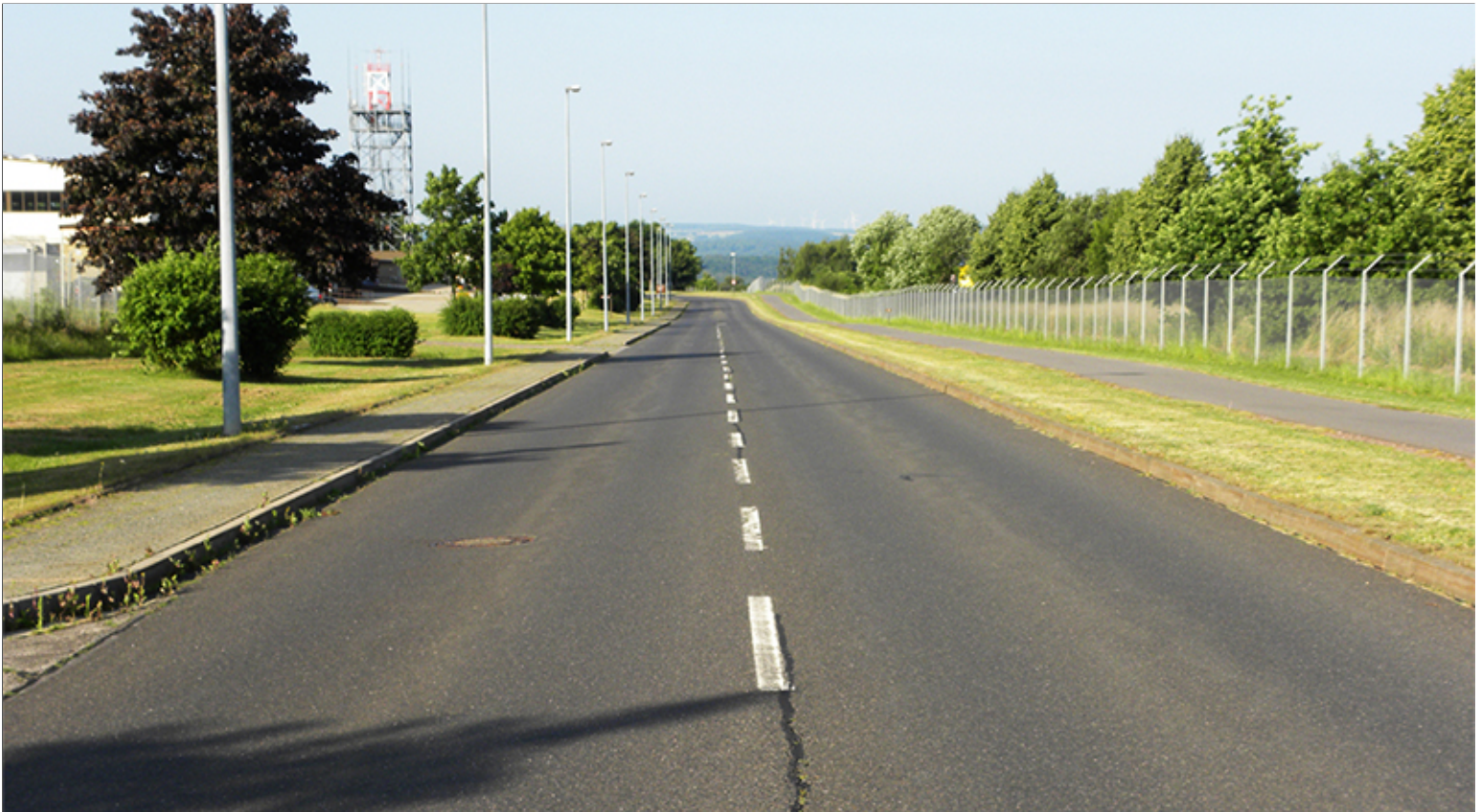
Travel Lane (a): 12' Median (b): 12' Curb and Gutter (c): 2' Sidewalk / Landscape (d): 12' Setback (f): Min. 35' or per ATFP
