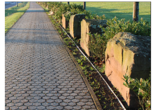
Rocks form Retaining Wall at Walk
