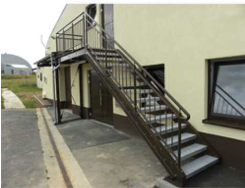
Exterior Stairway (Emergency Exit)
