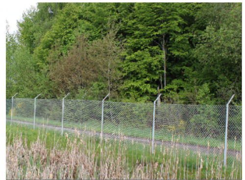
Security Fence near Housing
