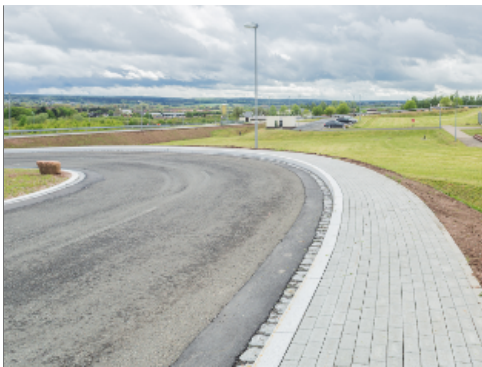
Gutter made of Pavers
