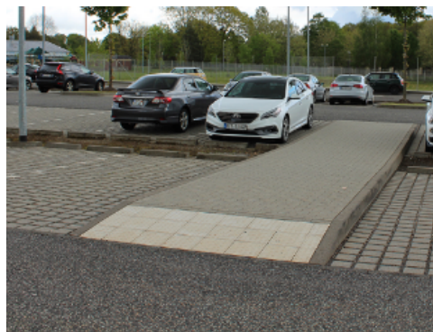
Ramp at Walkway in Parking Lot
