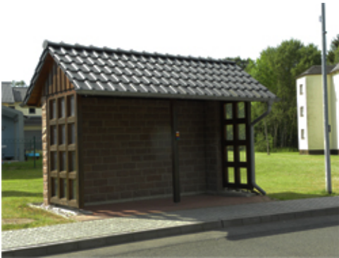
Fully Enclosed Bus Shelter
