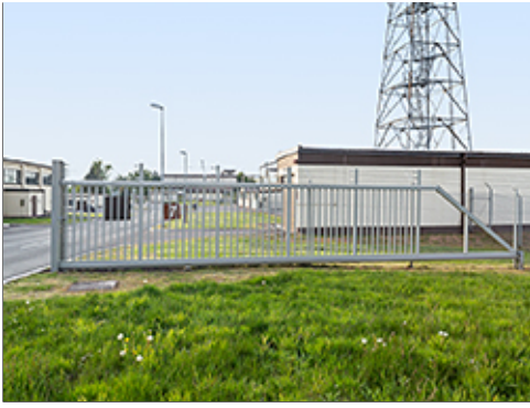
Sliding gate at Entry Control Facility
