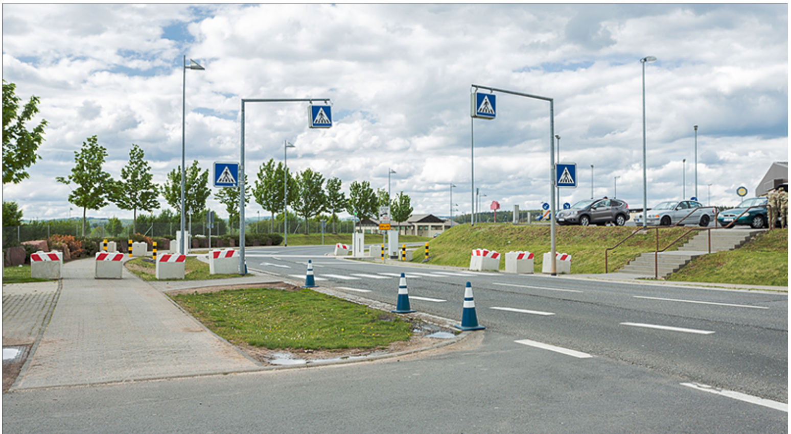
Road to Main Gate
