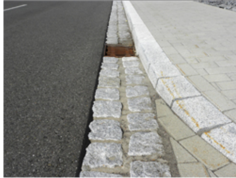
Curb with Gutter
