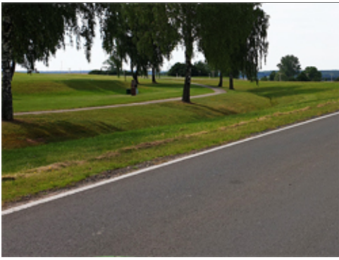
Trees and Grass next to Drainage Channel
