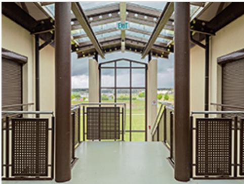
Stair Feature at Group 2 Dormitory
