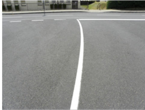
Striping at Intersection
