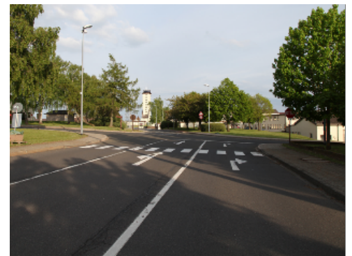
Streetlight at controlled Intersection
