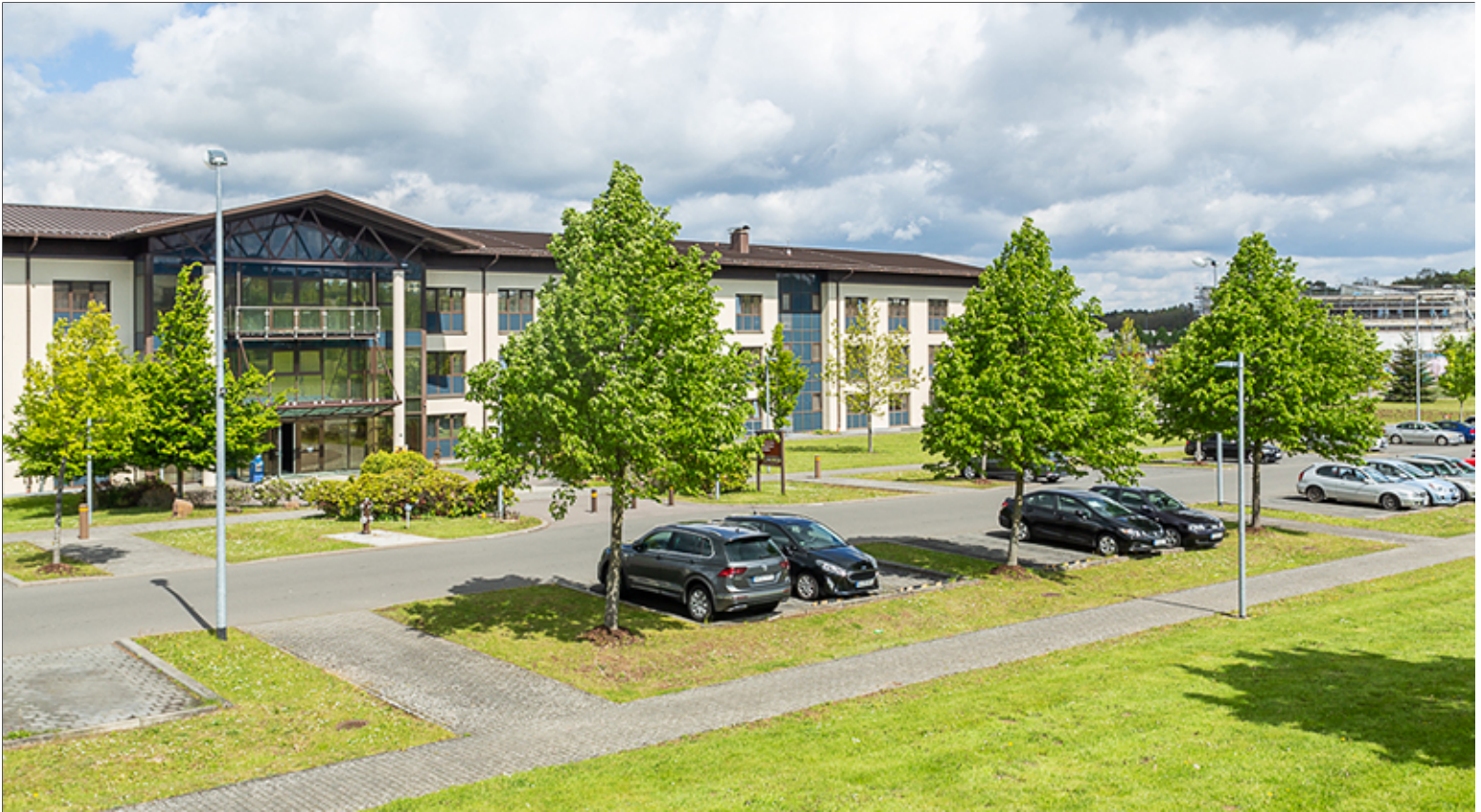
Parking near Building Entry
