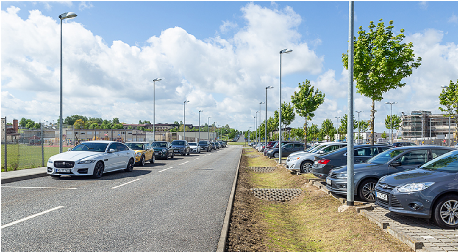
Drainage along Street
