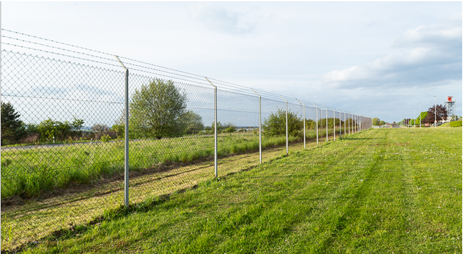
Chain Link Perimeter Fence
