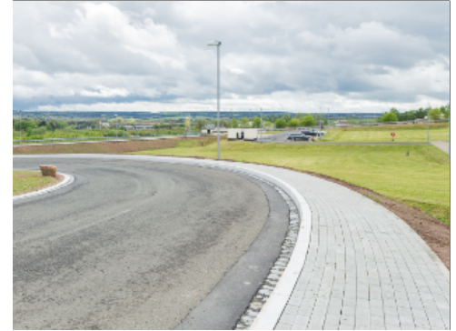
Gutter made of Pavers
