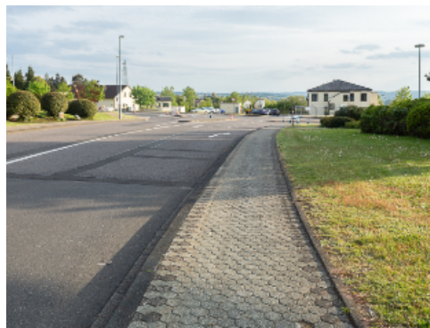
Sidewalk of Pavers
