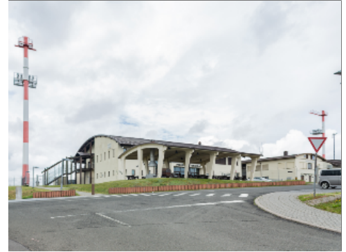
Intersection at Terminal
