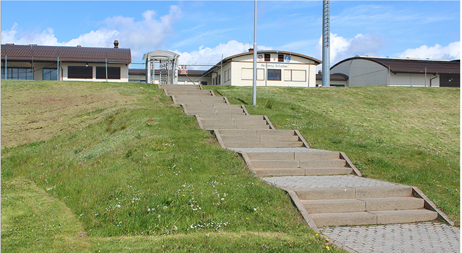
Stairs from Terminal to Parking
