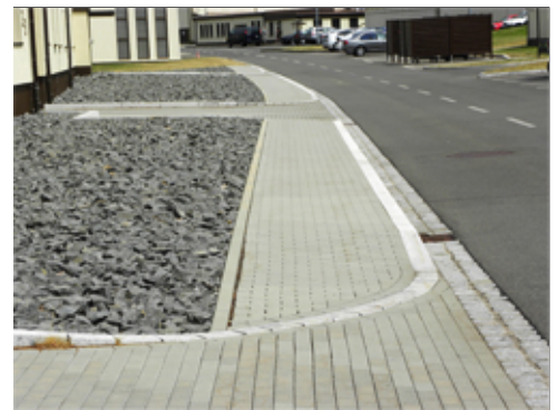
Sidewalk and Street
