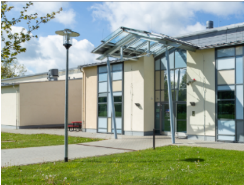
Light at Entry
