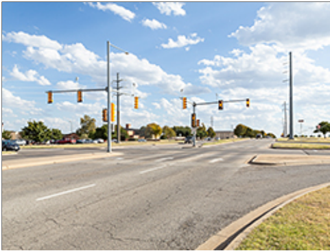
Traffic Signal at Arterial Intersection
