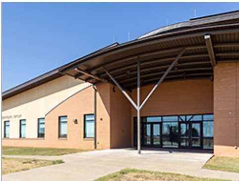
Concrete Paving at Entrance Plaza
