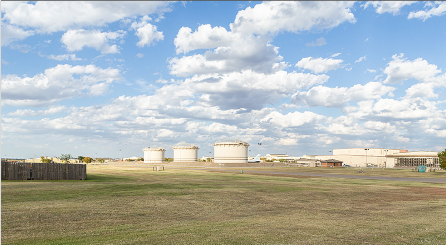
Open Space Buffer at Industrial Area
