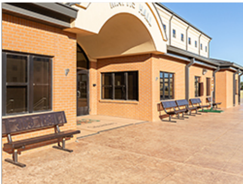
Colored Concrete at Group 2 Entrance
