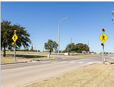
Pedestrian Crossing with Signs and Signals
