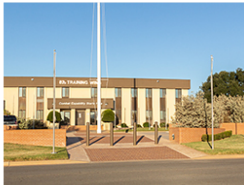
Unit Pavers at Flagpole Plaza
