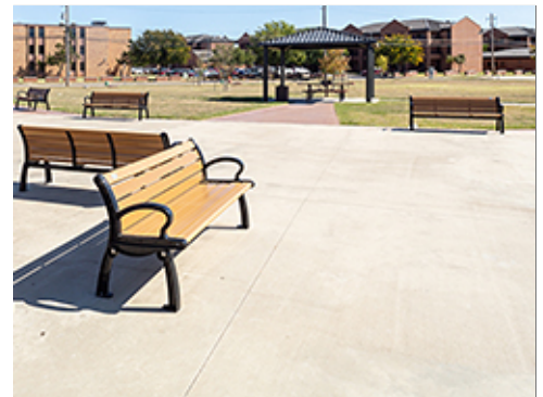
Concrete Paving at Recreational Area
