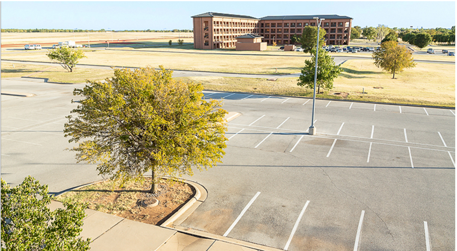
Standard Bituminous Paving and White Striping
