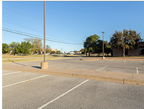
Raised Concrete Median
