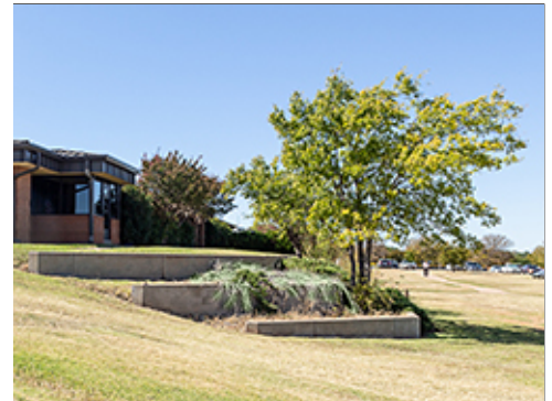
Use of Grading to Capture Rainwater
