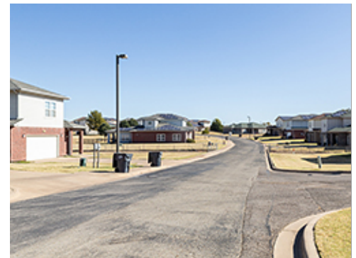
Buried Power Lines in Group 4
