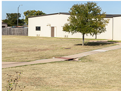
Grass Swale and Culvert at Group 3
