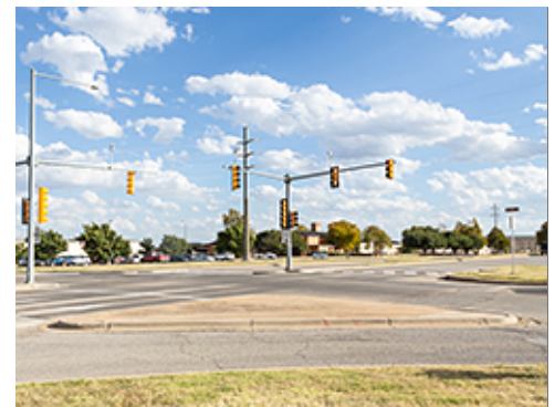
Concrete Island at Merge Lane
