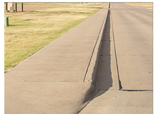
Transition at Curb Ramp
