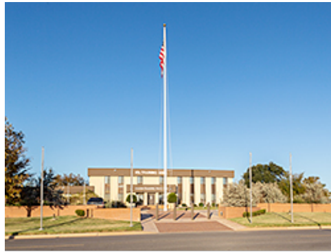
Installation Flag Pole
