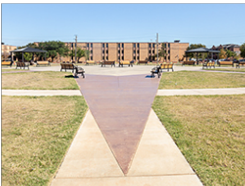
Colored Concrete Paving at Group 2
