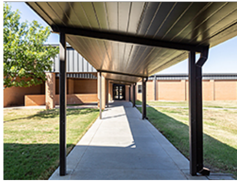
Shading Canopy Connecting Facilities
