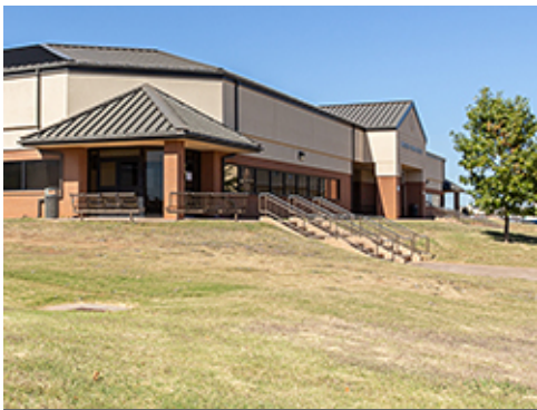
Site Stair at Entrance
