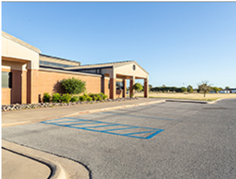
Blue Striping at Accessible Parking
