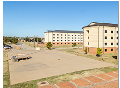
Concrete Paving at Group 2 Assembly Area
