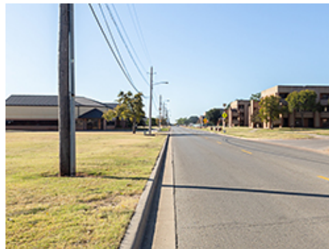
Overhead Power Lines
