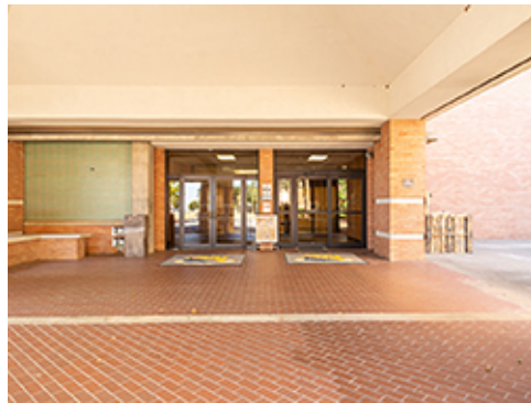
Unit Pavers at Group 1
