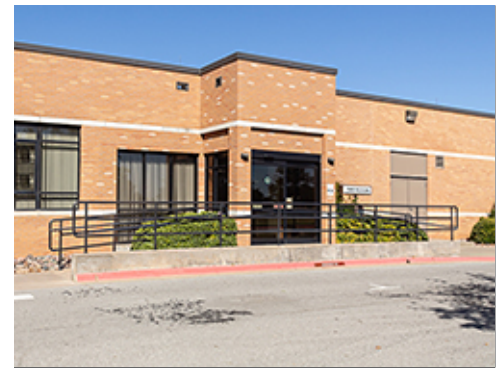
Site Ramp at Building Entrance
