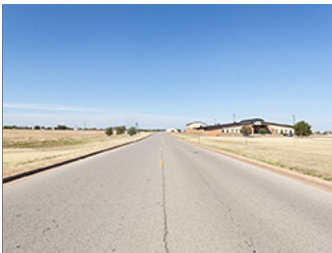
Collector with Center Striping
