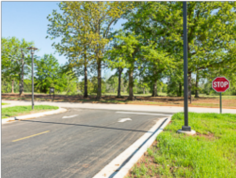
Bituminous Pavement with Concrete Curb
