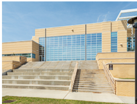
Stairs and Seating Area
