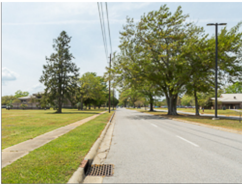
Overhead Power, Lighting & Drainage
