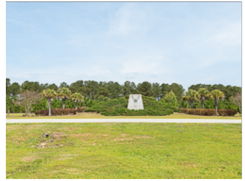
Drainage under Road
