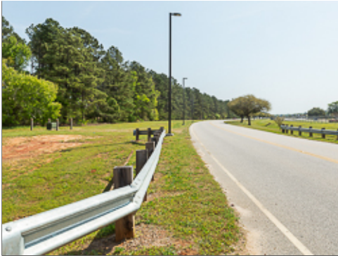
Street Lighting with Underground Power
