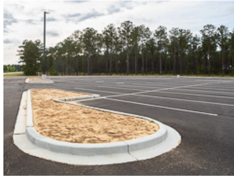
Concrete Island Curb & Gutter
