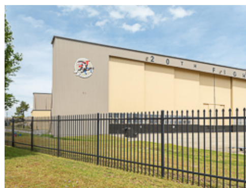
Security Fence at Hangar
