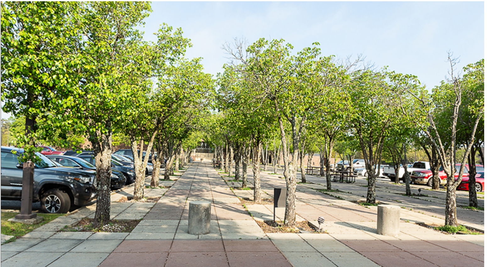
Plaza with Natural and Colored Concrete Paving
