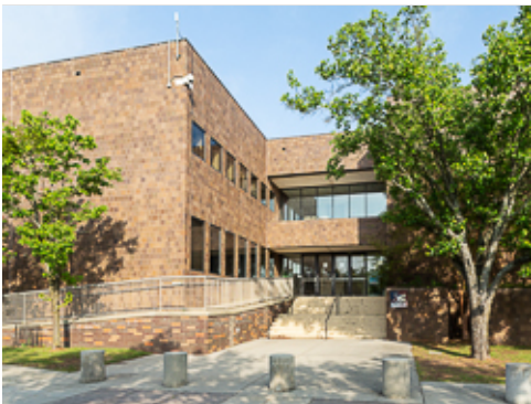
Shaded Plaza in Front of Building
