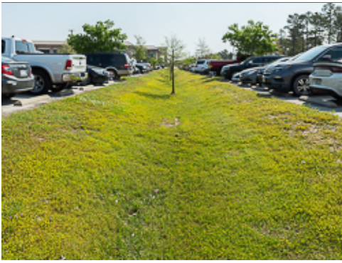
Swale in Parking Lot
