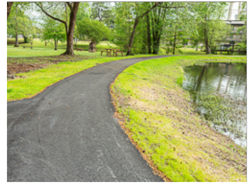
Bituminous Pavement Walk along Pond
