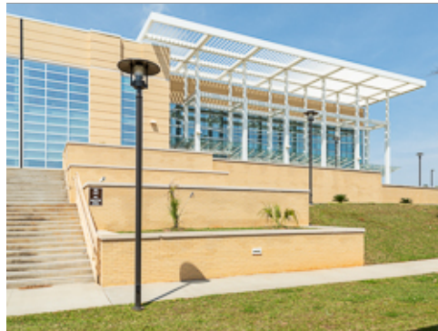
Pole and Wall Lighting
