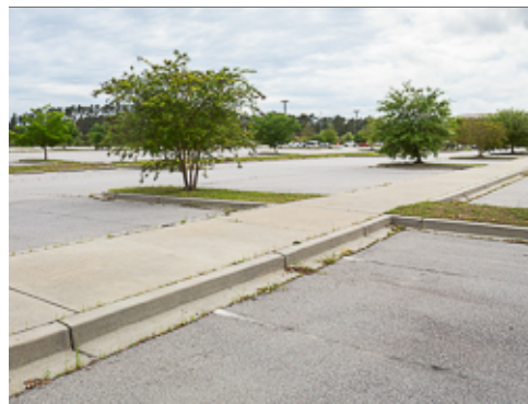
Concrete Curb and Gutter with Walk
