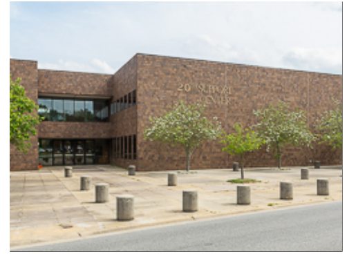
Concrete Bollards at Plaza
