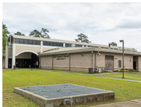
Recessed Utility Equipment
