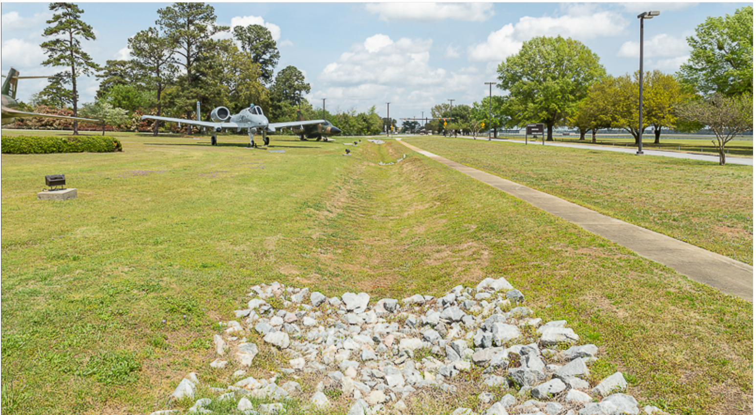
Drainage Channel with RipRap
