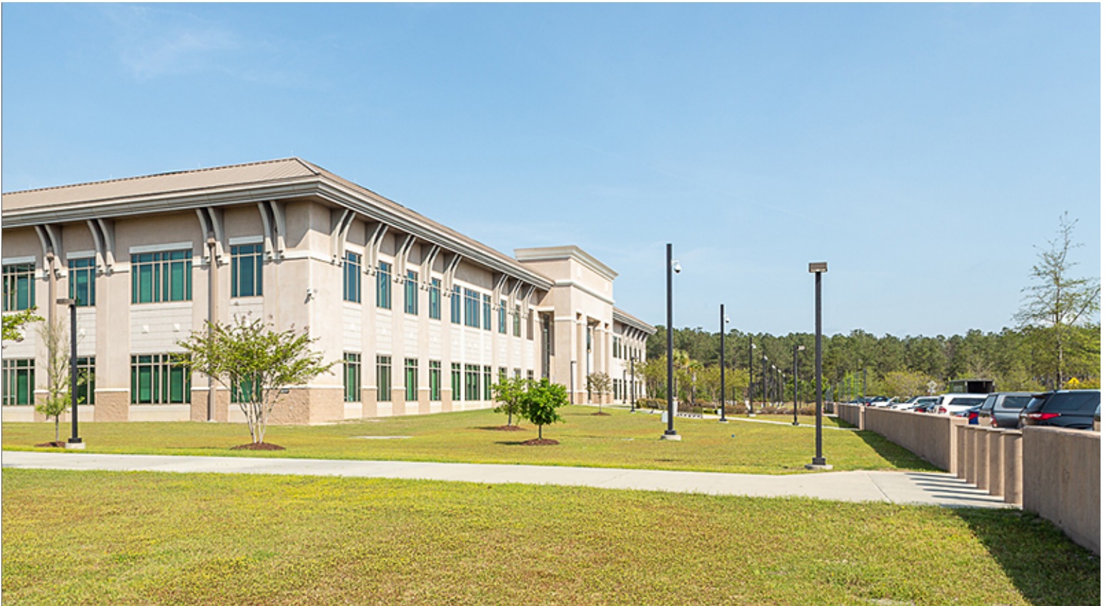
Coordinated Building Placement with Adjacent Parking and Fencing
