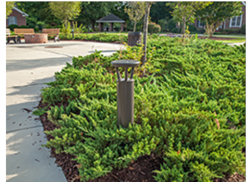
Lighted Bollard on Group 4
