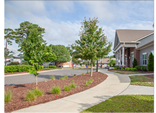
Concrete Sidewalk in Group 4
