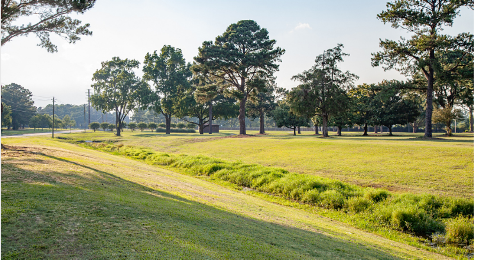
Drainage Basin Maintained as an Amenity
