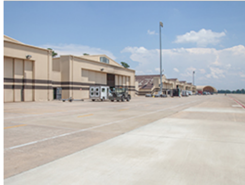
Operationally Required Concrete Paving
