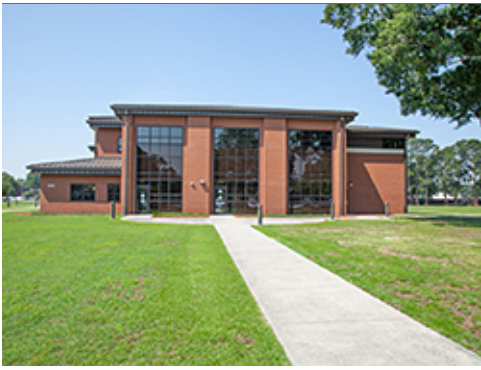
Concrete Paving at Secondary Entrance
