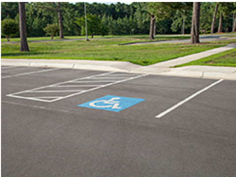
Standard Bituminous Paving, White Striping
