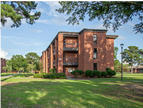
Trees Providing Shade on Buildings
