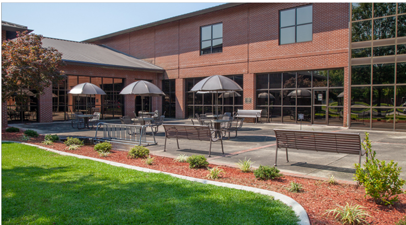
Concrete Paving with Brick Accents at Group 2
