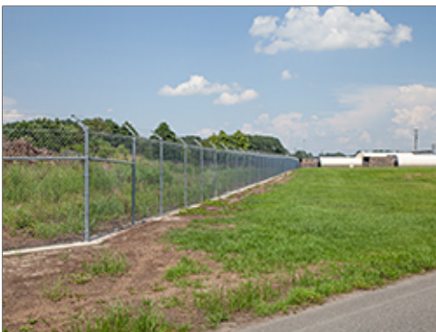
Perimeter Fence near Flightline
