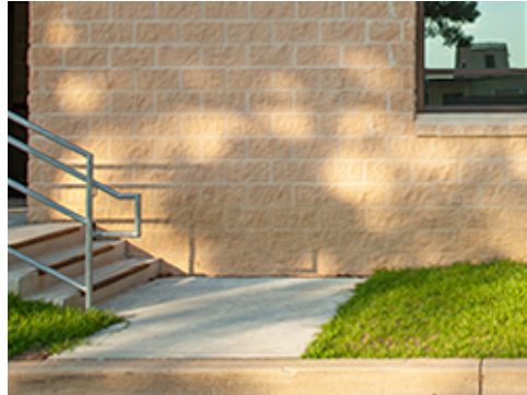
Stair and Landing
