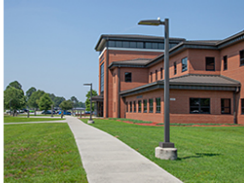
Pedestrian Lighting at Group 1
