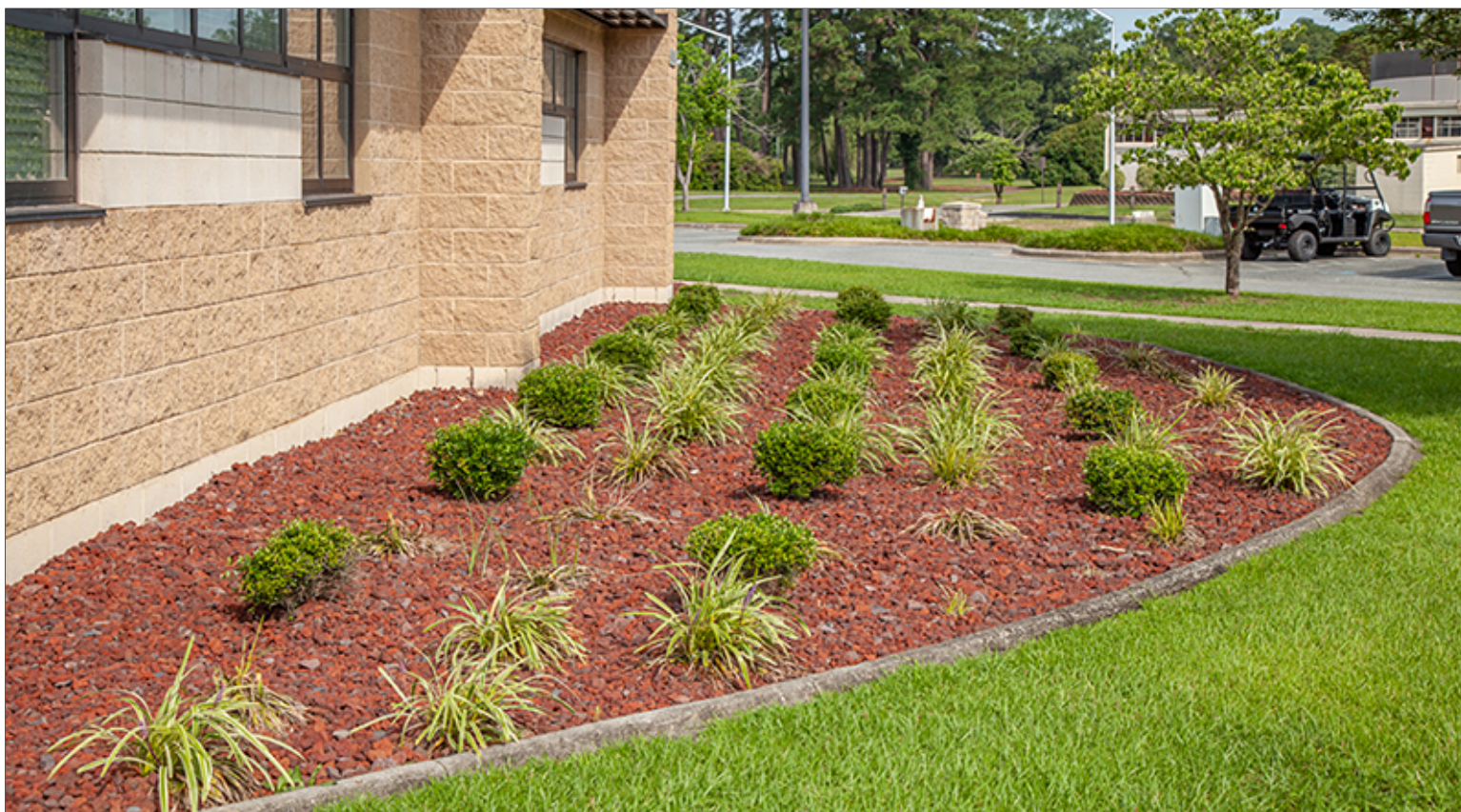
Rock Mulch, Concrete Edging and Xeric Planting in Group 1 near Flightline
