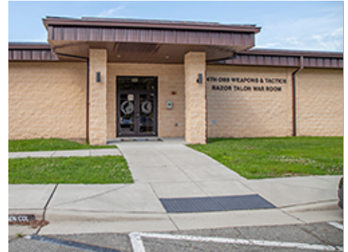
Grade Accommodated with Sidewalk
