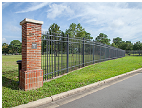
Brick Pier and Metal Fencing
