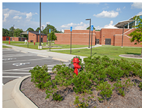
Fire Service Line and Hydrant
