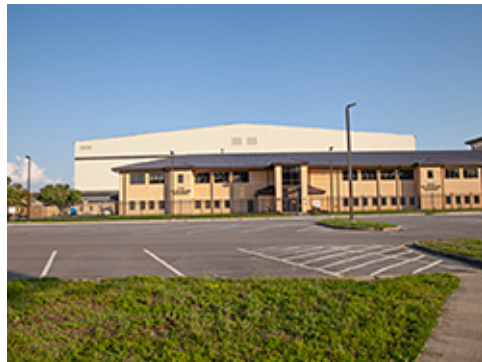
Group 3 Paving and Striping
