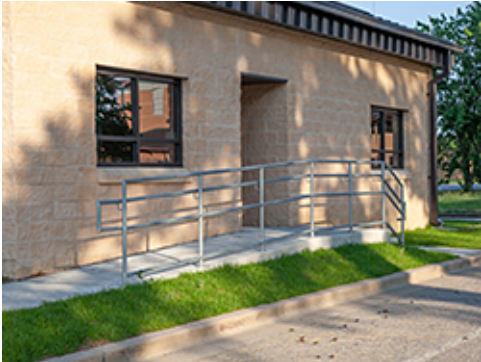
Integrated Ramp and Railing
