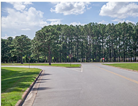
T Intersection with Merge Lane
