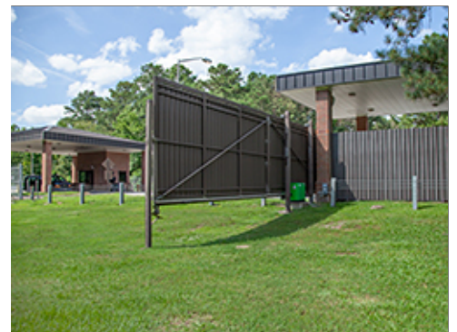
Construction Entrance Facilities
