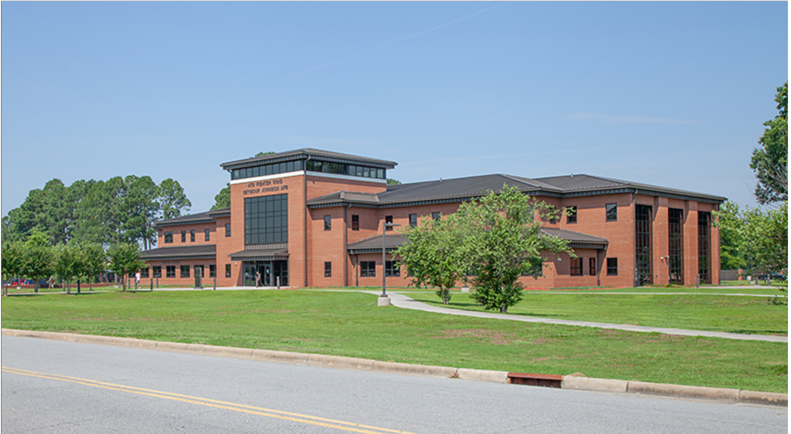
Group 1 Headquarters Facility with Red Brick and Metal Roof
