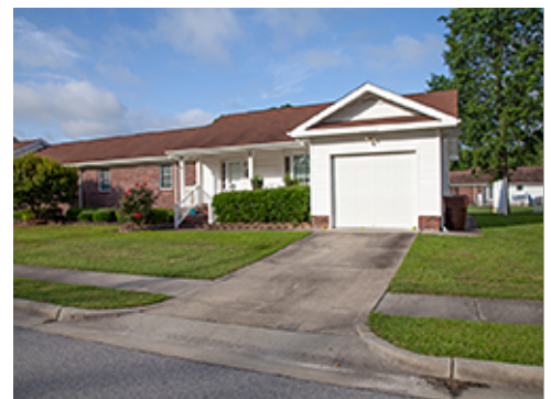
Concrete Driveway at Group 4
