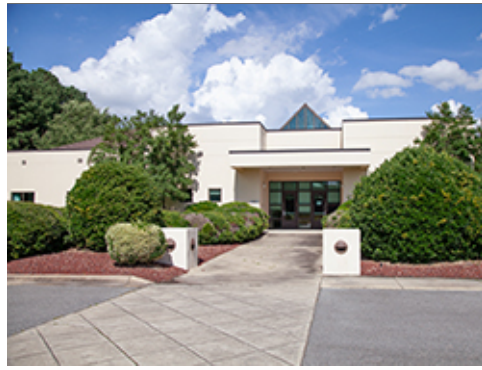
Decorative Control Joints at Group 2
