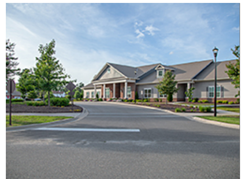
Intersection at Group 4
