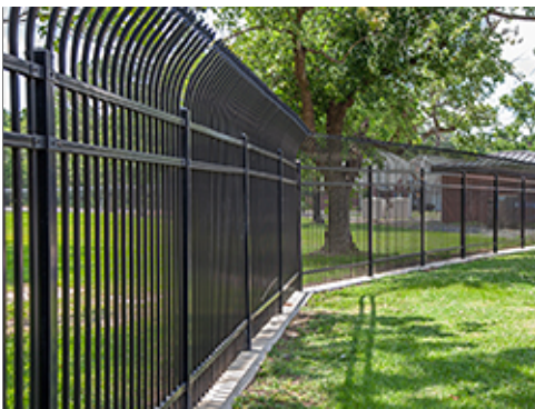
Fencing Detail with Outriggers
