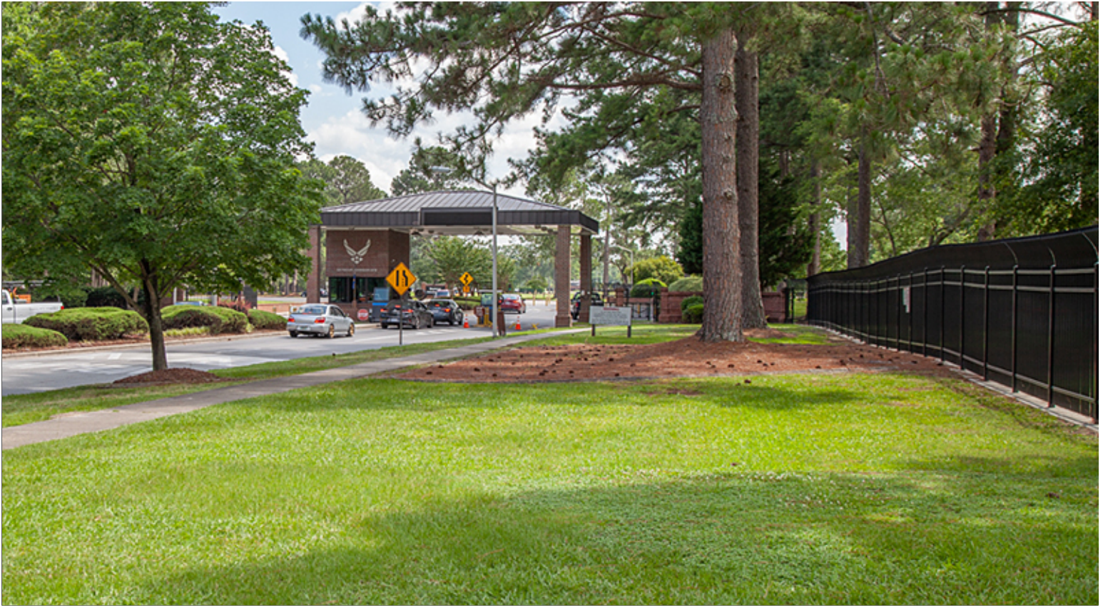
Fencing at Group 1 Berkeley Gate
