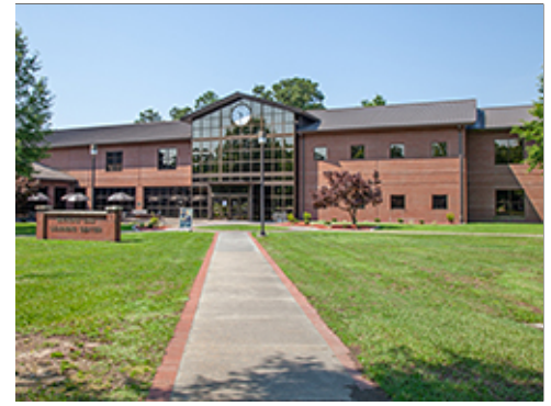
Brick Edging at Group 2
