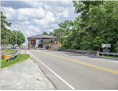
Truck and Commercial Gate
