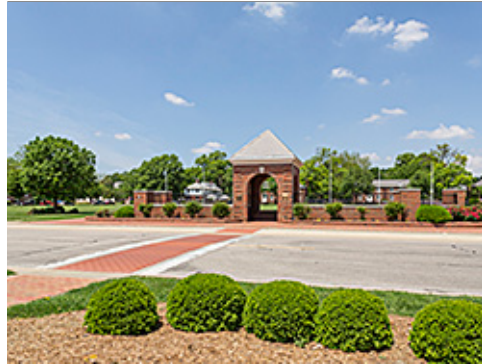
Colored Pavers Crosswalk at Group 1
