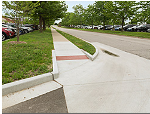
Curb Ramp at Street Crosswalk
