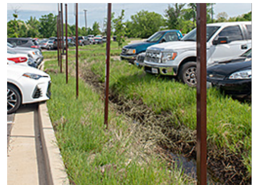
Grasses in Bioswale
