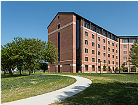
Concrete Paving in Group 2
