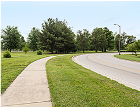
Detatched Sidewalk along Collector Street
