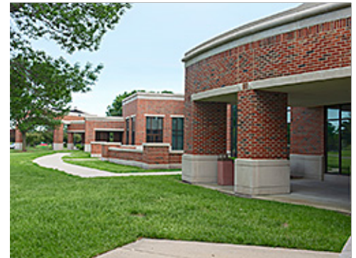
Brick and Architectural Precast
