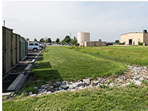
Parking Surface Discharge to Riprap
