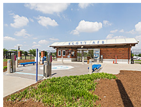
MetroLink Entrance Station
