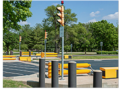
ATRP Control Systems
