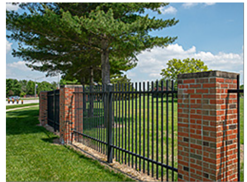
Perimeter Fence Adjacent to Group 1
