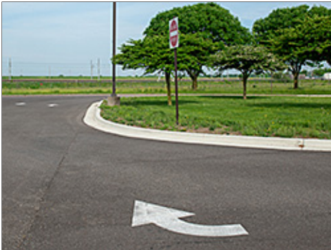
Bitumenous Concrete Paving
