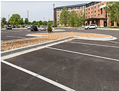
Integral Curb and Gutter
