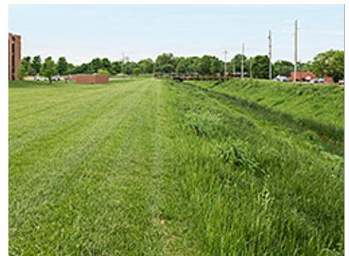
Integrated Stormwater Greenway
