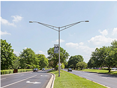
Double Pole Street Lighting
