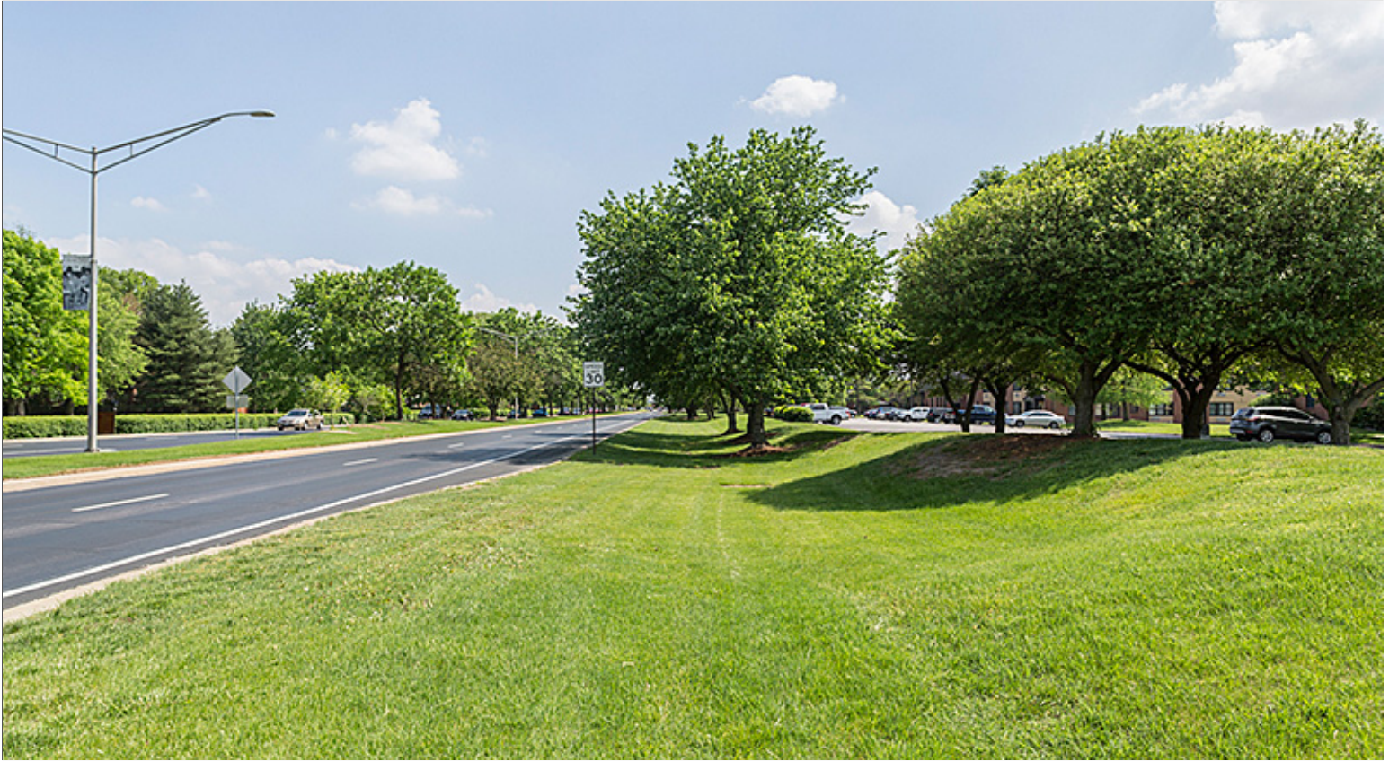
Gentle Grades in Topography and Grassy Basins with Pervious Subgrade Materials
