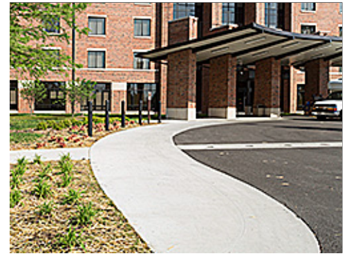
Zero Curb at Entrance
