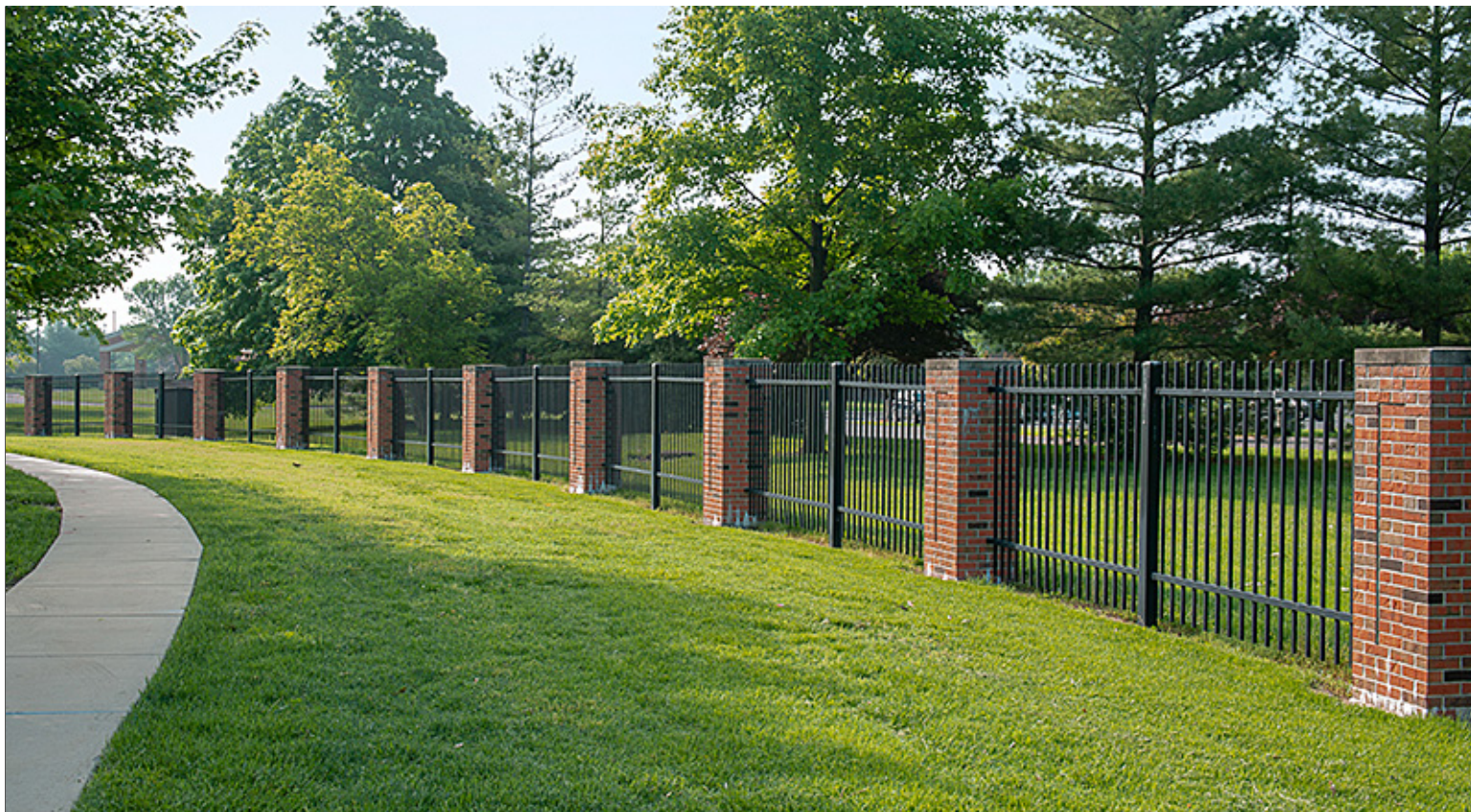
Perimeter Fence Adjacent to Facility Group 1 Entry Control Facility (ECF)
