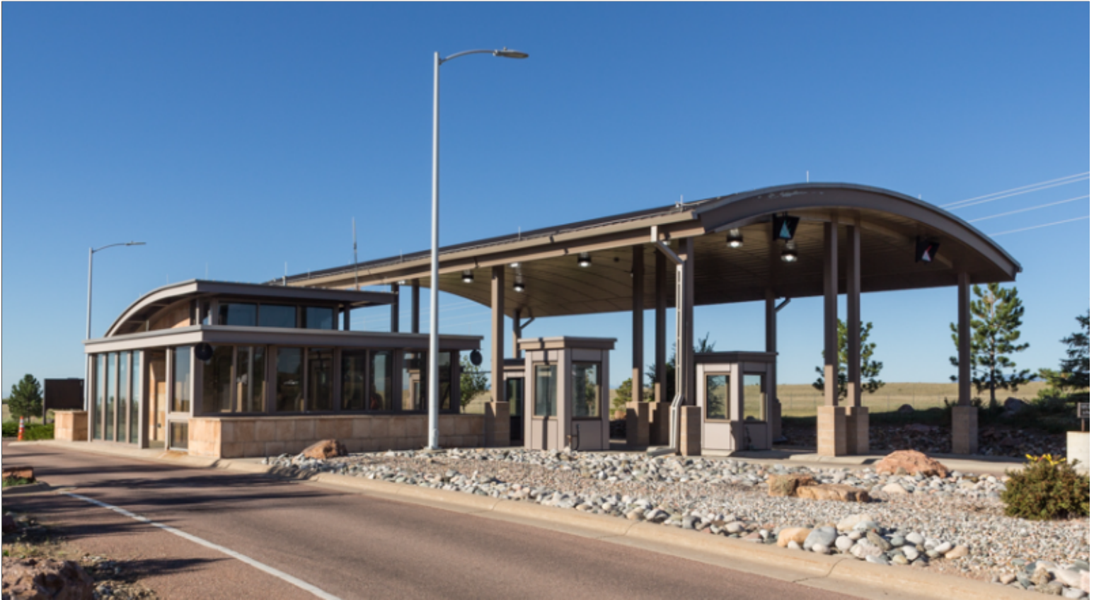
North Entry Control Facility
