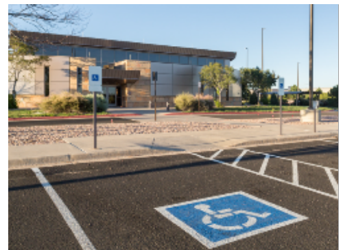
Adjacent Accessible Parking
