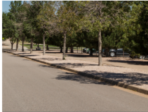
Curb and Gutter
