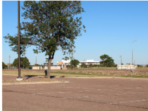
Paving and Striping
