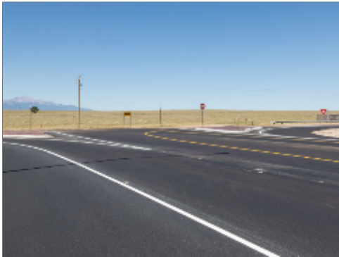
Falcon Parkway Asphalt Paving
