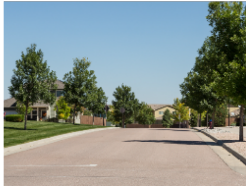
TVC Privatized Housing Asphalt Paving
