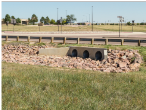
Culvert with Wingwalls and Slope Protection
