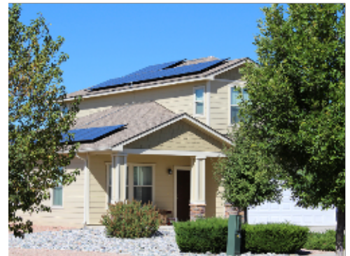
Screening at Exposed Utilities
