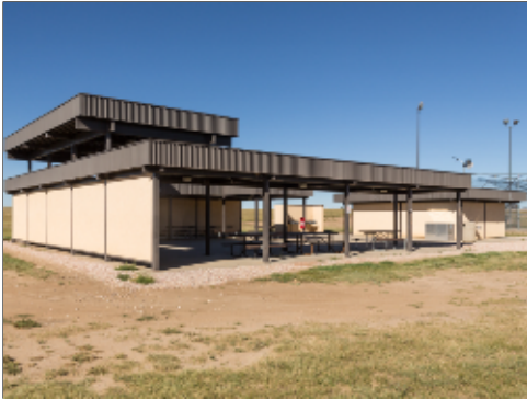
Community Area Pavilion
