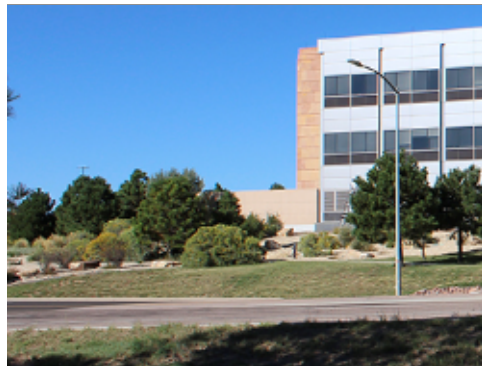
Screening at Utility Enclosure
