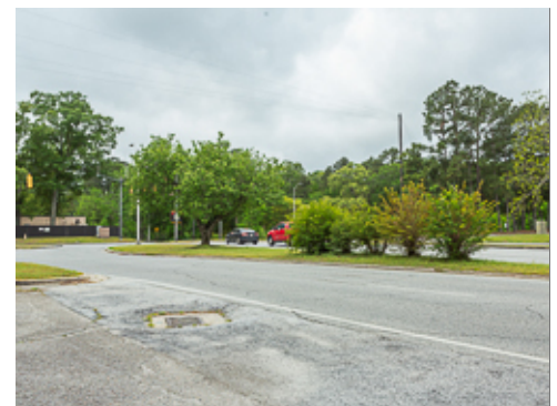
Local Street Intersection
