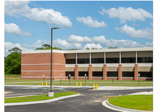
Pole Light at Parking Island
