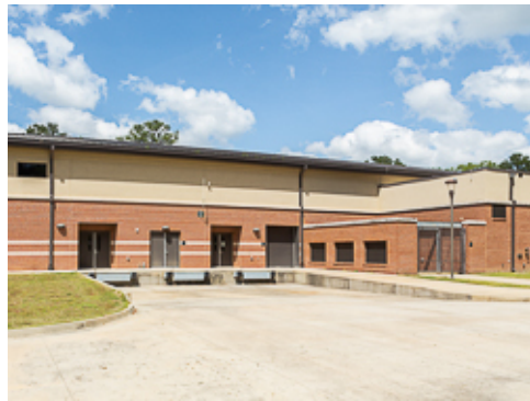
Ramp to Loading Dock
