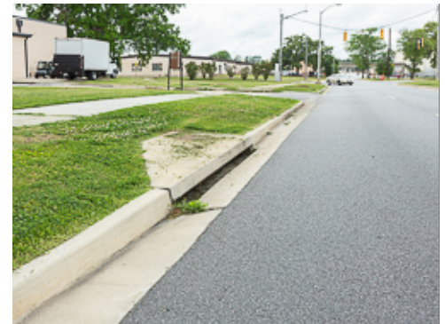
Cohesive Storm Drainage Elements
