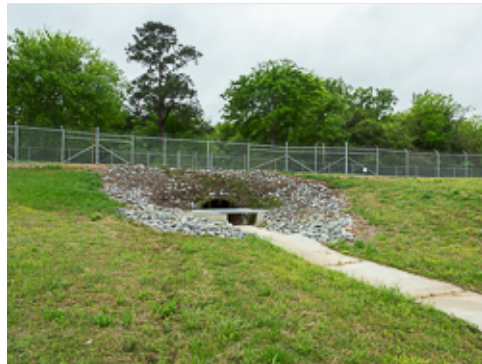
Drainage Under Road / Fence
