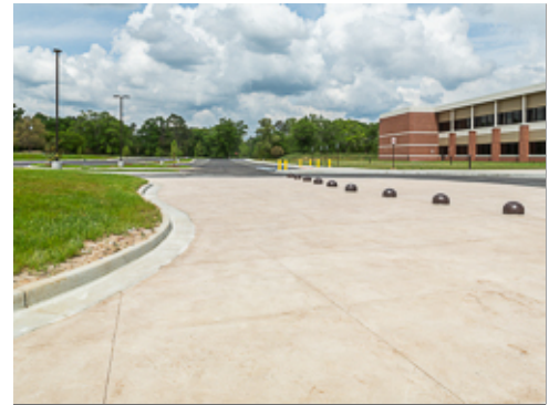
Special Paving at Group 1
