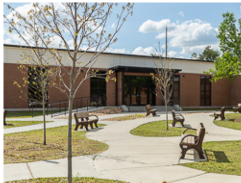
Ramp to Entry
