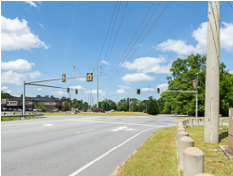
Vehicle Barriers at Utility Components
