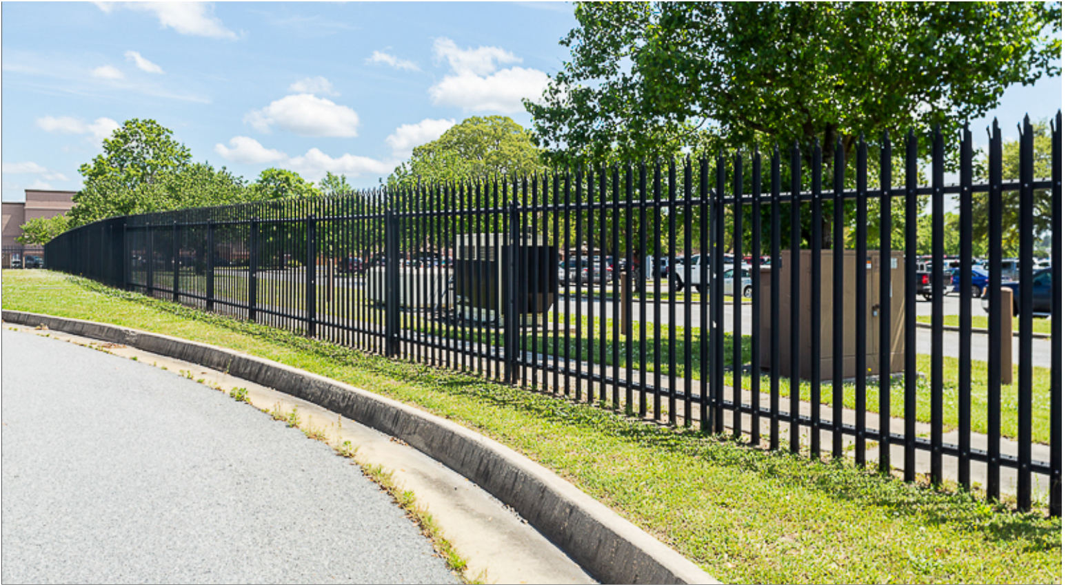
Perimeter Fence near Entry
