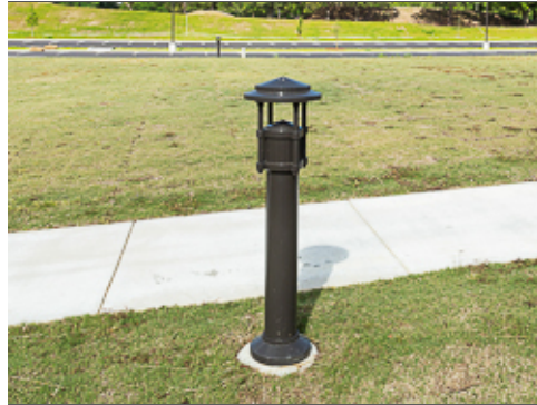
Bollard Light on Sidewalk
