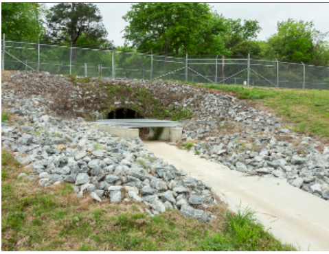
Drainage Channel under Fence
