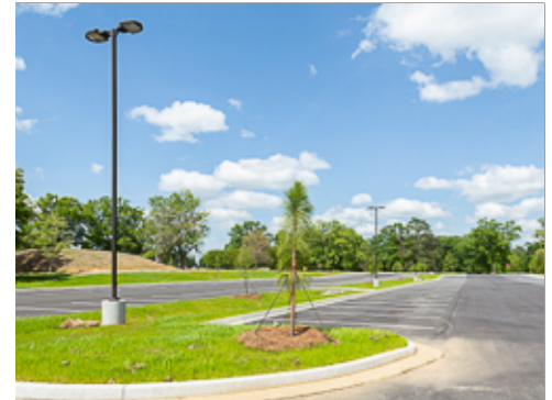
Light Pole Protected from Traffic
