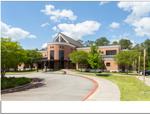
Sidewalk along Street
