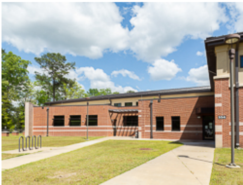
Sloped Sidewalk to Building
