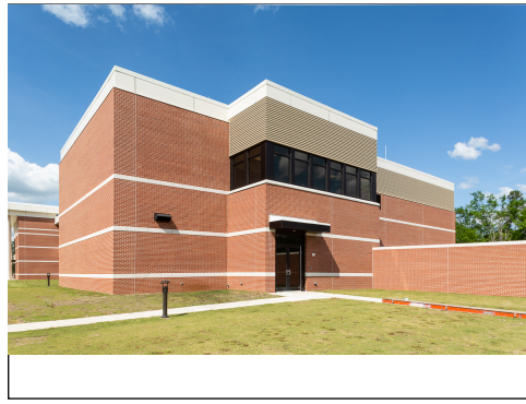
Lighting on Pedestrian Path
