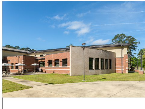
Concrete Paving, Tables on Plaza
