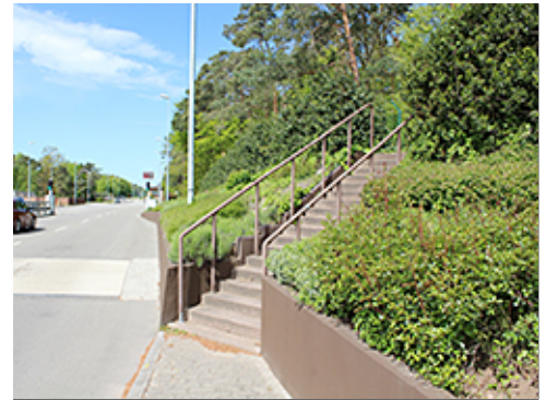
Stair and Retaining Wall
