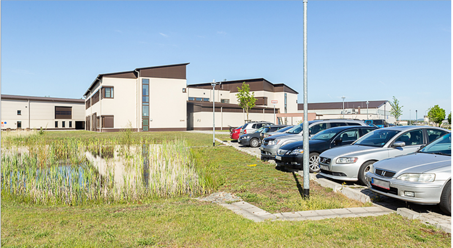
Stormwater Drainage Directed from Parking Lot to Retention Area
