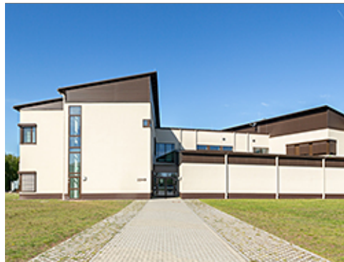
Unit Pavers at Entrance
