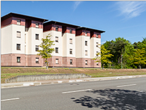
Building Setback at Group 2
