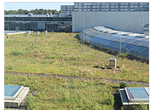
Vegetated Roof retaining Stormwater
