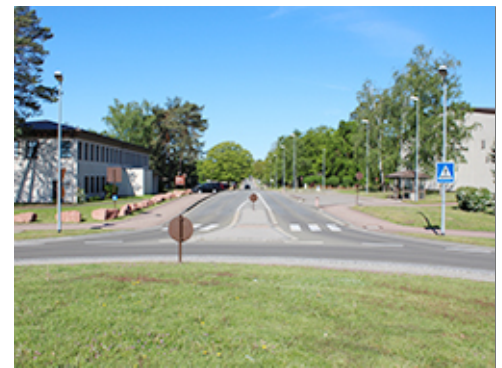
Divided Median at Roundabout
