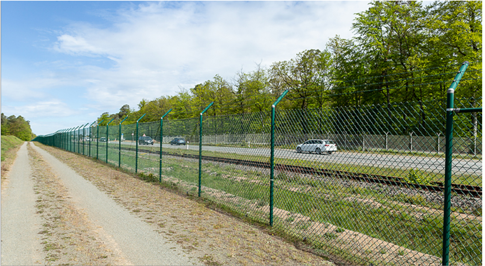
Base-wide Standard Perimeter Fencing
