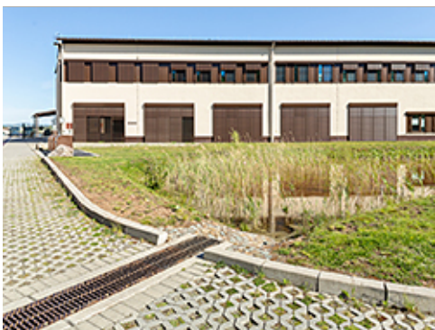
Street Drainage Directed to Retention Area
