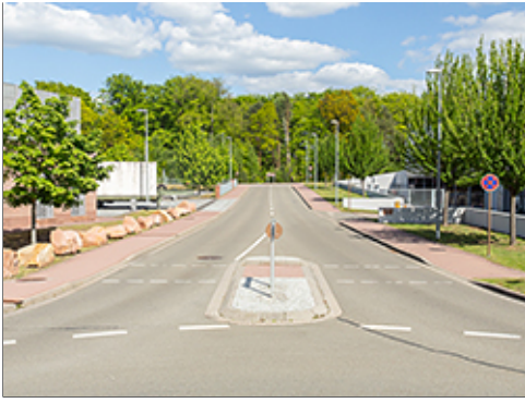
Divided Lanes Near Roundabout
