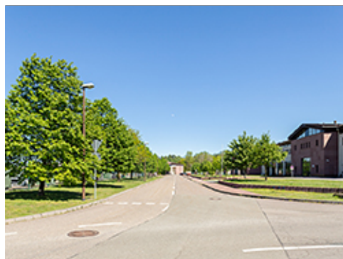
Two-way Traffic with Center Striping
