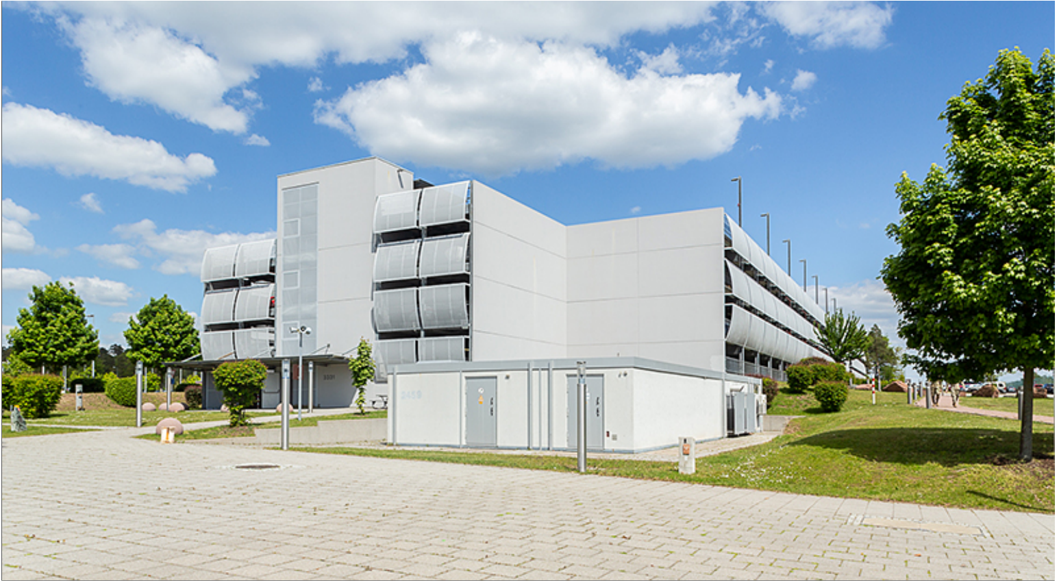
Garage with Wall System of Precast Panels and Perforated Metal Shading Panels
