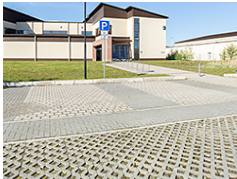
Unit Pavers and Grass Pavers at Aisle
