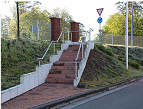
Stair as Retaining Wall
