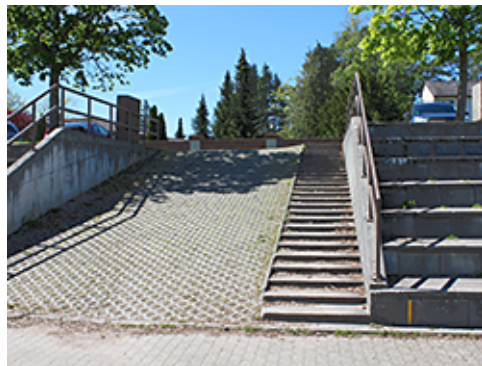
Stair at Access Drive
