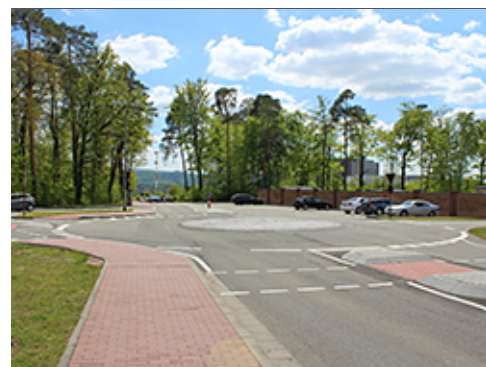
Decorative Paving Near Group 1
