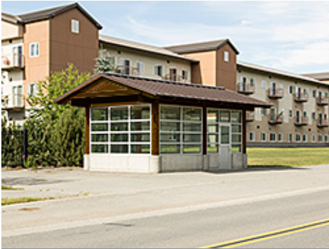
Fully Enclosed Bus Shelter
