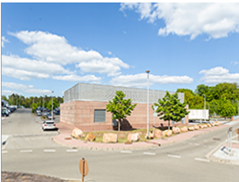
Roundabout at Group 1
