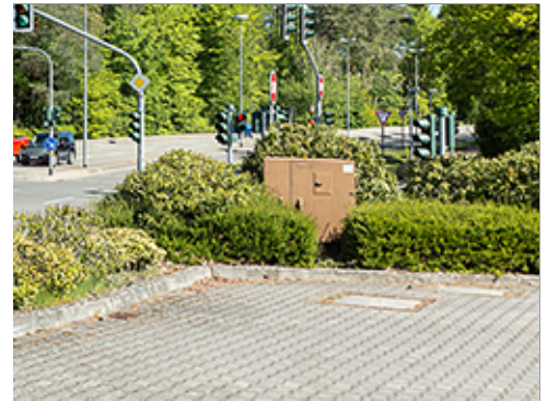
Screening at Utility Cabinet
