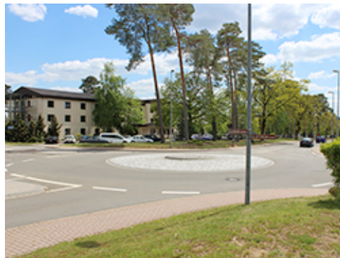
Roundabout at Group 2
