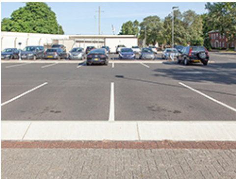
Standard Bituminous Paving, White Striping
