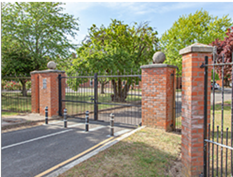
Masonry Piers at Group 1
