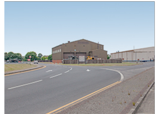
Striping to Denote Principal Route
