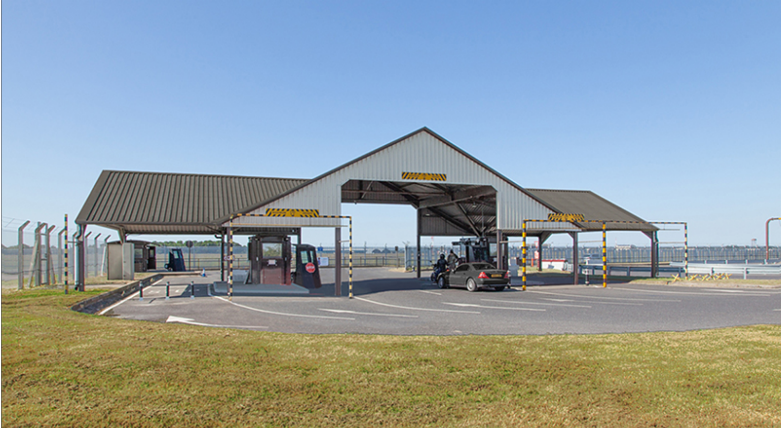
Main Gate at A1101
