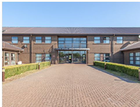
Interlocking Pavers at Group 1
