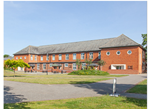
Adaptive Use of a Historical Building
