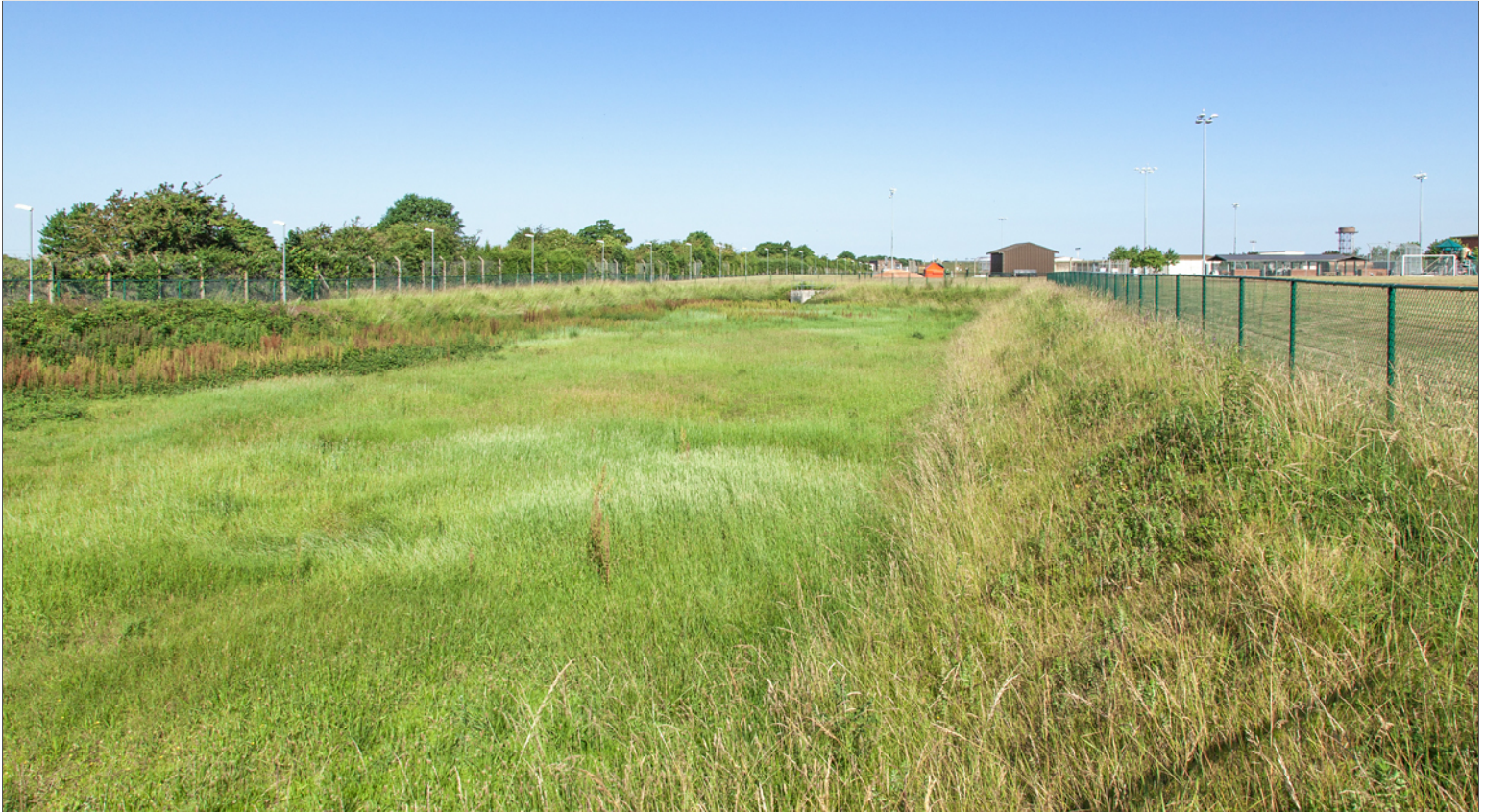
Stormwater Retention Basin with Integrated Fencing and Vegetation
