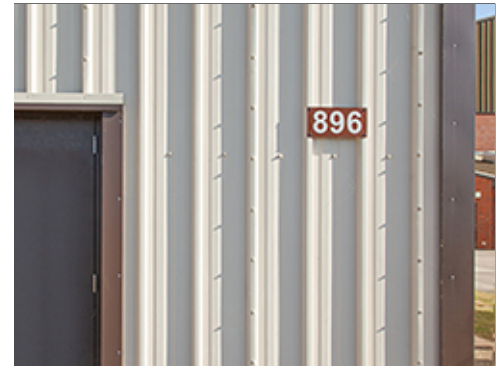
Standard Building Number at Group 3
