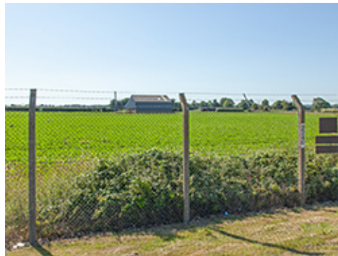
Concrete Posts with Outriggers
