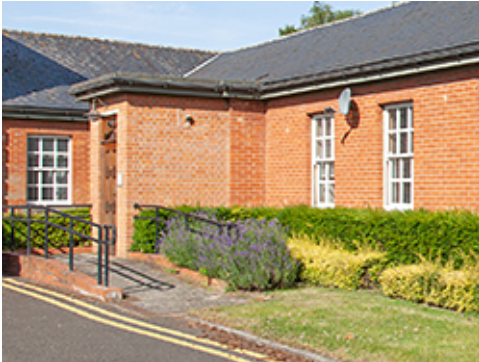
Site Ramp at Entrance
