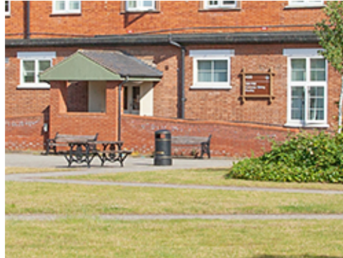
Sloped Wall along Ramp
