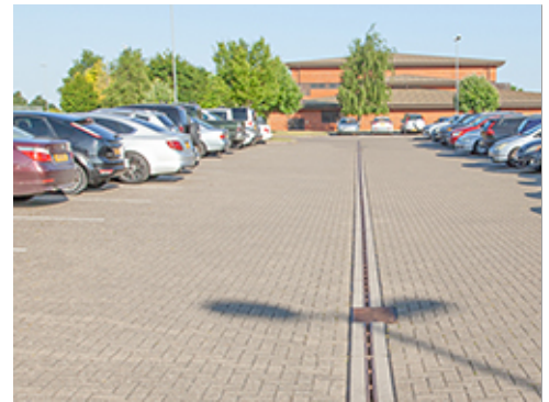
Paving Sloped to Trench Drain
