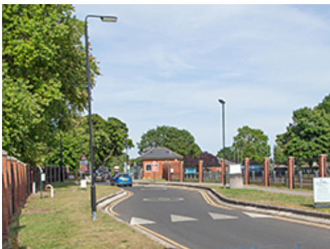
Light Fixtures at Controlled Access Area
