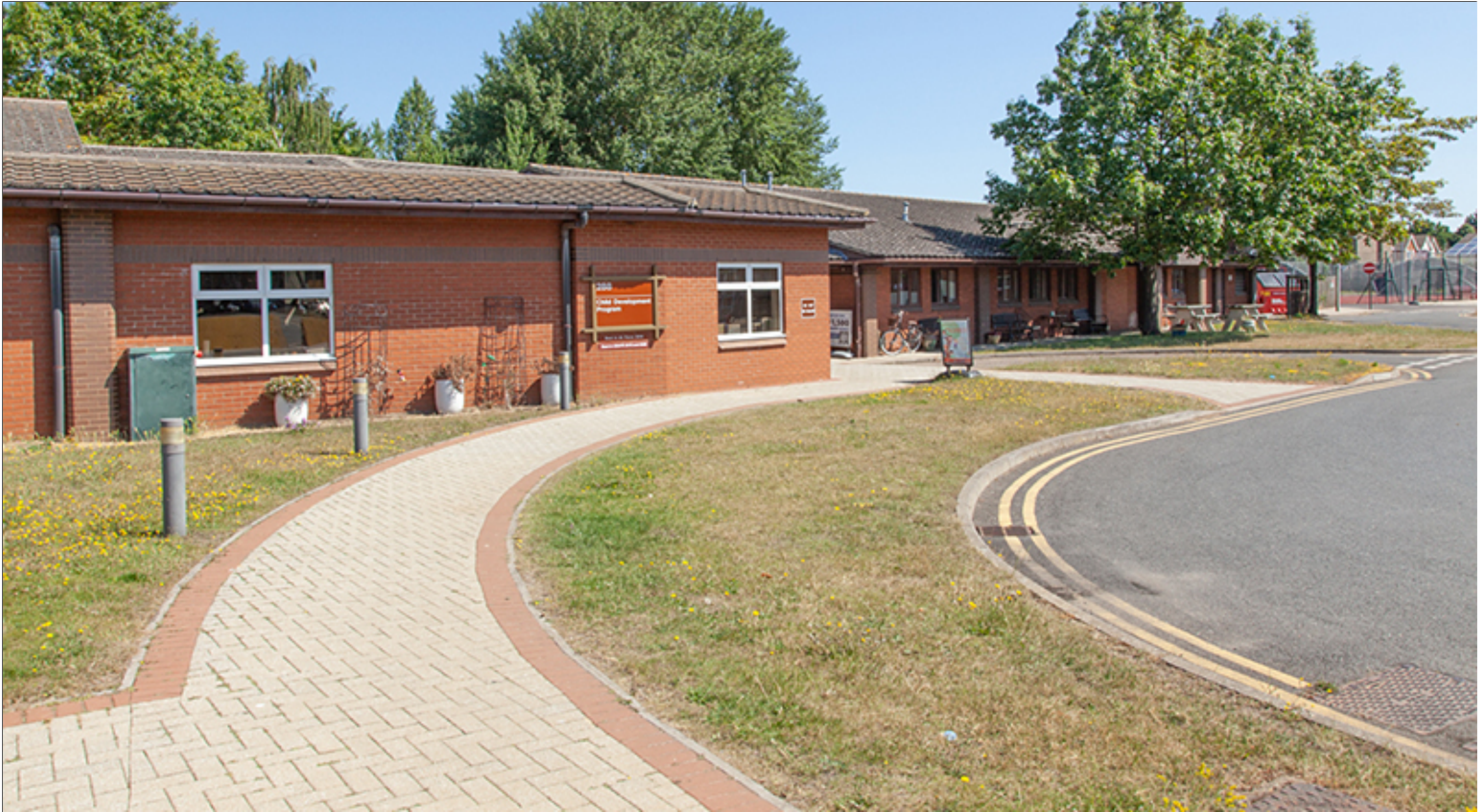
Permeable Pavers with Interlocking Pattern and Contrasting Color for Edging
