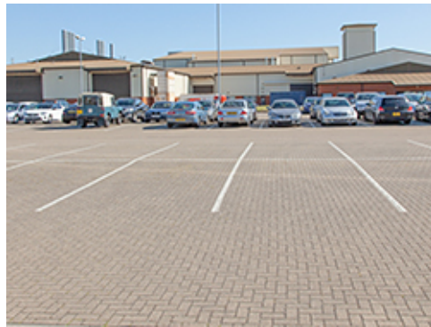
Painting Striping on Unit Pavers
