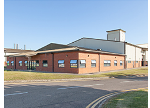
Site Sloped to Accommodate Grade
