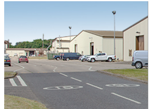
Street Adjacent to Group 3 Facilities
