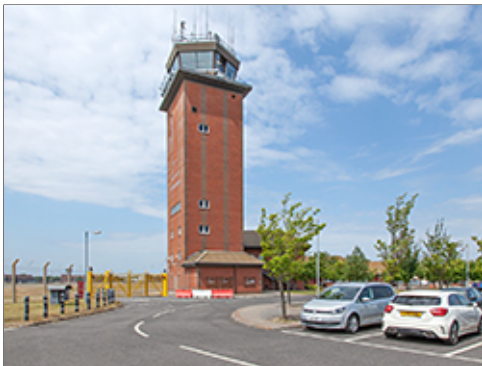
Local Street near Group 2
