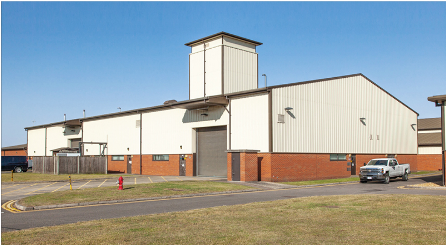
Architectural Features, Materials and Detailing Expressive of the Industrial Use
