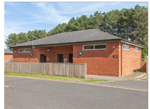
Toilet Rooms at Park
