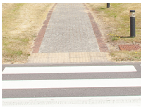
Curb Ramp at Crosswalk
