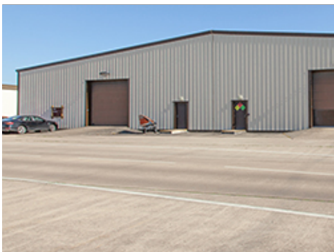
Functionally Required Concrete Paving
