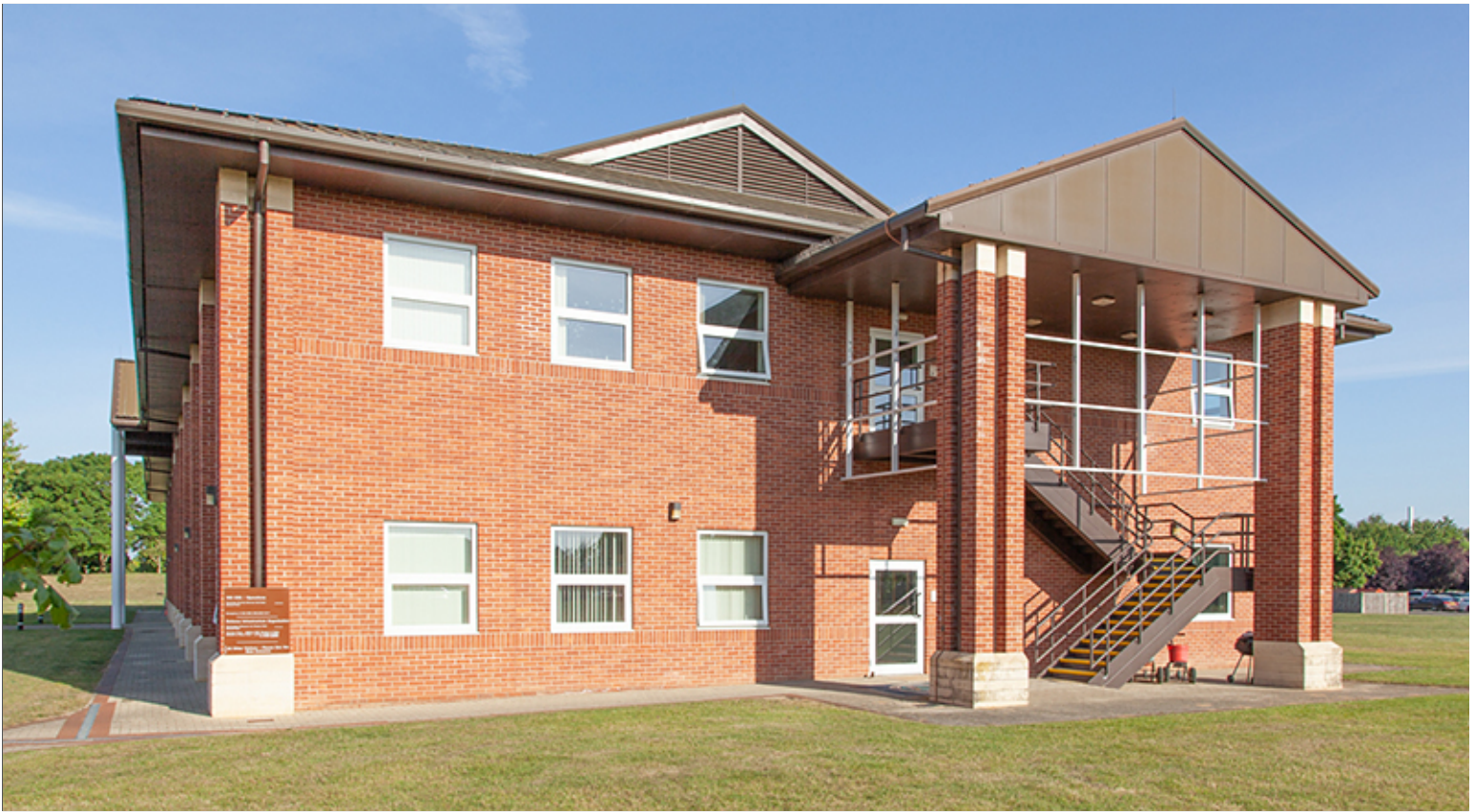
Predominant Use of Red Brick with Architectural Precast Accents Metal Panels at Gabled End Wall and Metal Soffits
