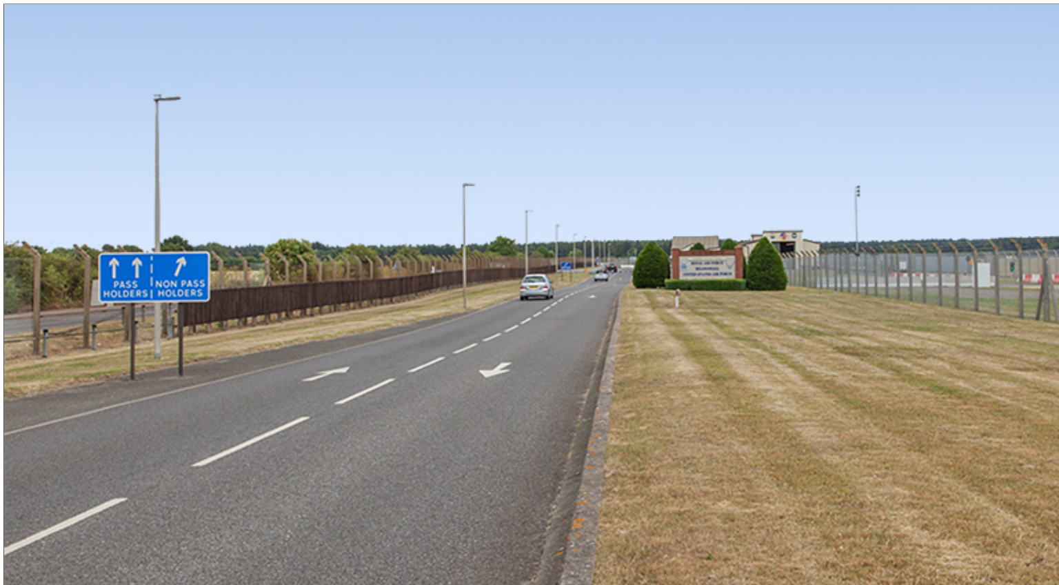
Directional Signs and Approved Monument Sign at Main Gate
