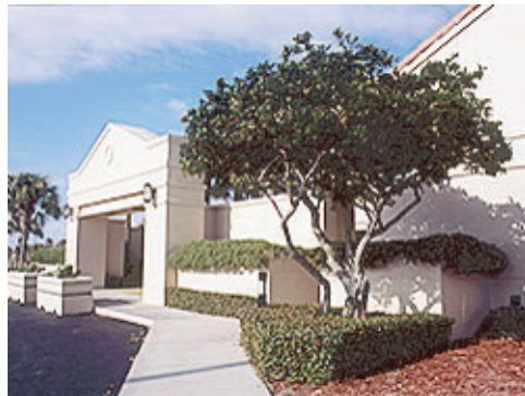
Attached Sidewalk at Parking Area
