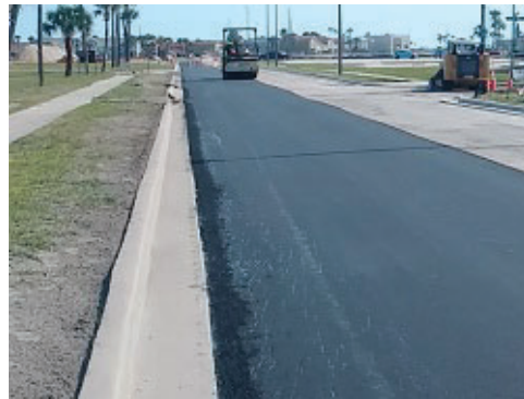
Compaction Process
