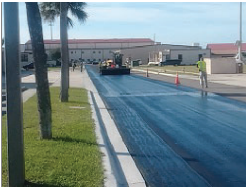
Placement of Compliant Materials
