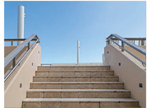
Stair with Highly Durable Finishes
