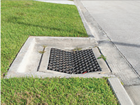
Underground Utility Services
