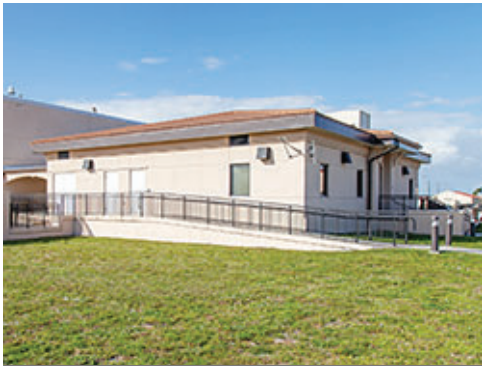
Ramp Integrated with Building
