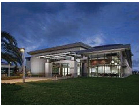
Coordinated Path and Entrance Lighting
