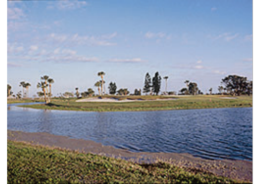
South Base Regional Stormwater Canal
