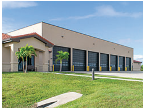
Group 3 Apparatus Bays at Fire Station
