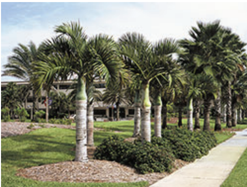
Detached Sidewalk at Street
