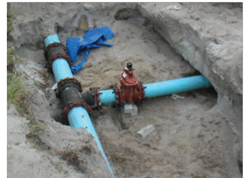
Underground Utility Services
