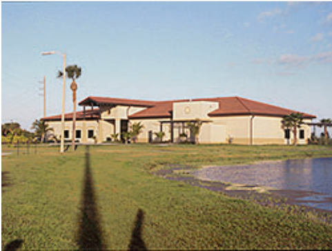
Generally Flat Site
