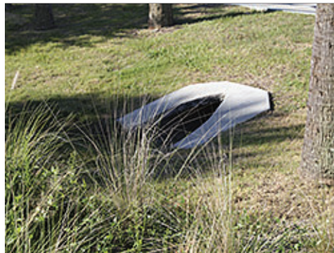
Underground Utility Services
