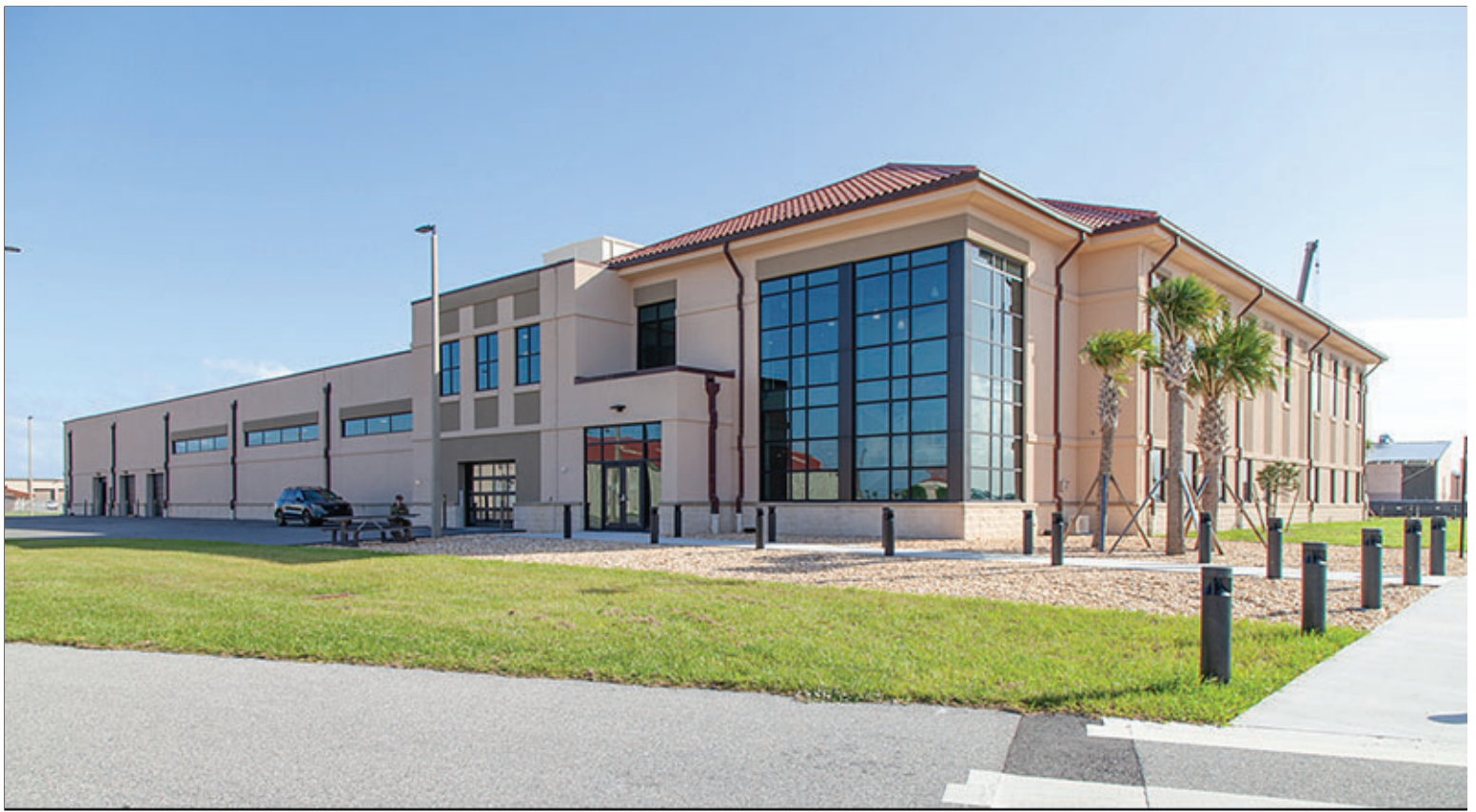
Curtain Wall Glazing Feature Used to Define Entrance
