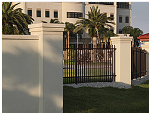
Perimeter Fence Detail
