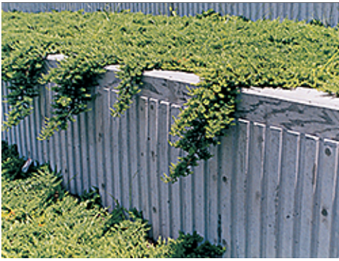
Screened Retaining Walls
