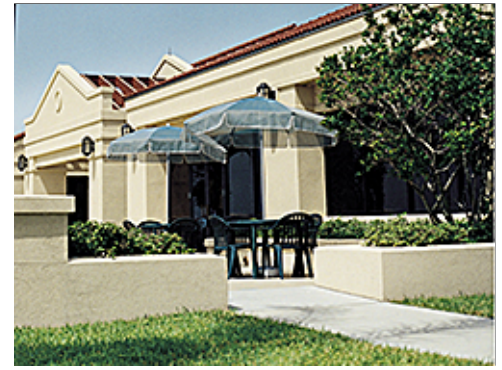
Screen Walls and Planters
