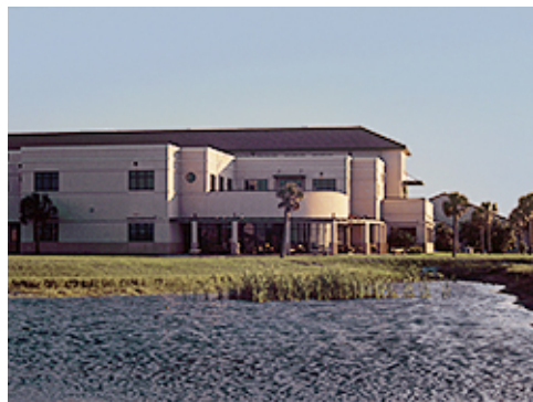
Retention Pond in Open Space
