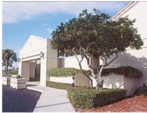
Attached Sidewalk at Parking Area
