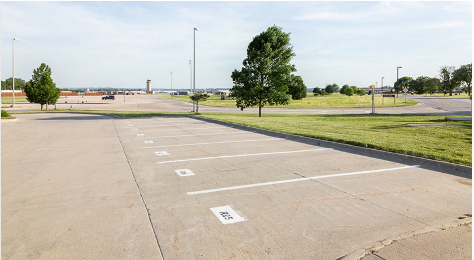
Concrete Paving with Standard White Striping
