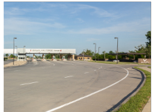
Approach Route to Stratcom Gate
