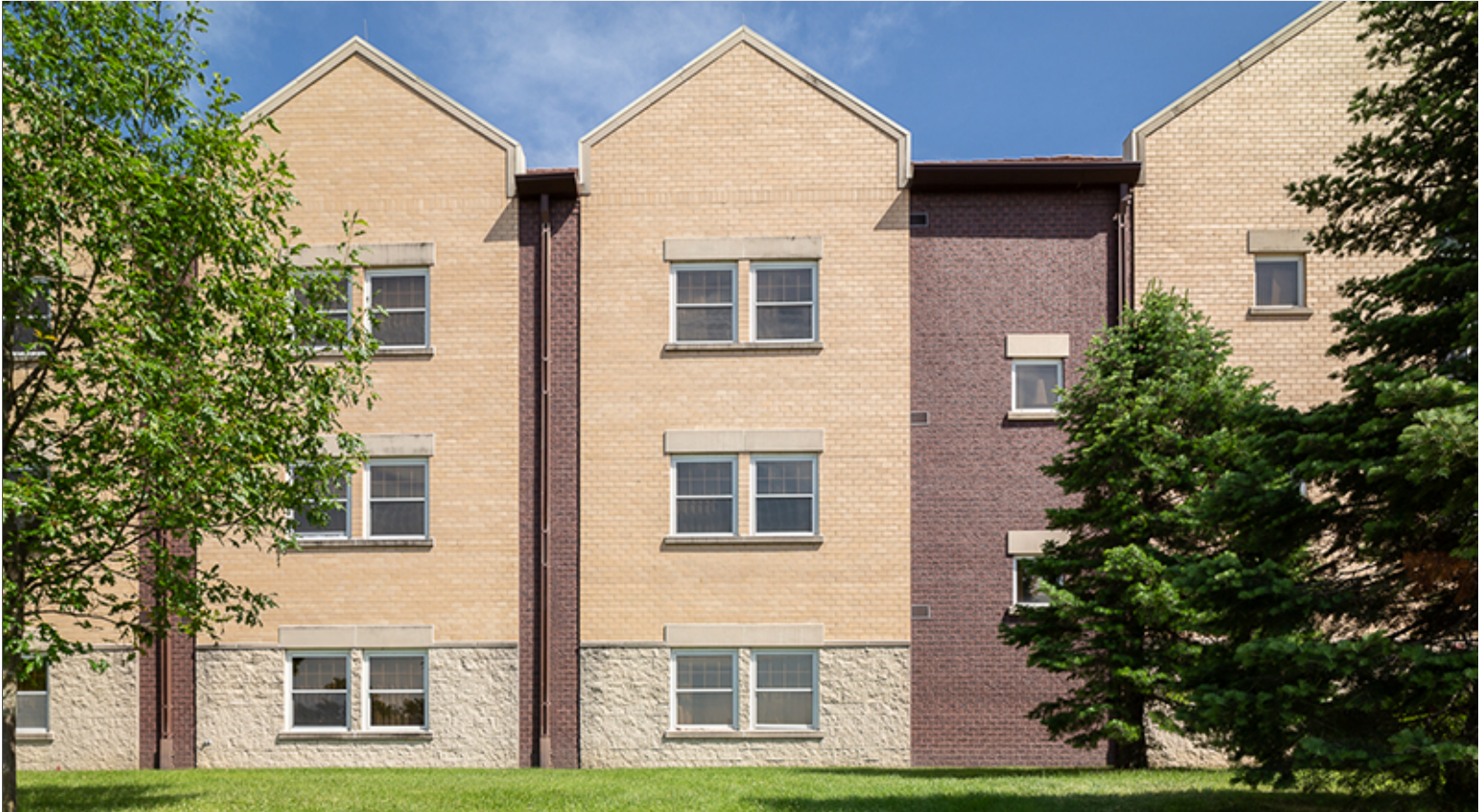
Roof Drain Downspouts Connected to Storm Sewer System
