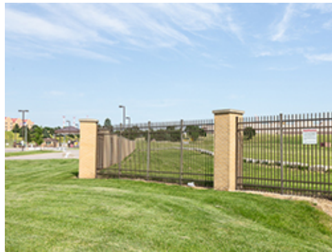
Post and Rail Fencing at Group 1
