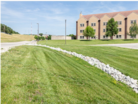
Rock Rip Rap in Drainage Swale
