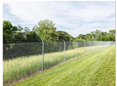
Galvanized Chain Link at Group 3
