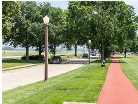
Historical Area Light Fixtures
