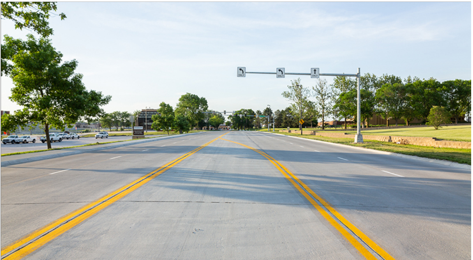
Concrete Paving with Standards Striping
