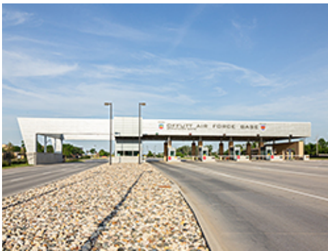
SAC Gate on Butler Boulevard
