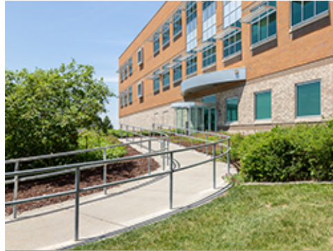
Ramp with Railings
