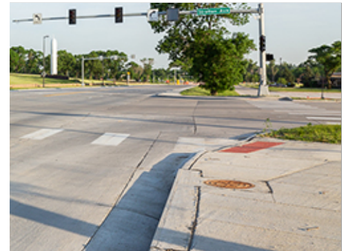
Stormwater Inlet at Curb and Gutter
