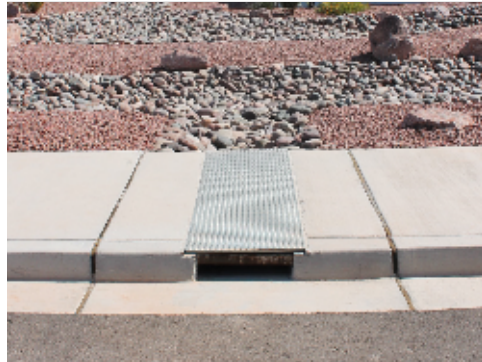
Curb Outlet and Swale
