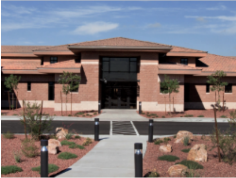
Alignment with Main Entrance
