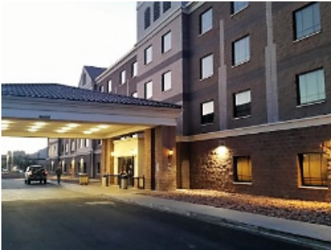
Lighting at Main Entrance
