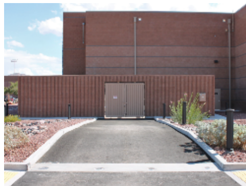
Mechanical Yard Enclosure and Access Drive
