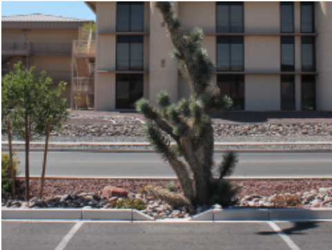
Curb Cut and Swale
