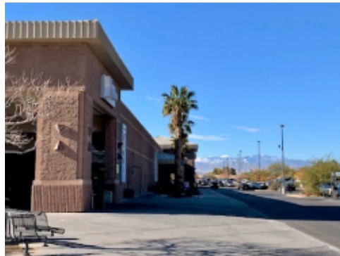
Concrete Paving at Plaza
