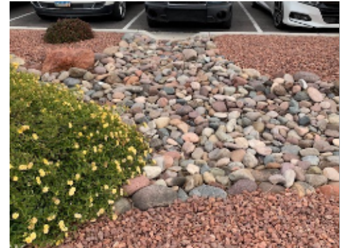
Curb Cut and Swale
