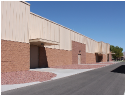
GOV Access Drive
