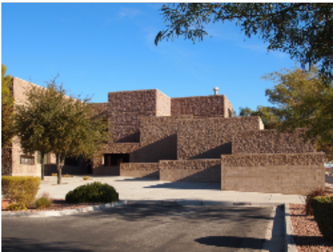
Concrete Paving at Facility
