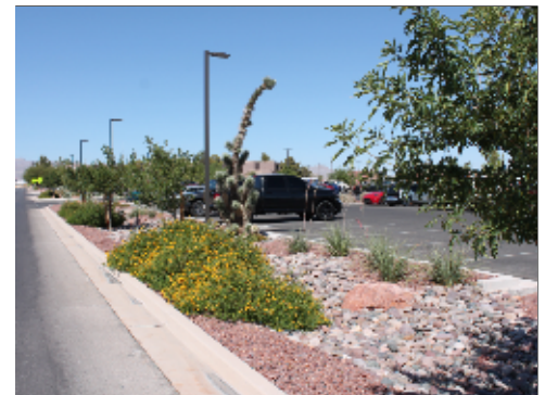
Street Curb and Gutter
