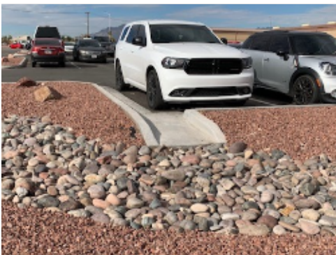
Curb Cut and Swale
