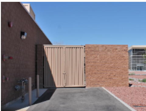
Mechanical Yard Enclosure and Access Drive
