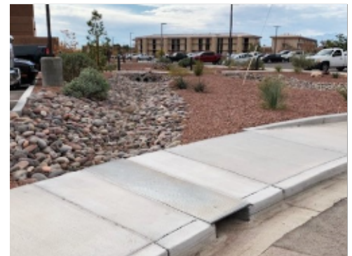
Curb Outlet and Swale
