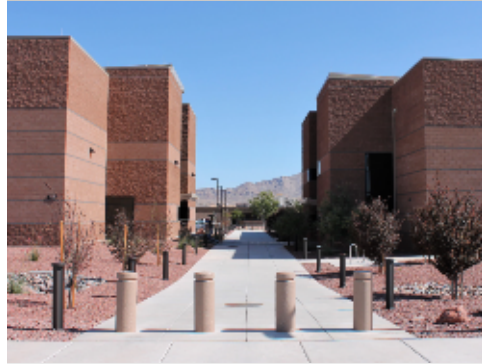
Bollards for Controlled Access
