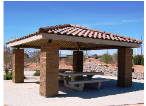
Concrete Paving at Pavilion
