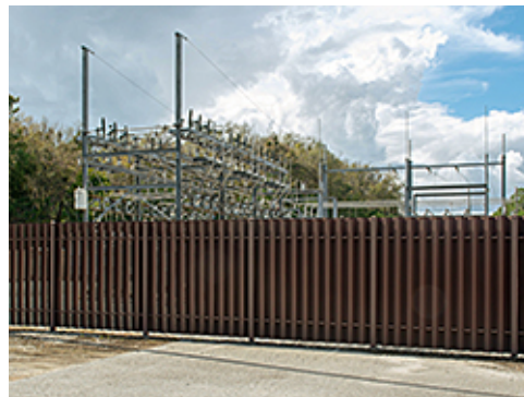
Screening at Utility Structure
