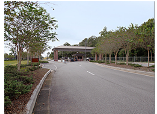
Group 1 Facility and Elements
