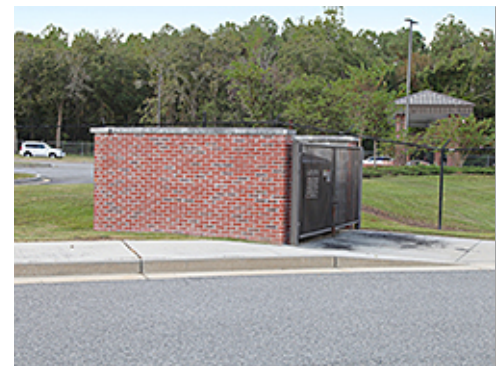
Dumpster Enclosure at Group 1
