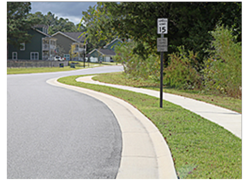
Detached Sidewalk in Group 4
