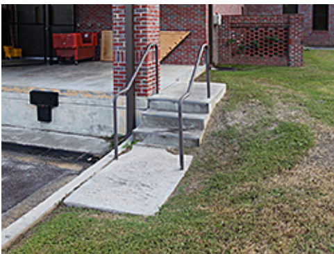
Site Stair at Loading Dock
