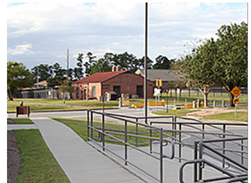
T Intersection at Group 2 Facility
