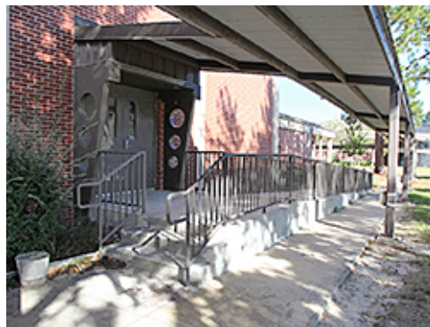
Ramp and Stair at Secondary Entrance
