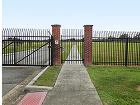
Accessible Sidewalks at Pedestrian Gate
