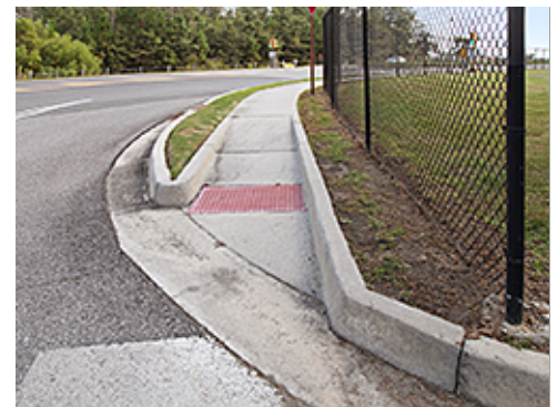
Ramp at Street Intersection
