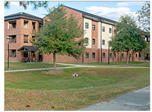
On-Site Detention Area
