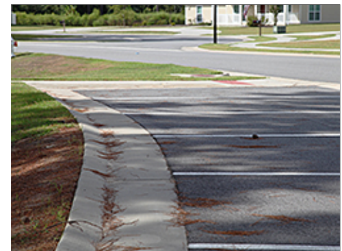
Mountable Curb in Group 4
