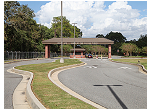
Gate at Davidson Road
