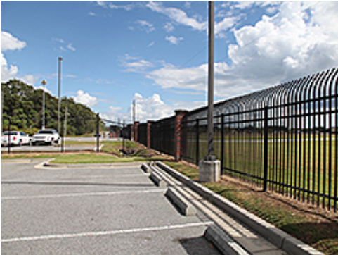
Base Standard Paving and Striping
