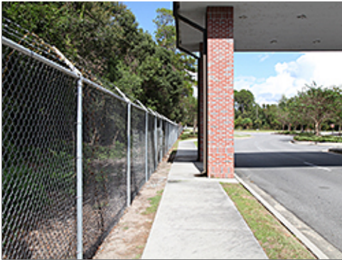
Chain Link Fencing
