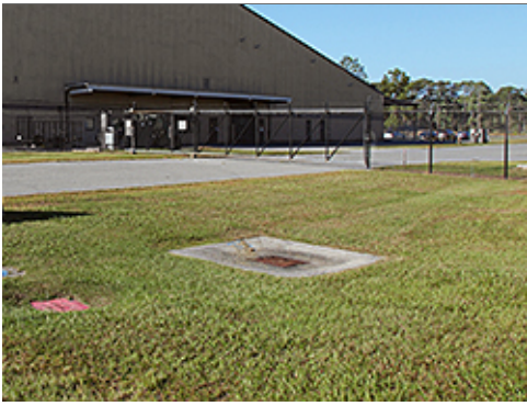
Drainage Inlet in Group 3
