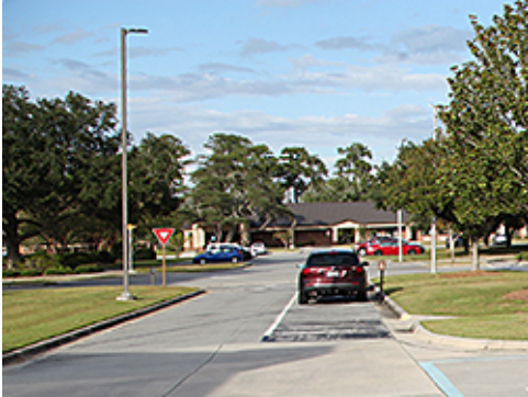
Standard Street Lighting
