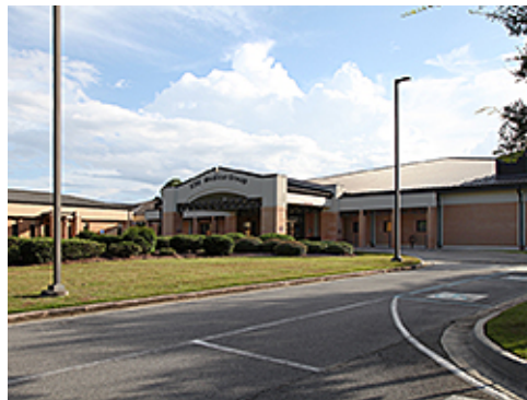
T Intersection at Group 1 Facility
