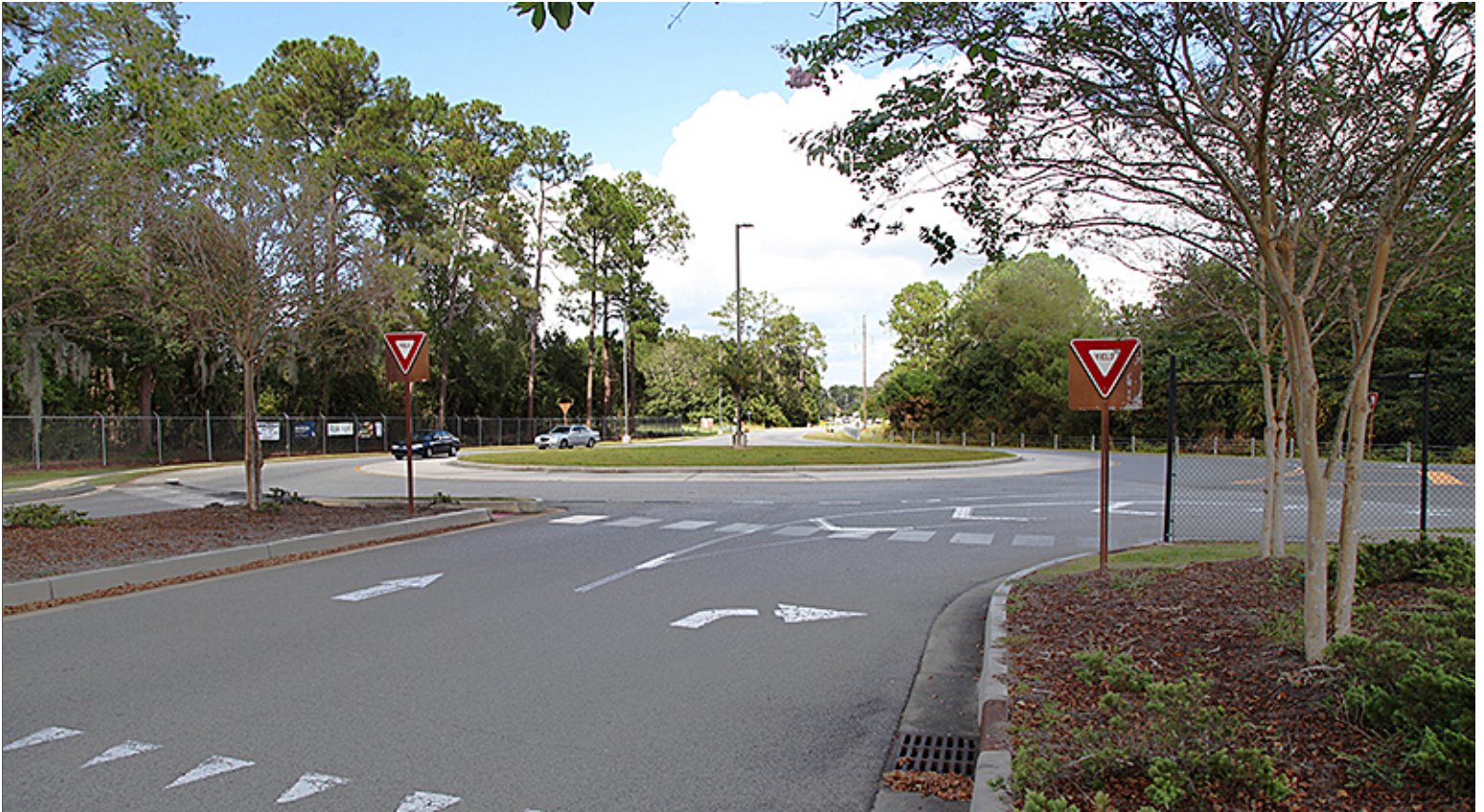
Roundabout at Davidson Road
