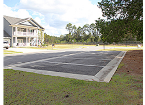
Group 4 Paving and Striping
