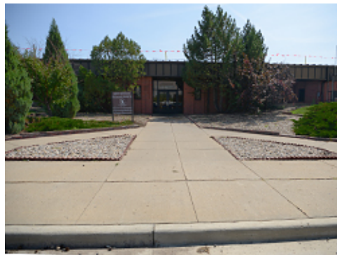
Entrance Plaza at Group 2
