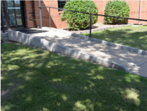
Group 1 - Ramp to Access Main Entrance
