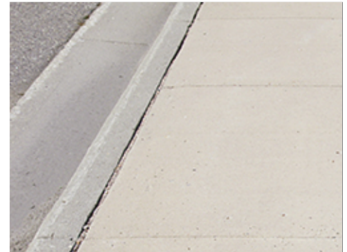
Integral Curb with Attached Sidewalk
