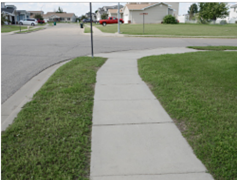
Standard Flared Curb Cut for Walkway
