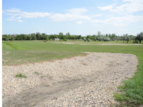
Xeriscap Drainage Swale
