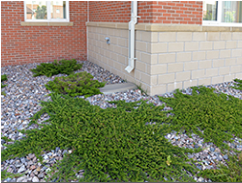
Rock Mulch at Foundation
