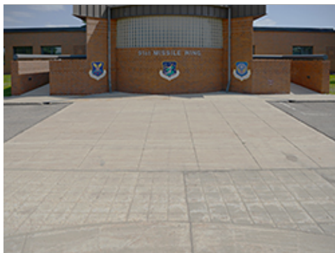
Group 1 Contrasting Paving
