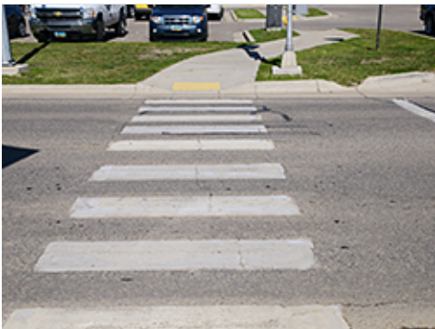
Standard Crosswalk Markings and Coloring
