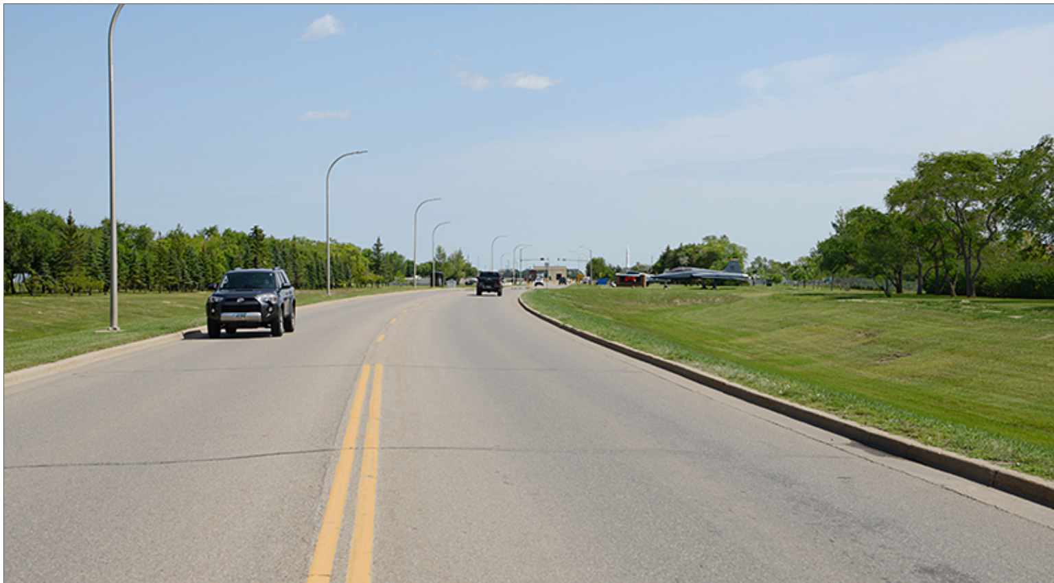
Main Arterial with Open Space Buffer and Screening Adjacent to Housing and MDG Clinic
