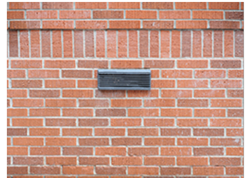
Group 1 Entrance Ramp Lighting
