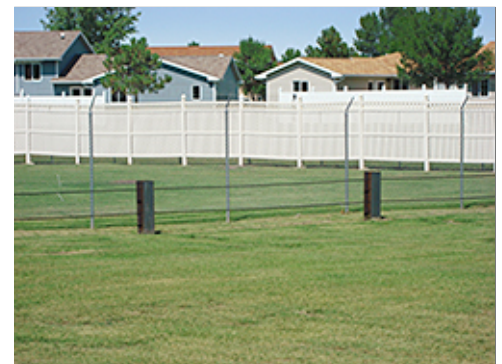
Perimeter Fence with Privacy Fence Beyond
