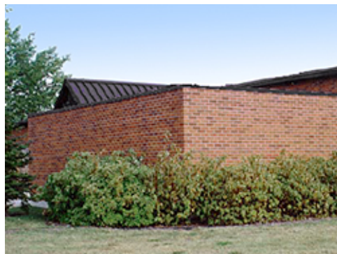
Landscaping to Soften Brick Screening
