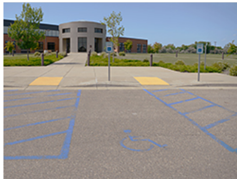
Base Standard Accessible Parking
