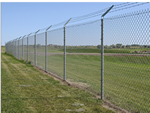
Typical Perimeter Fence
