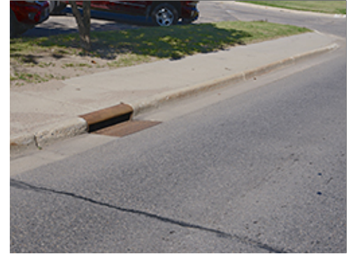
Integral Curb and Gutter
