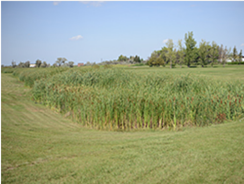
Berm and Swale to Direct Stormwater
