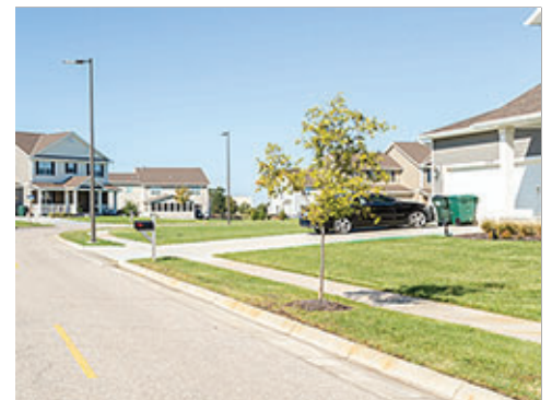
Detached Sidewalk at Group 4
