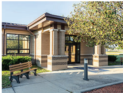
Concrete Entrance Plaza
