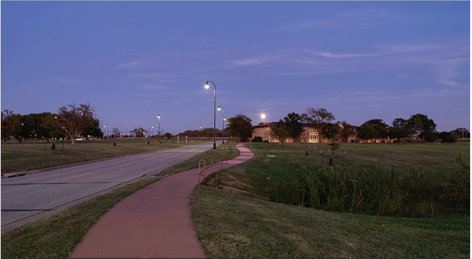
Uniform Street Lighting and Sidewalk Lighting
