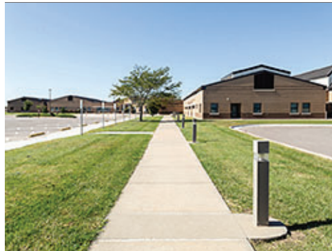
Lighted Bollards Defining Sidewalk
