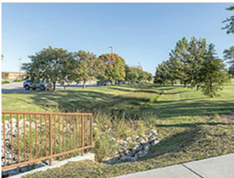
Landscaped Drainage Basin
