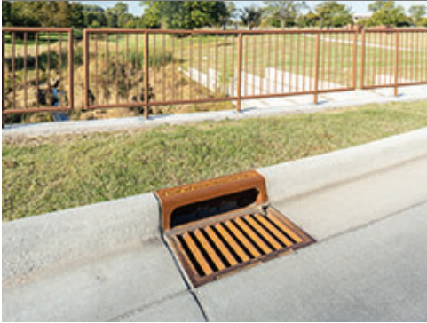
Inlet and Grate
