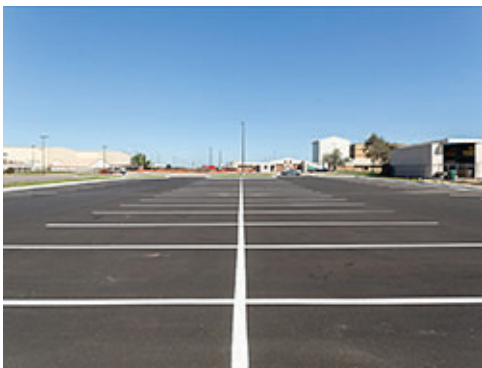
Asphaltic Concrete with White Striping
