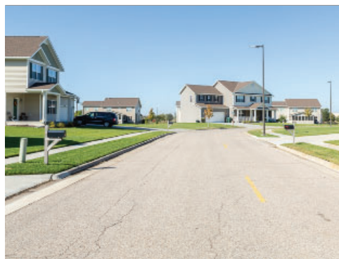
Streetscape at Family Housing
