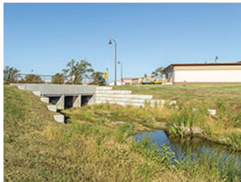
Stormwater Culvert at Street
