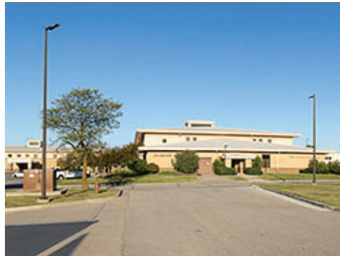
Fixtures at Group 3
