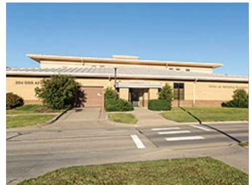
Sloped Drive and Sidewalk
