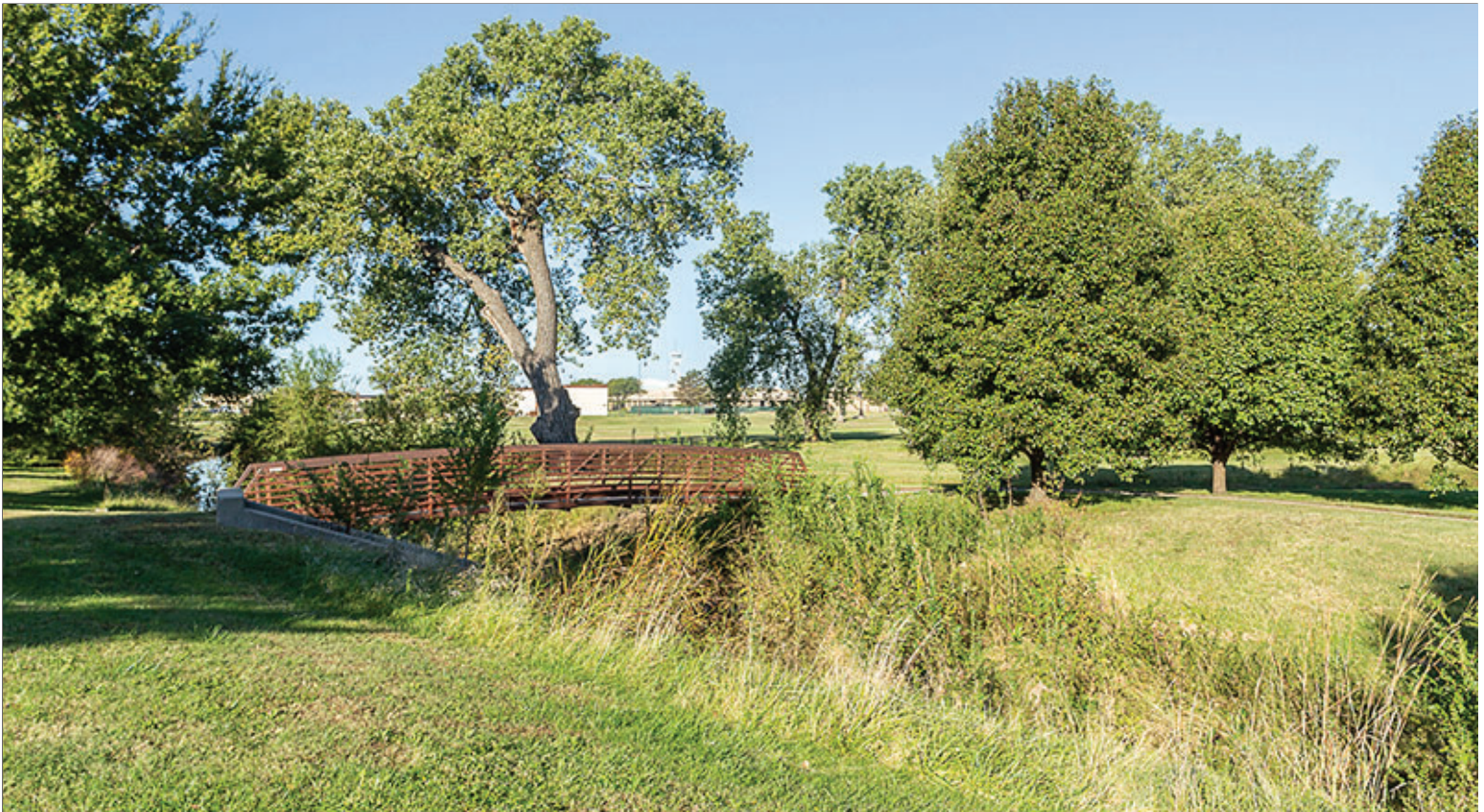
Bridge over Drainage Basin as an Amenity
