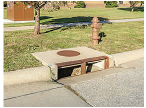
Storm Drain Inlet
