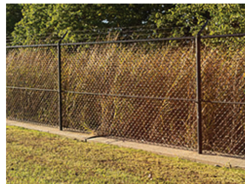
Chain Link Fencing near Group 3
