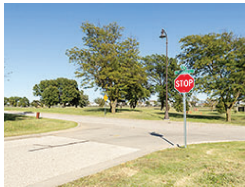
Standard Placement of Signing and Lighting
