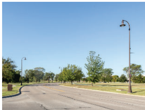
Street Light Fixtures along Special Route
