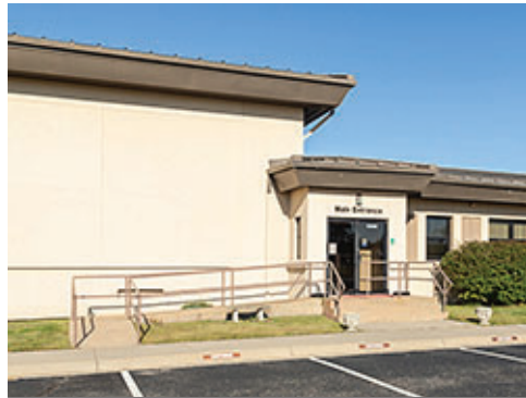
Ramp and Stair at Entrance
