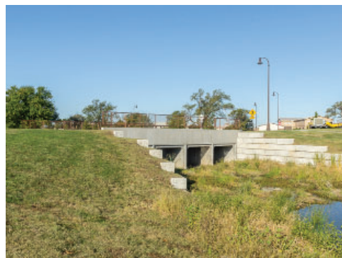
Engineered Culvert and Channel
