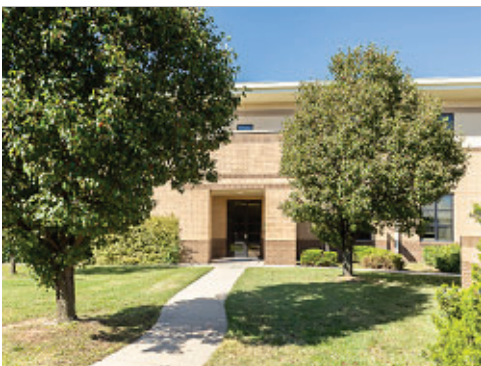
Concrete Sidewalk at Group 3
