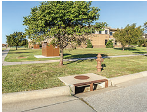
Integrated Storm Inlet
