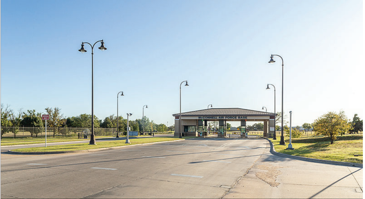
Main Gate at McConnell Group 1
