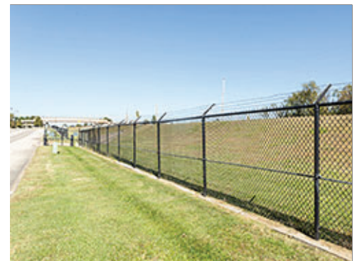
Chain Link Perimeter Fence near Group 3
