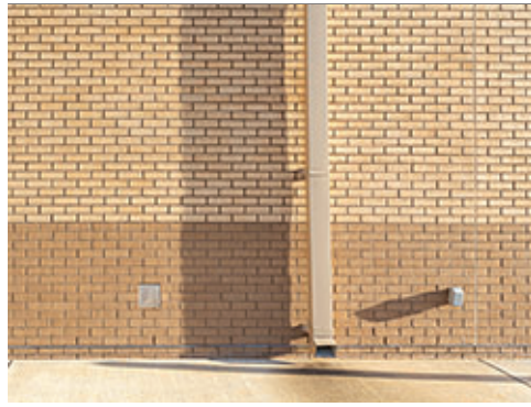
Roof Drainage to Surface Swale
