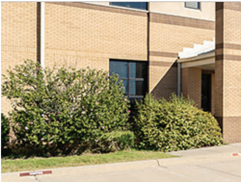
Roof Drainage Directed through Planting Bed
