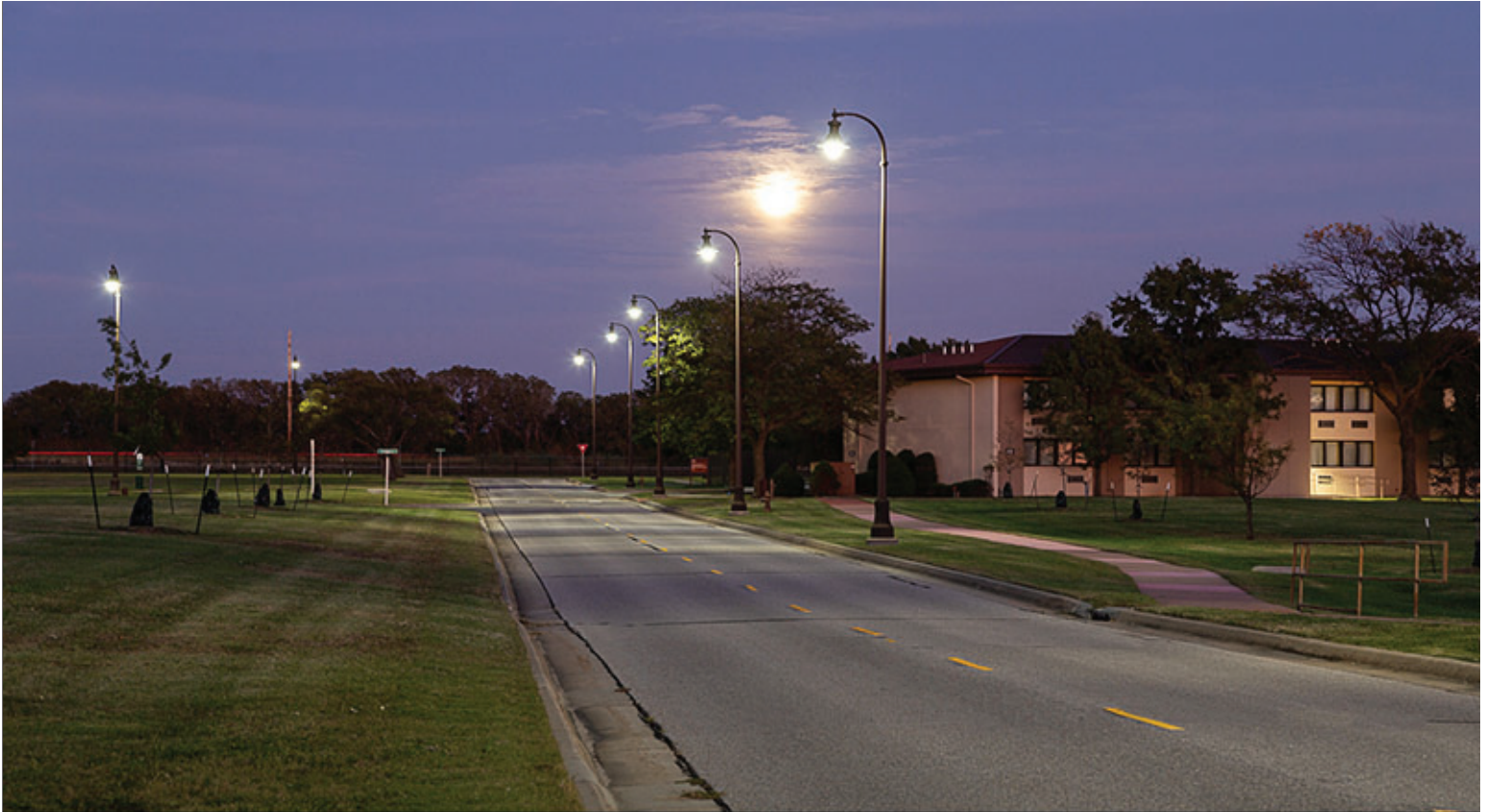
Decorative "Teardrop" Street Light Fixtures
