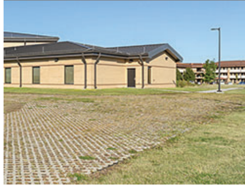
Pavers Allowing Percolation
