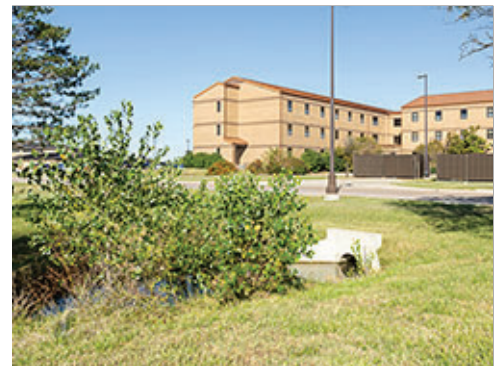
Stormwater Pipe at Street
