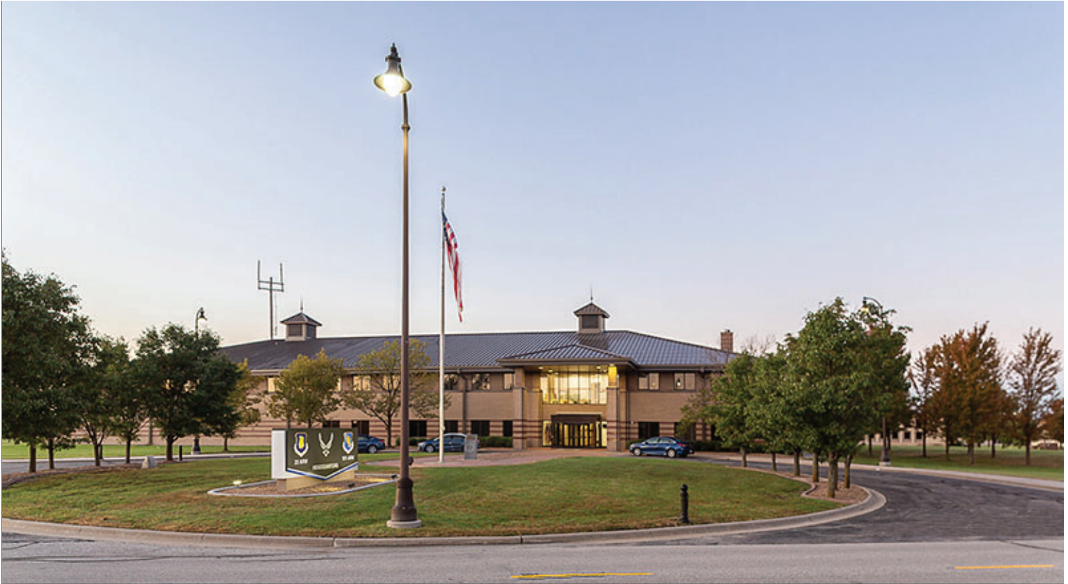
Monument Sign with Lighting
