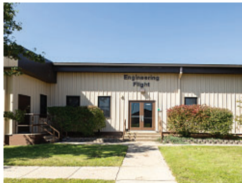
Site Cast Stair at Entrance
