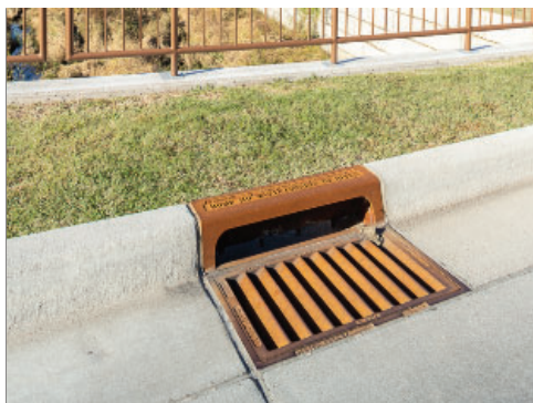
Dimensionally Coordinated Inlet
