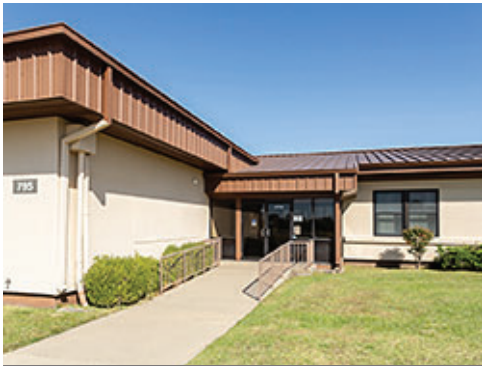
Ramp at Main Entrance
