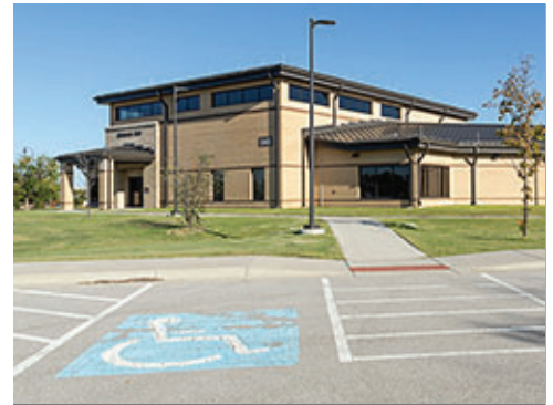
Curb Ramp at Accessible Parking
