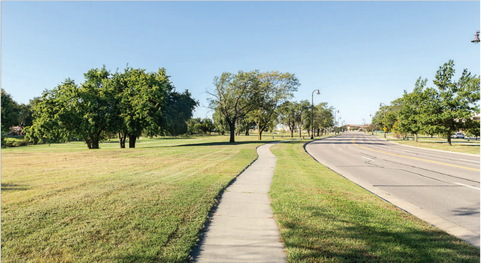
Detached Sidewalk with Grass Parkway
