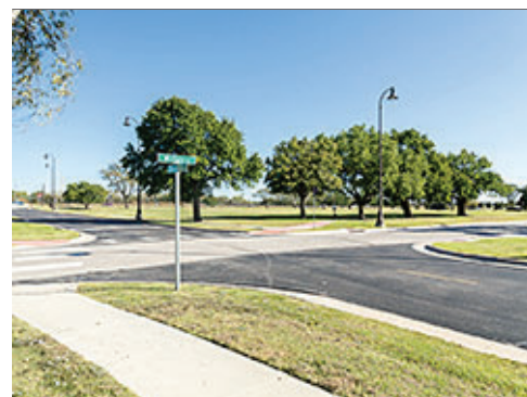
Integrated Signs and Lighting
