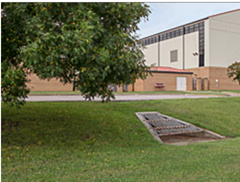
Concrete Outlet Discharge to Retention Area
