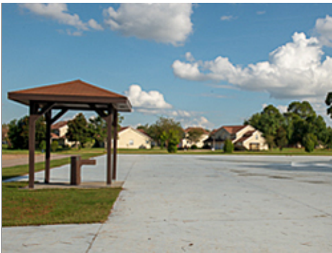
Natural Colored Concrete Paving
