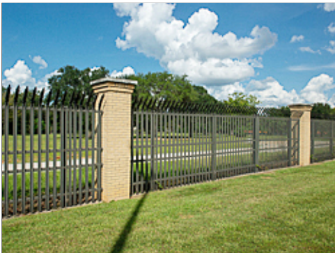
Metal Fencing with Brick Piers
