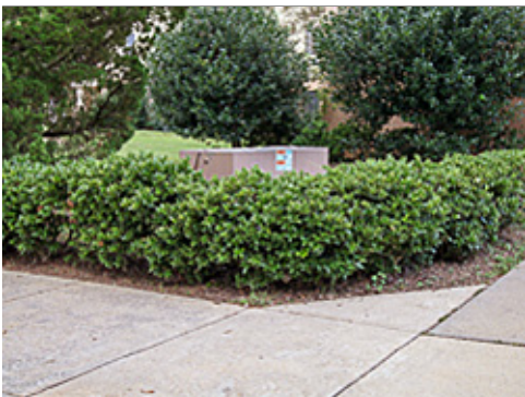
Shrubs Screening Utility Elements
