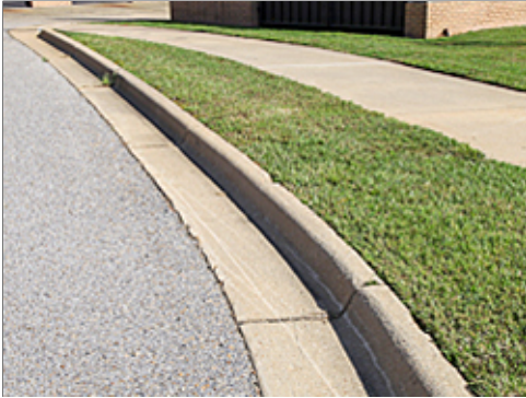
Integral curb and Gutter
