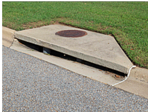
Drainage Inlet at Street
