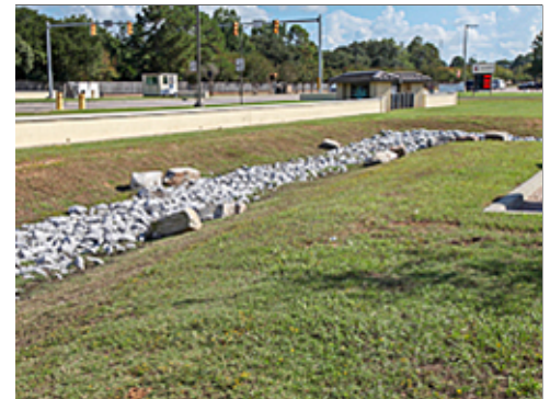
Rip Rap at Swale
