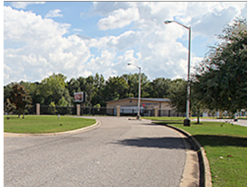
Typical Street Light Fixtures
