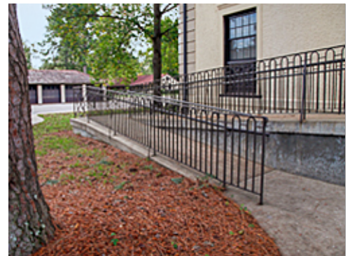
Ramp at Secondary Entrance
