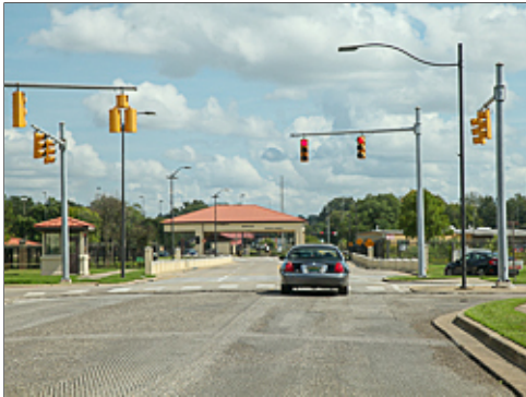
Street Lighting at Group 2
