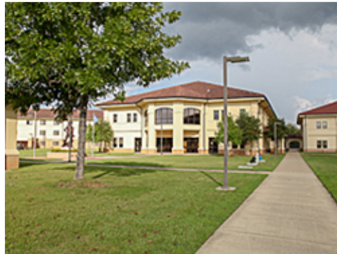
Concrete Sidewalk at Group 2
