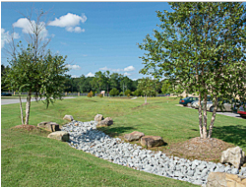
Swale Discharging to Open Space
