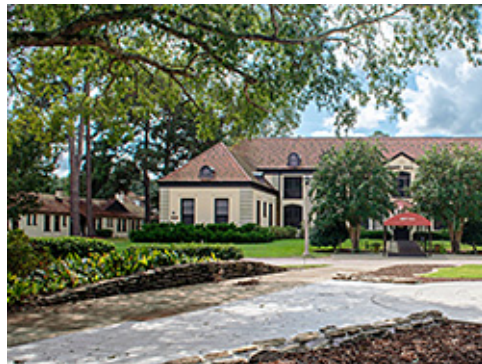
Defining Sidewalks and Features
