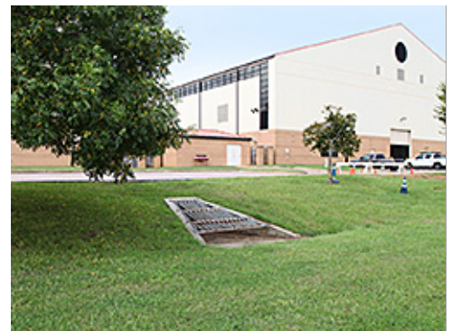
Stormwater Directed as Irrigation
