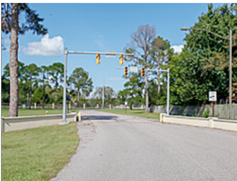
Standard Traffic Control Device
