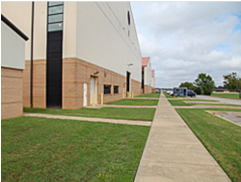
Concrete Sidewalk at Group 3
