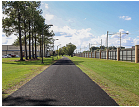
Asphalt Surface for Trail
