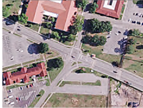
Intersection of Maxwell Blvd E and S Pine St
