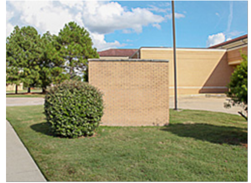
Standard Dumpster Enclosure
