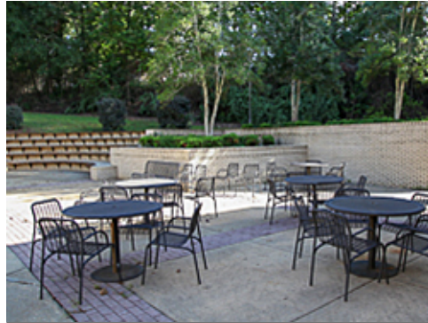
Concrete Paving with Accent Pavers
