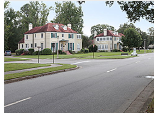
Intersection in Group 4
