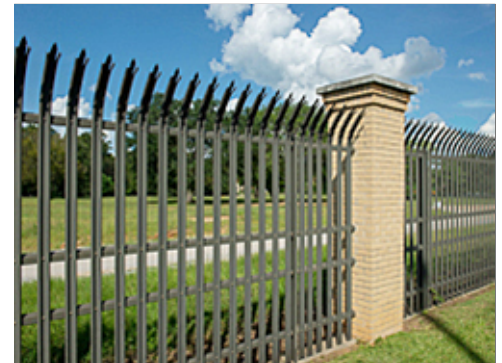
Brick Pier with Precast Cap Detail
