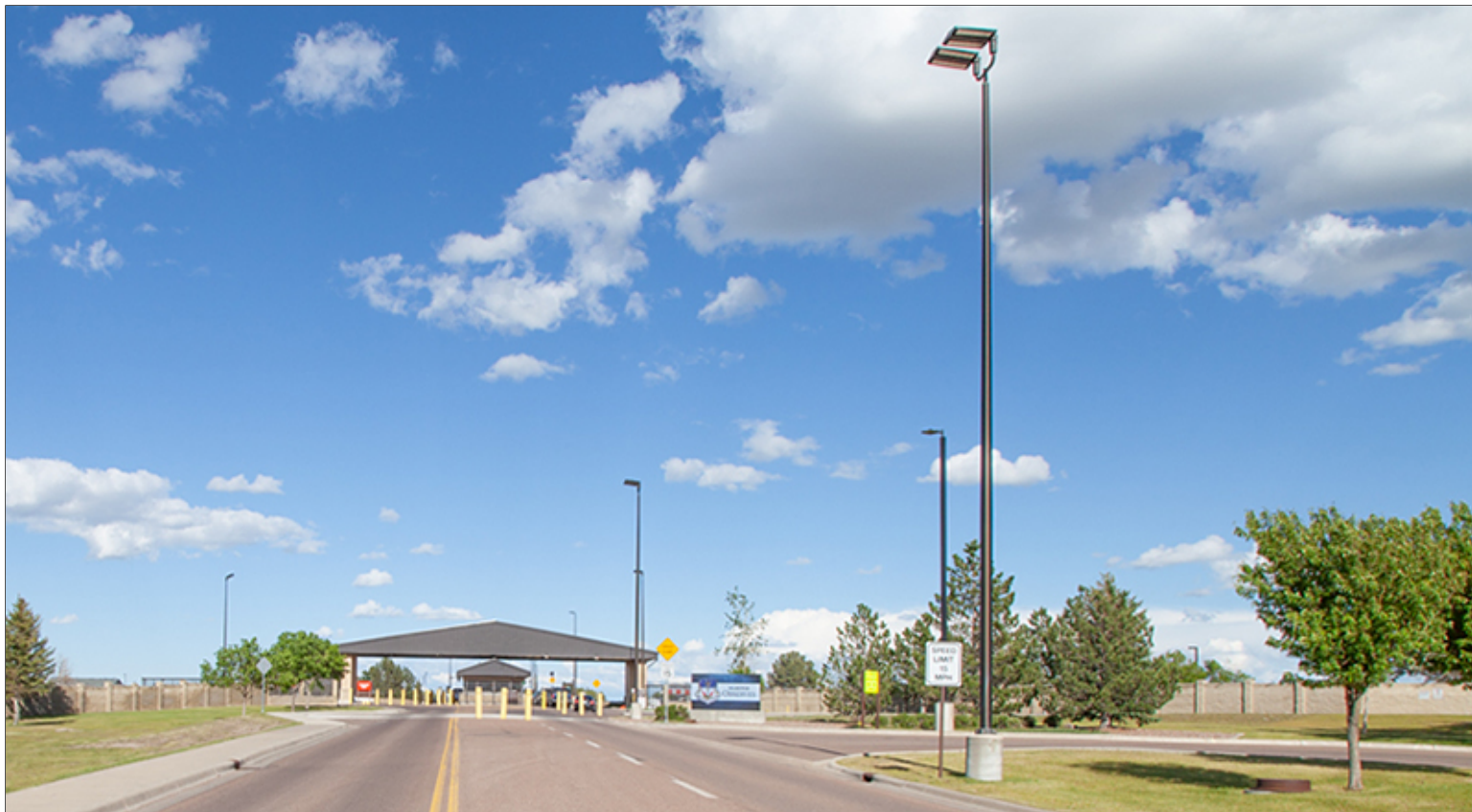
Street Light Fixtures at Group 1 Commercial Gate
