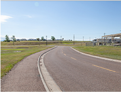
Asphaltic Paving Adjacent to Group 3
