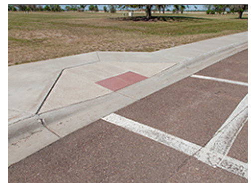
Accessible Curb Ramp
