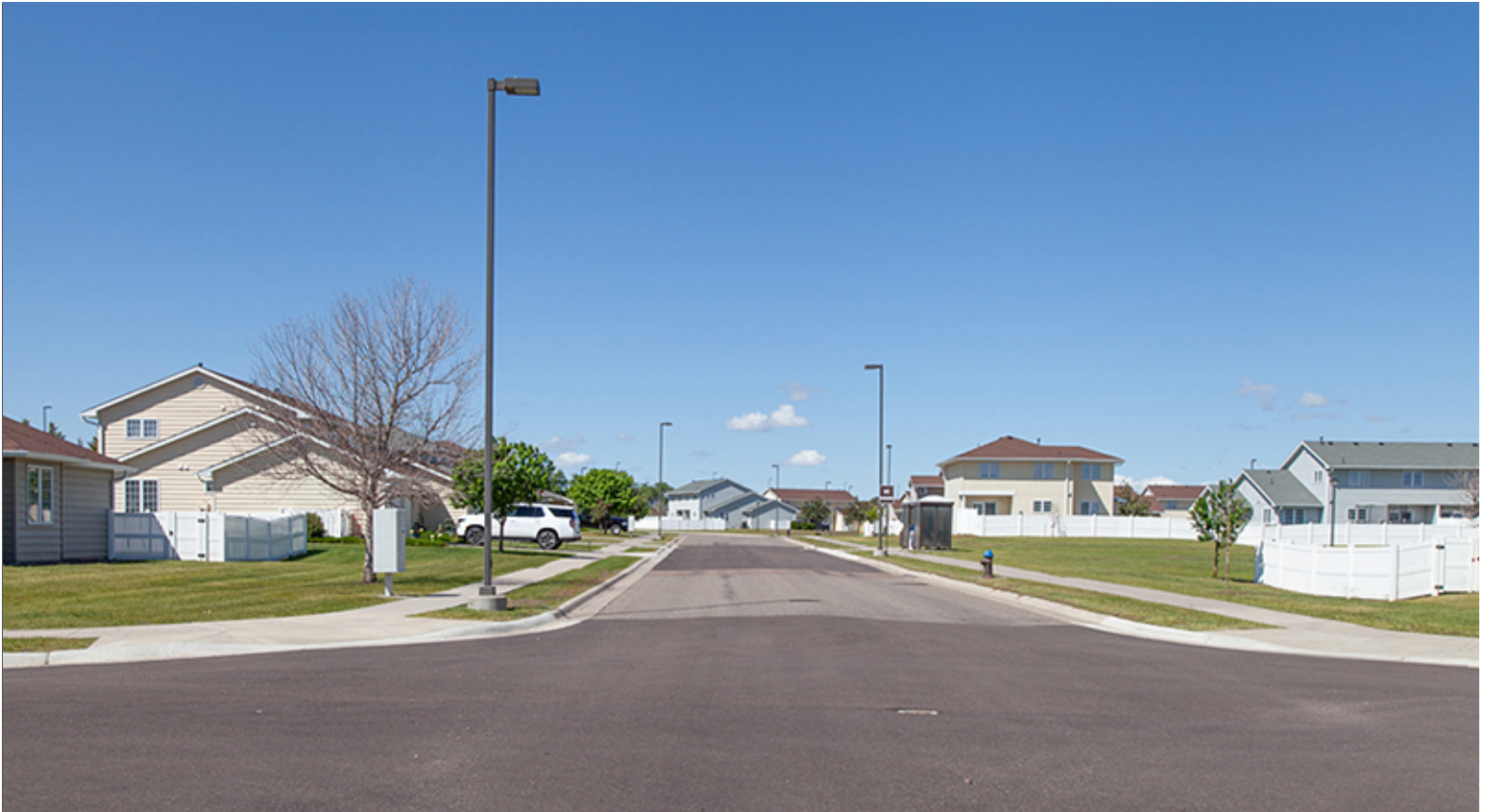
Uniform Placement of Street Light Fixtures in Group 4
