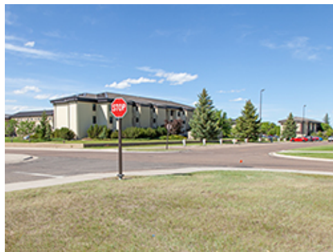
Intersection Elements at Group 2 Facility
