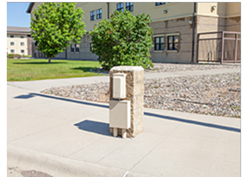
Outlets for Automobile Engine Heaters
