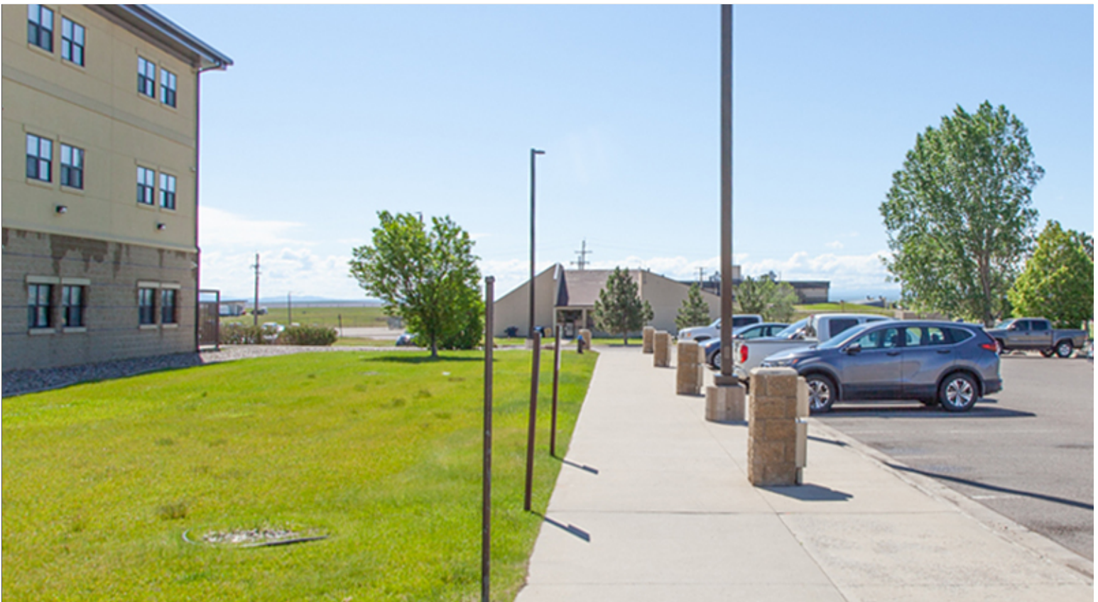
Sidewalk along Parking Lot with Width to Accommodate Bumper Overhang and Electric Service Pedestals
