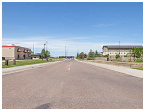
Collector at Group 2
