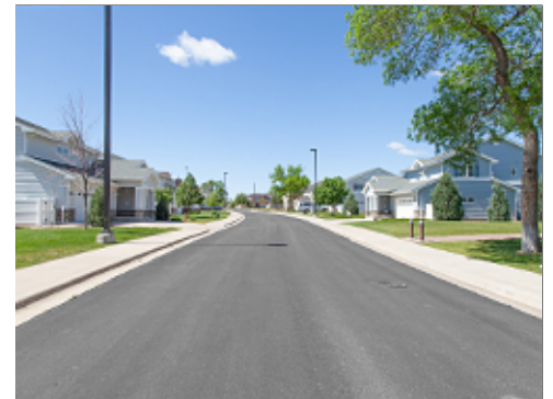
Typical Streetscape at Group 4
