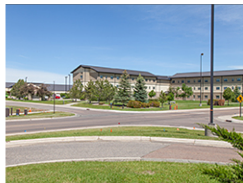
Intersection Elements at Group 2 Facility
