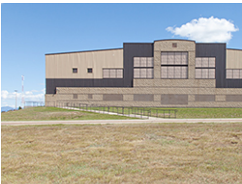
Site Ramp at Fitness Center
