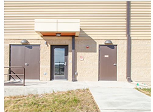
Sidewalk Width to Accommodate Equipment
