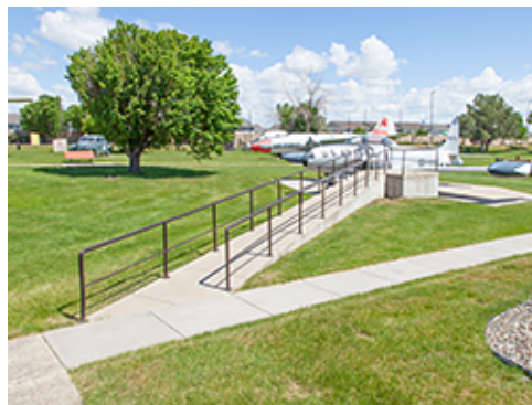
Site Ramp at Airpark
