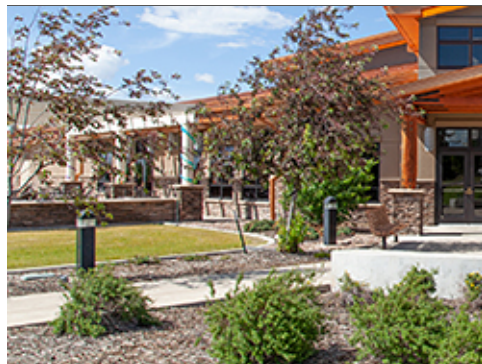
Lighted Bollards at Group 2
