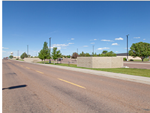
Screened Utilities at Group 2
