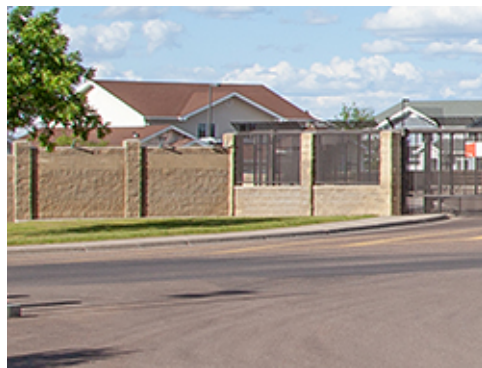
CMU Columns with Metal Fence Infill
