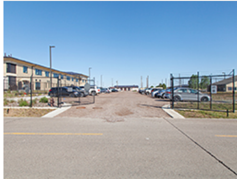
Permeable Paving at Parking Area
