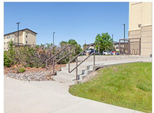
Site Stair at Dormitory
