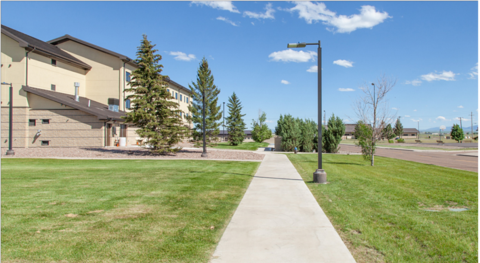
Pedestrian Scaled Light Fixture along Sidewalk at Group 2 Dormitory
