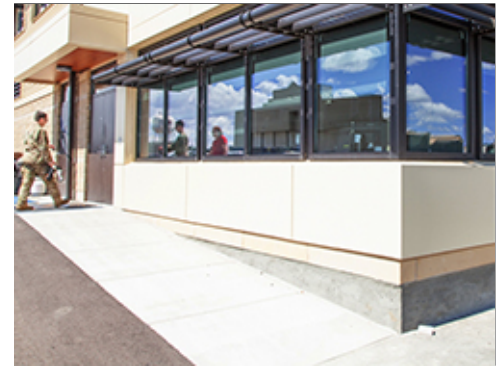
Concrete Paving at Entrance
