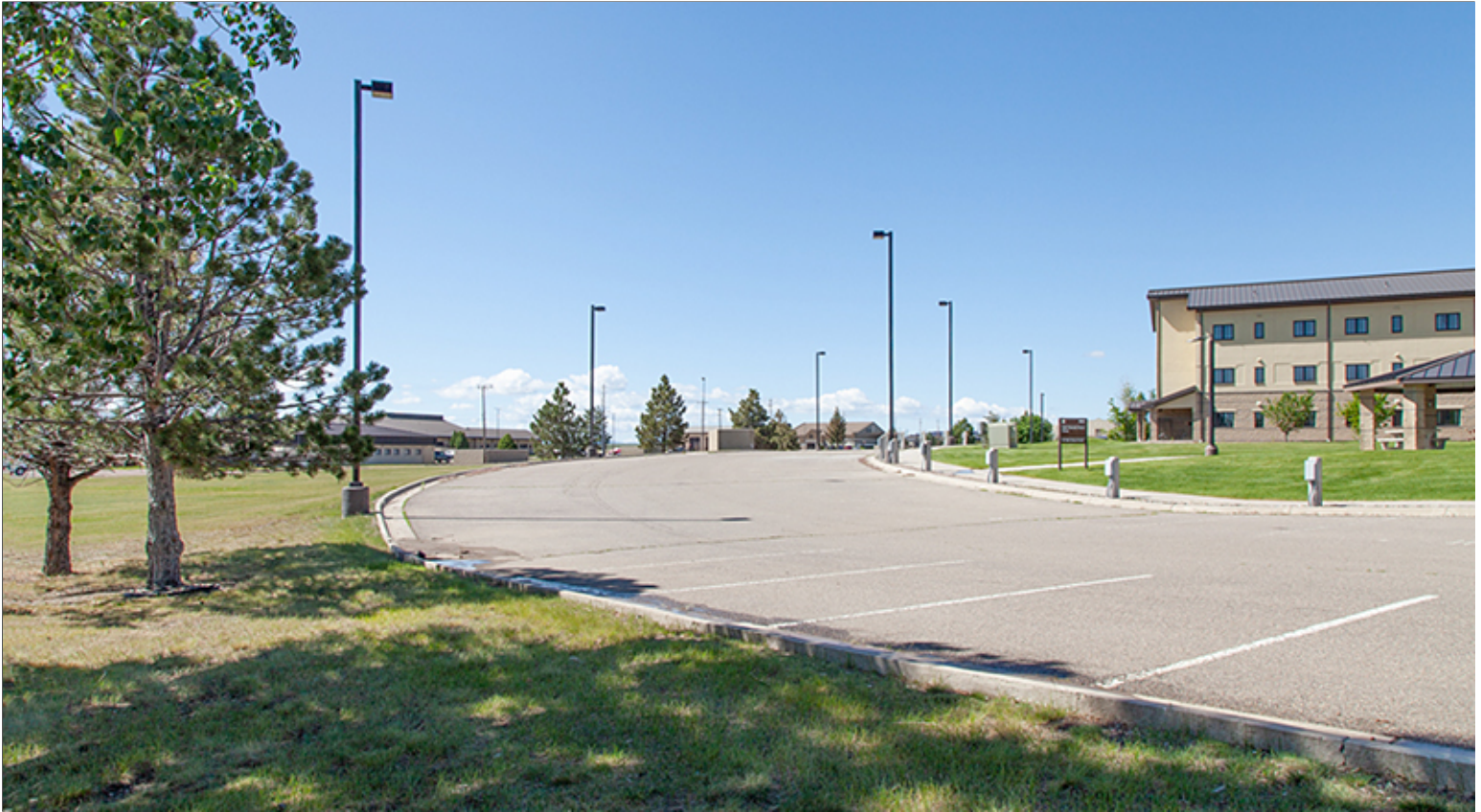
Buried Utility Service Lines at Group 2
