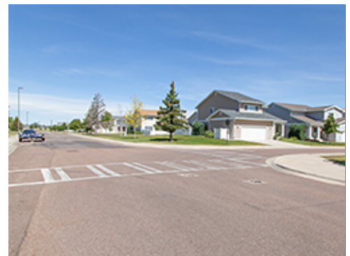
Intersection at Group 4 Housing
