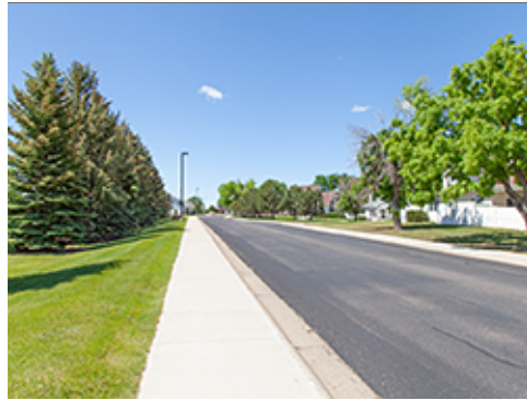
Sidewalks on Both Sides of Street in Group 4
