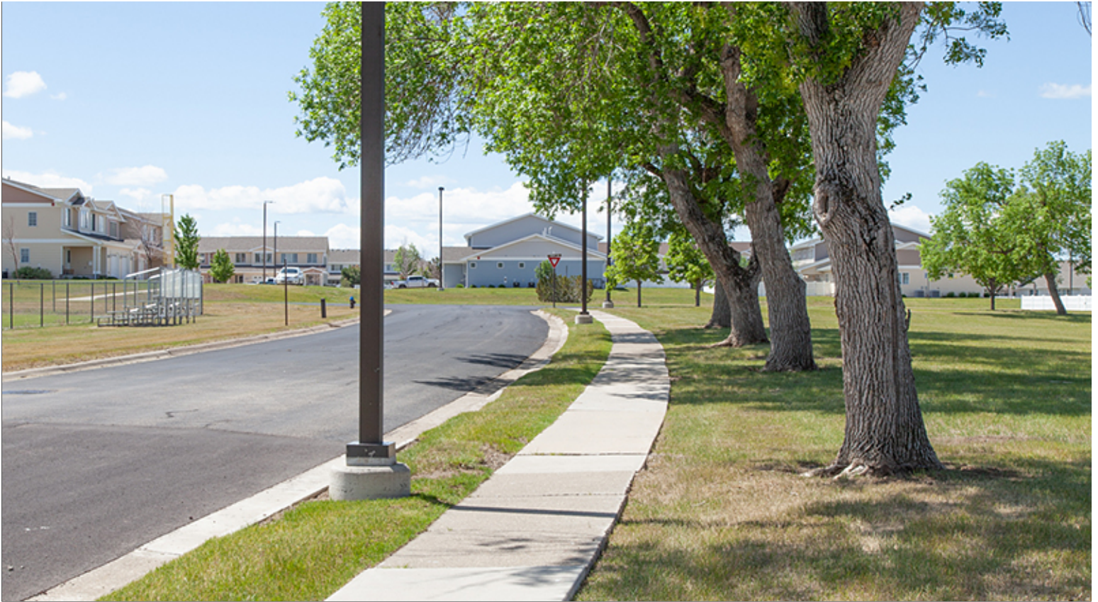
Detached Sidewalk and Coordinated Placement of Landscaping, Signs, Utility Elements and Light Fixtures
