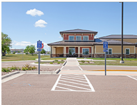
Accessible Parking Spaces
