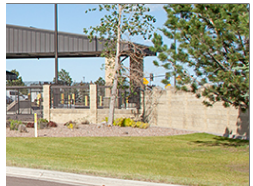
Masonry Wall with Metal Fencing
