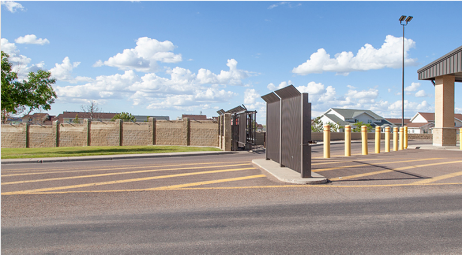
Metal Fencing with Outriggers, Metal Gate and Concrete Masonry Unit (CMU) Walls
