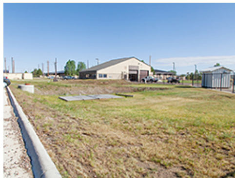
Drainage Basin at Group 3
