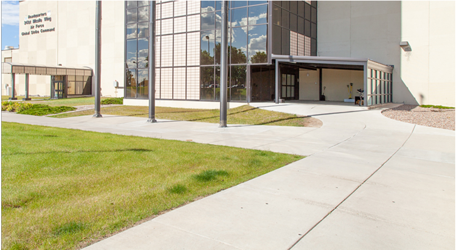
Concrete Plaza at Group 1 Entrance
