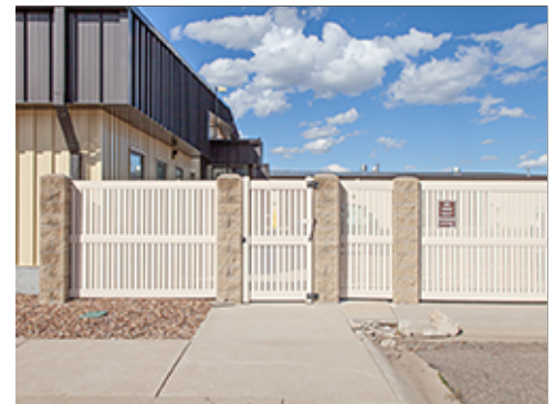
Fence with Concrete Masonry Unit Columns
