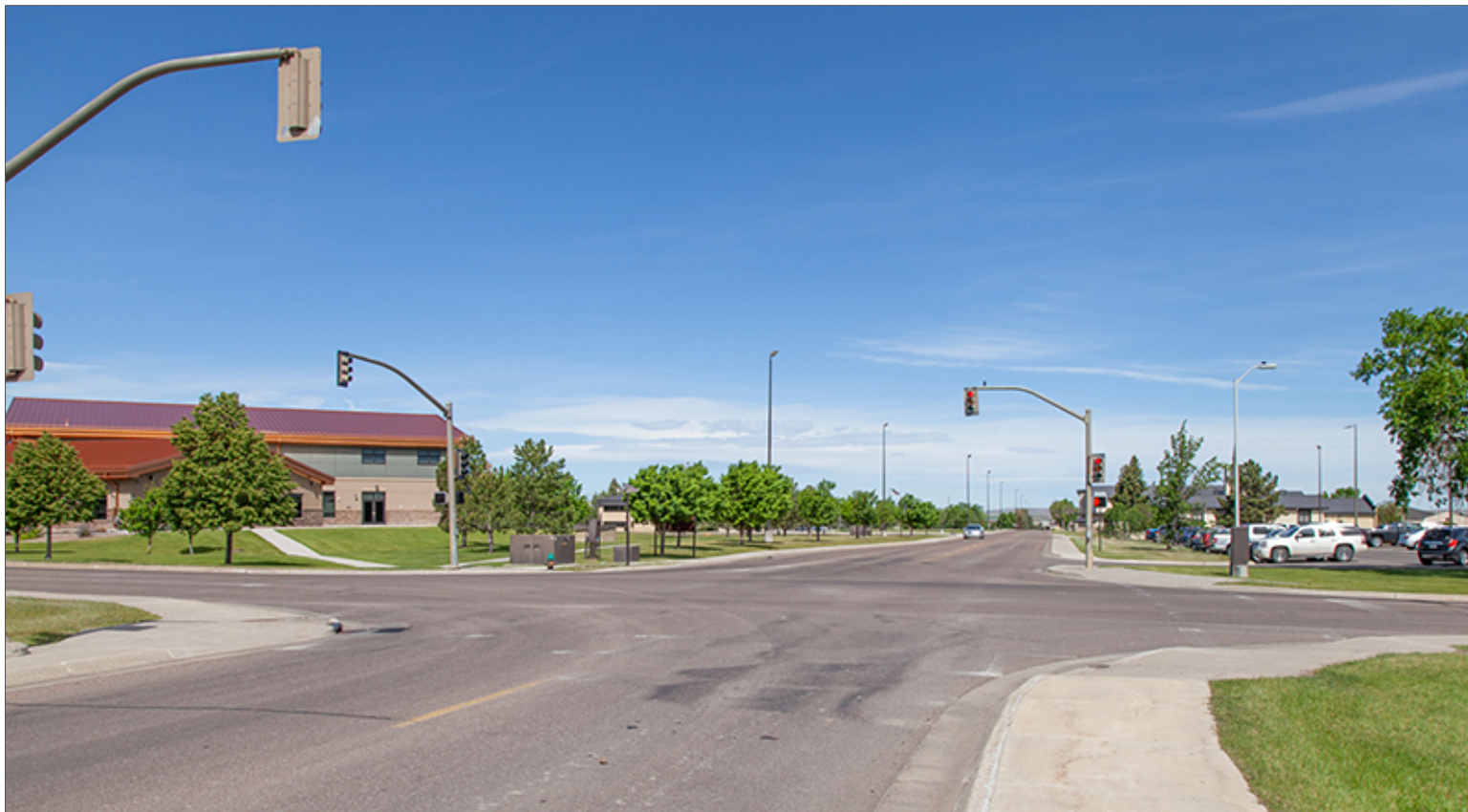
Intersection at Goddard Drive and 72nd Street North
