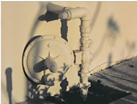
Painted Utility Components to Match Wall
