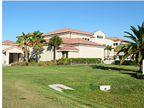
Storm Drainage Discharge Elements
