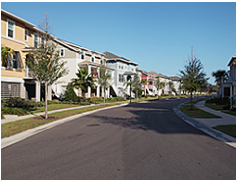
Local Street with Detached Sidewalks
