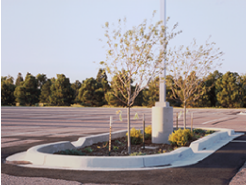
Island with Rainwater Ingress
