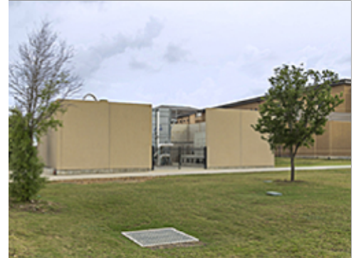
Screened Utility Yard
