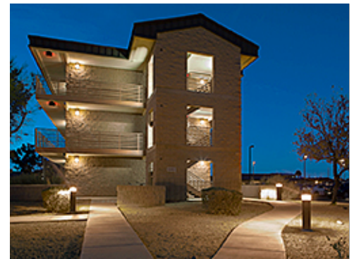
Coordinated Site and Building Lighting
