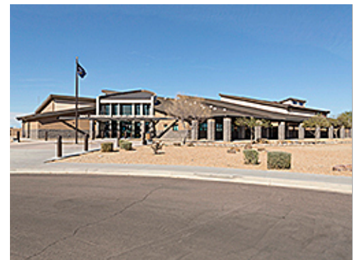
Adjacent Attached Sidewalk and Entrance
