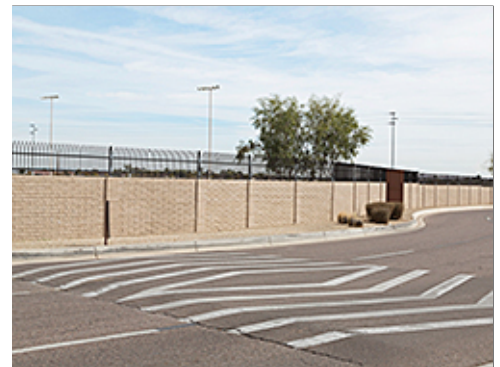
Striping at Speed Control Elements
