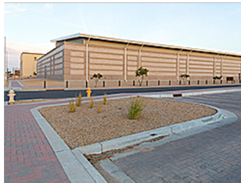
Integral Curb and Concrete Edging
