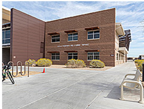
Plaza Adjacent to Primary Entrance
