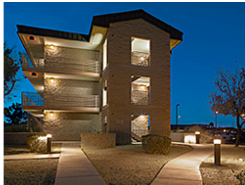
Light Bollards and Building Lighting
