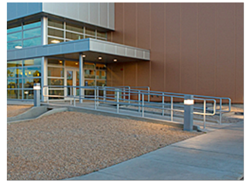
Accessible Ramp at Entrance
