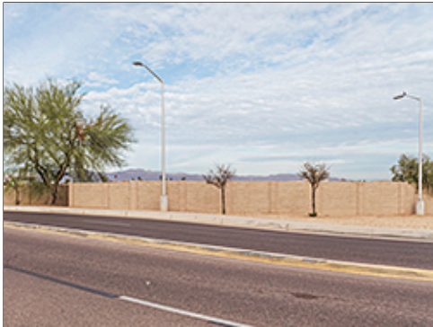
Lighting along Arterial Street
