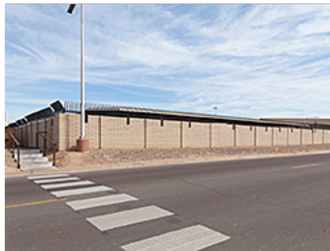
Standard Striping at Crosswalk
