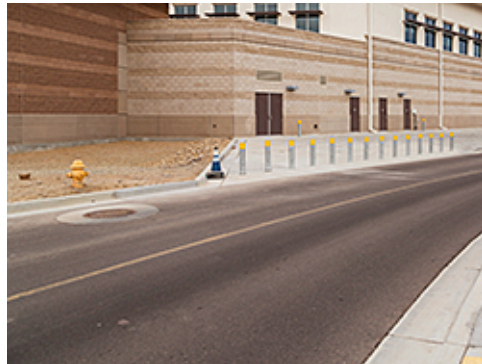
Fire Hydrant and Manhole Access
