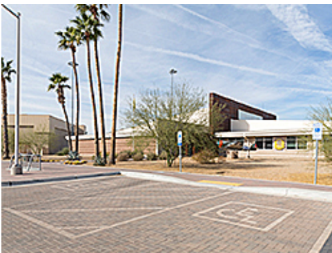
Direct Link to Main Entrance
