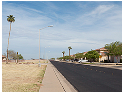
Understated Group 4 Light Fixtures
