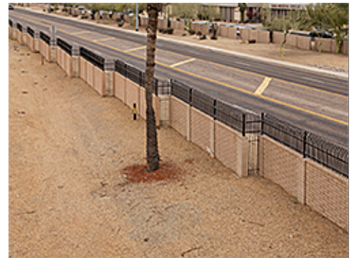
Perimeter Fence at Arterial
