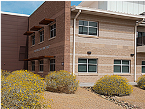
Roof Drain Discharge to Swale
