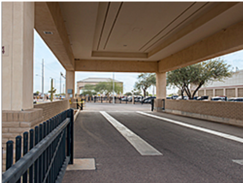
Access Control Devices
