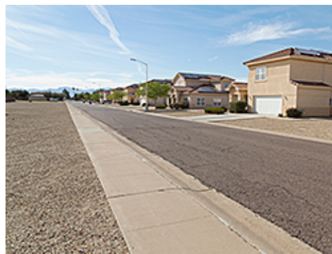
Group 4 Curb and Gutter
