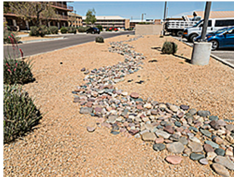
Parking Lot Drainage to Swale
