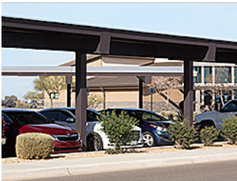
Curb and Landscape Median
