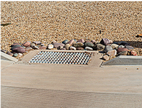
Area Drain Inlet
