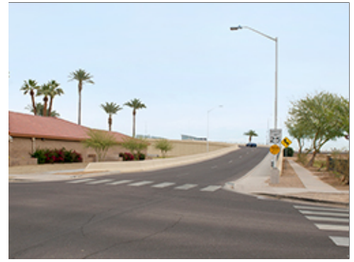
Approach to Overpass
