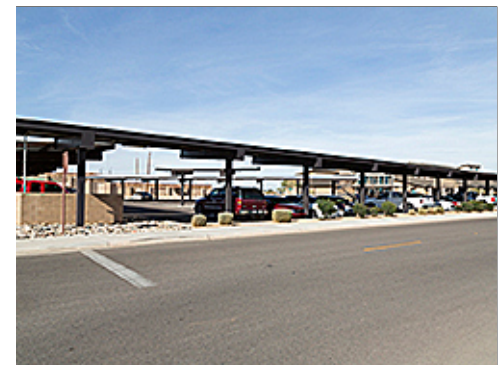
Solar Array and Shading
