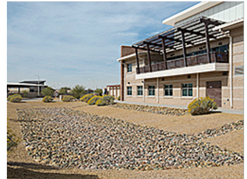
Swale discharge to Rock Mulch Basin
