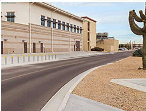
Typical Street Frontage
