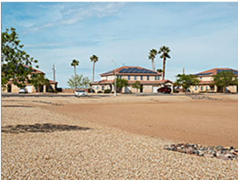
Integrated Stormwater Feature
