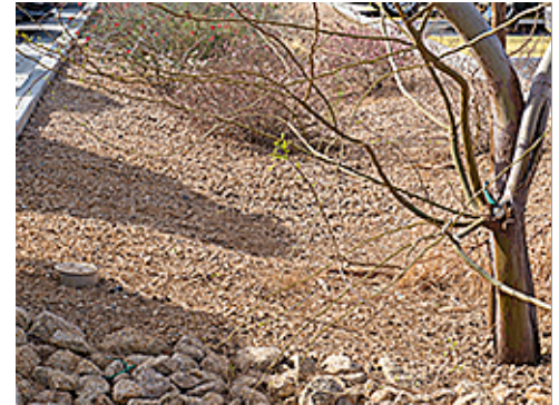
Bioswale in Central Median
