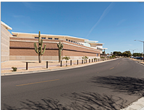
Typical Asphaltic Concrete Paving
