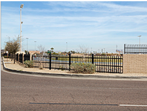
Masonry Wall and Metal Fencing
