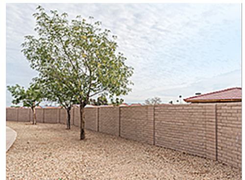
Tree Plantings Protected by Wall
