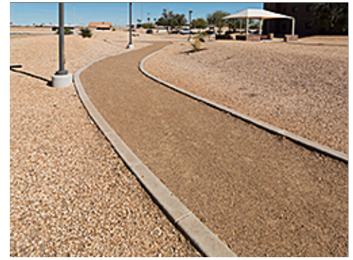
Trail Paving and Edging
