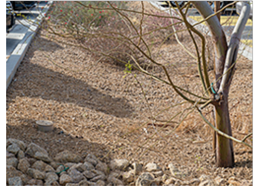
Plantings Integrated with Bioswale
