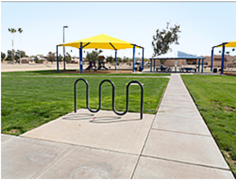
Concrete Paving at Recreation Area
