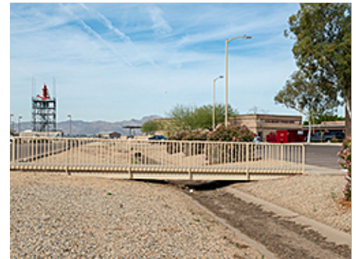
Concrete Drainage Basin
