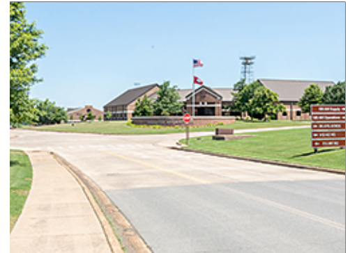
Transition in Paving at Intersection
