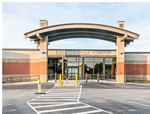
Ramp at Crosswalk/Entrance
