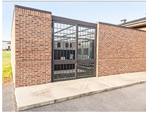
Utility Element Beyond Screenwall
