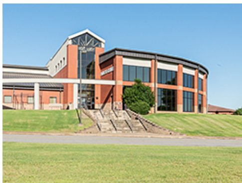
Site Stair at Entrance
