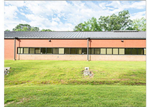
Integrated Stormwater Greenway
