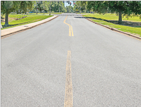
Bituminous Concrete Paving
