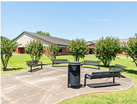
Concrete Paving in Group 2
