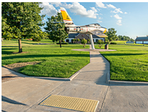
Curb Ramp at Street Crosswalk
