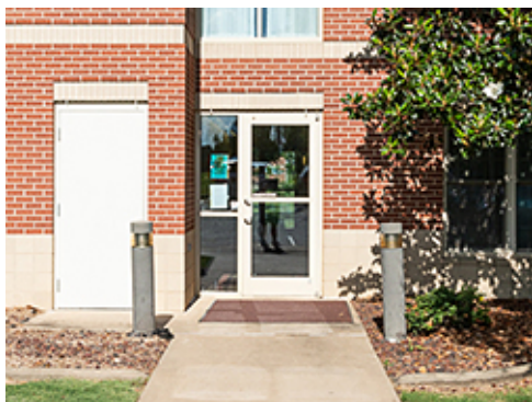
Decorative Lighted Bollards and Fixtures
