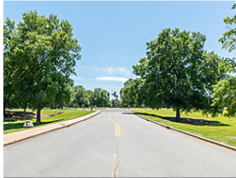
Underground Electrical Distribution
