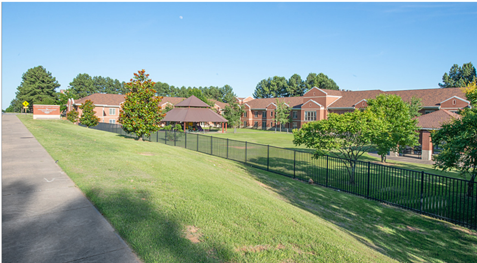
Fence at Temporary Lodging Facility
