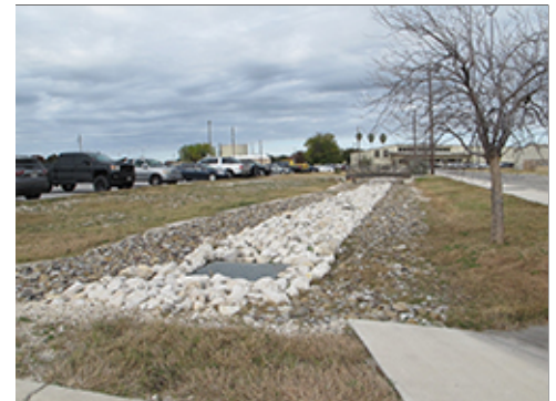
Swale Discharge to Rock Mulch Basin
