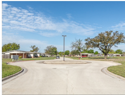
Paved Traffic Circle
