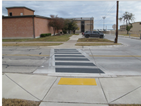
Standard Striping at Crosswalk
