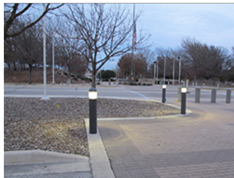
Brick Paving and Concrete Edging
