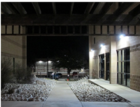
Building and Area Lighting
