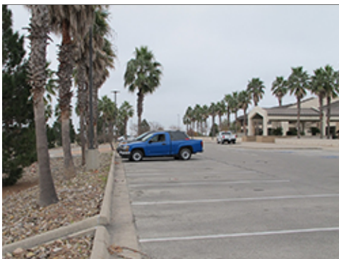
Curbing with Drainage Channel
