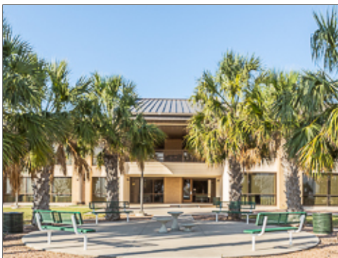
Concrete Paving and Seating
