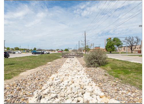
Rock-Line Drainage Swale
