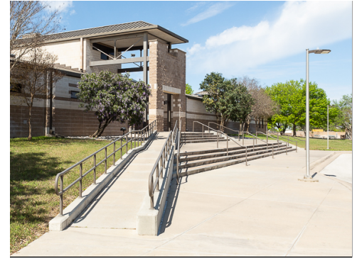
Accessible Ramp at Entrance
