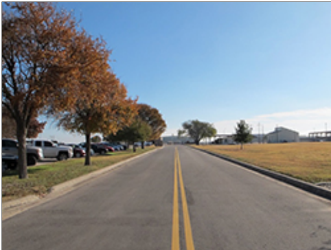
Typical Asphalt Concrete Paving
