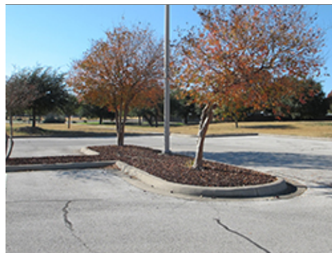
Integral Curb and Concrete Edging
