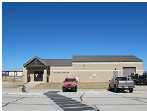
Crosswalk Striping Near Main Entrance
