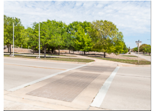
Colored Paving at Crosswalk
