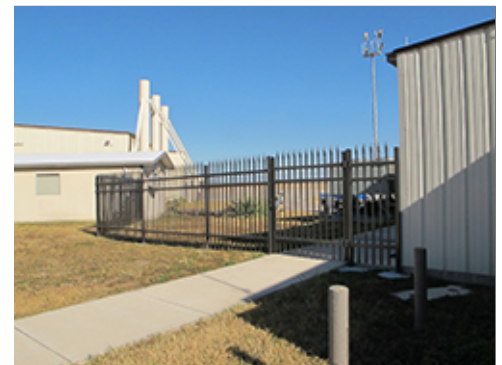
Iron Fencing at Flight Line
