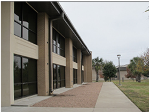
Roof Drain Discharge to Rock Mulch
