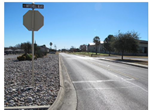
Standard Curb and Gutter
