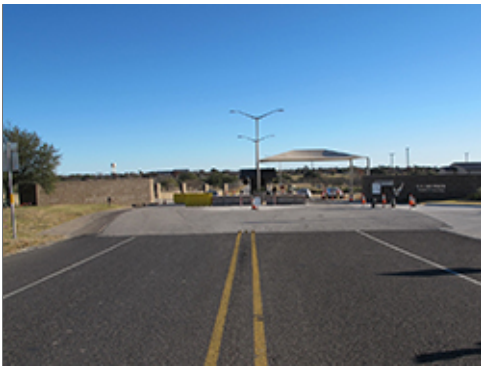
Access Control Devices
