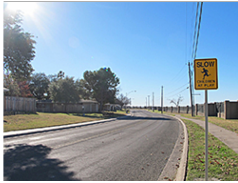
Group 4 Curb and Gutter
