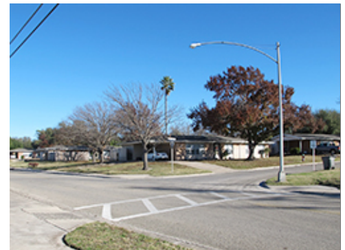
Lighting in Facility Group 4
