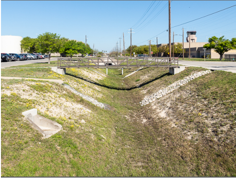
Stormwater Drainage Swale
