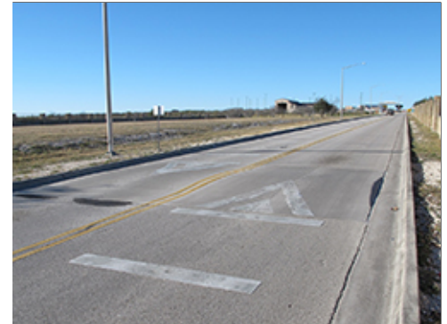
Striping at Speed Control Elements
