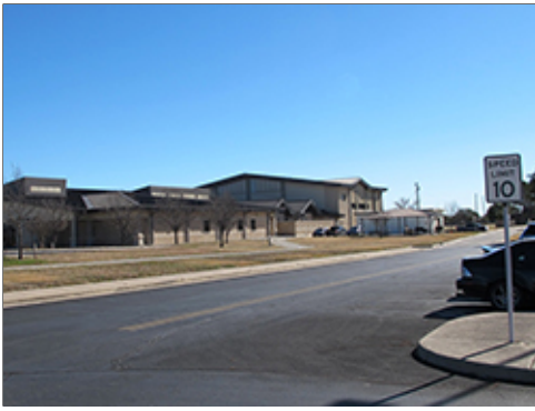
Island at Street Transition
