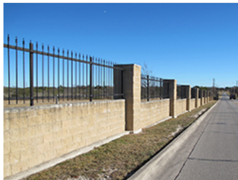
Perimeter Fence at Arterial
