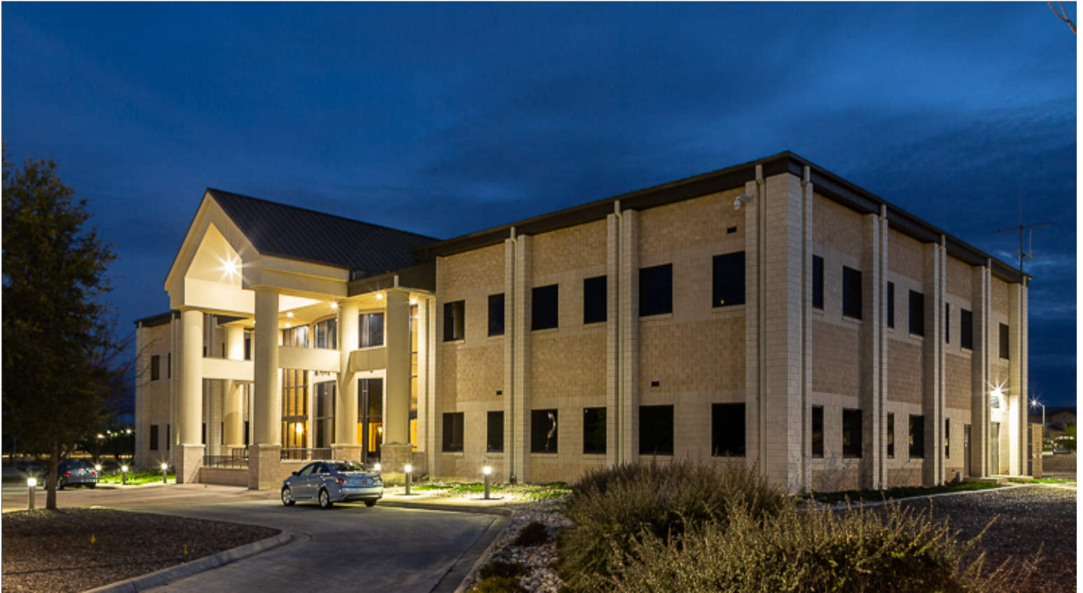
Expression of Structure in Entrance Portico and in Pilasters along Facades
