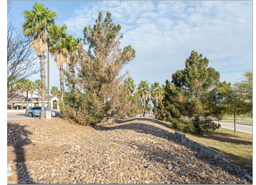
Bioswale in Median
