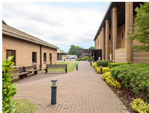
Plaza Linking Facilities
