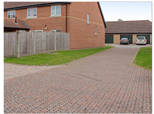
Decorative Interlocking Pavers at Group 4
