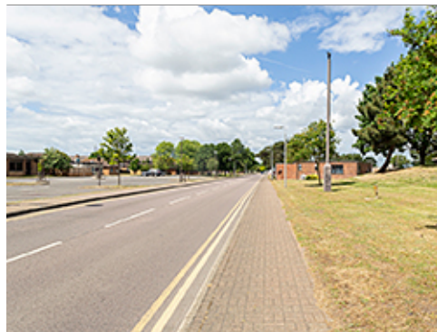
Sidewalk with Unit Pavers
