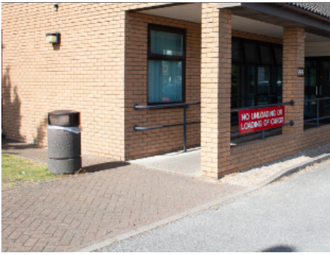
Ramp at Entry
