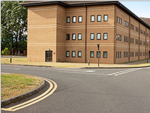
Striping at Curb
