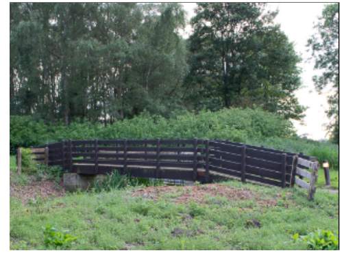
Ramp at Bridge
