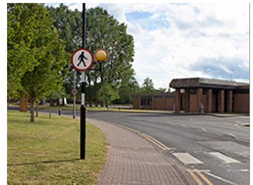
Combined Lighting and Sign Mounting
