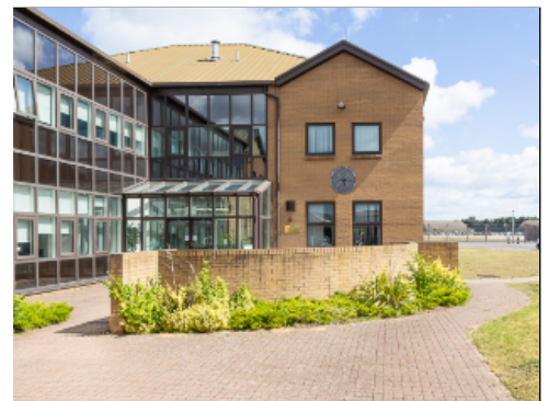
Pavers and Screen Wall
