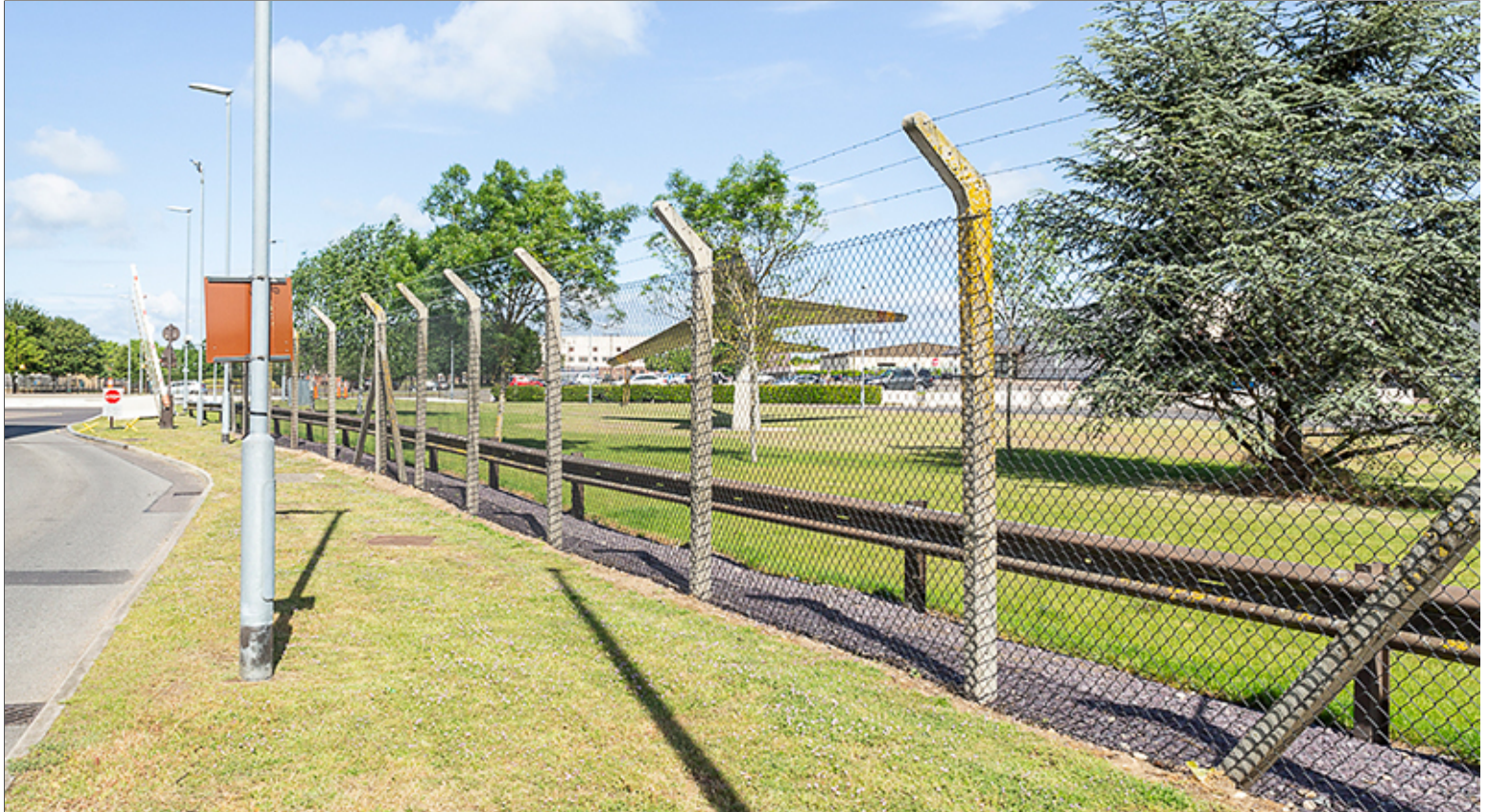
Perimeter Fence Adjacent to Main Gate
