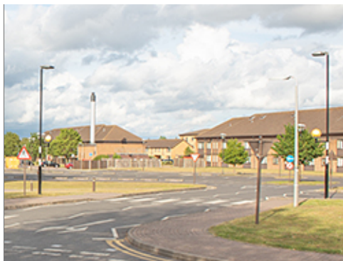
Buried Utility Lines
