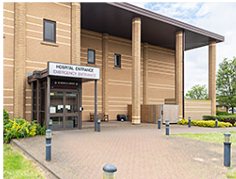
Plaza at Group 1 Entrance
