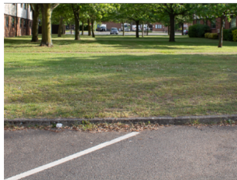
Concrete Curb at Grass
