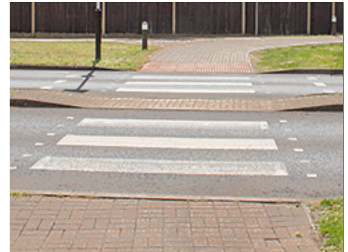
Curb Ramp at Crosswalk
