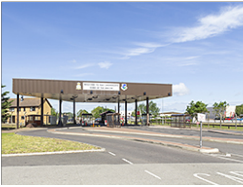
Arterial at Main Gate
