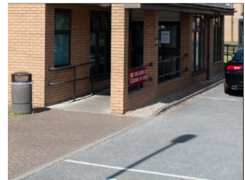
Lowered Curb for Access
