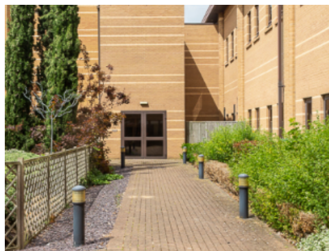
Bollard Lights at Hospital
