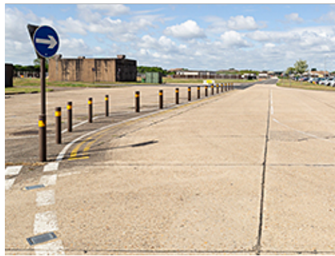
Concrete Paving at Group 3
