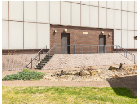
Stairs to Pavilion
