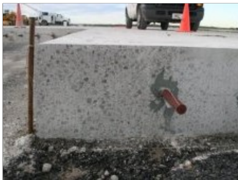
Dowel - Concrete Pavement
