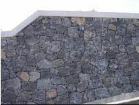
Azorean Stone Wall with Concrete Cap
