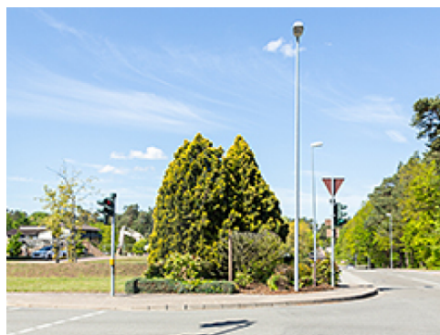
Coordinated Placement of Poles
