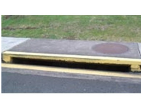
Typical Storm Drain
