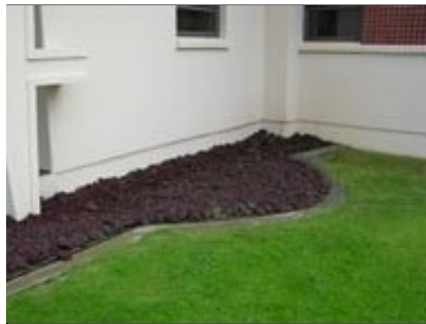
Rock Mulch at Foundation Wall
