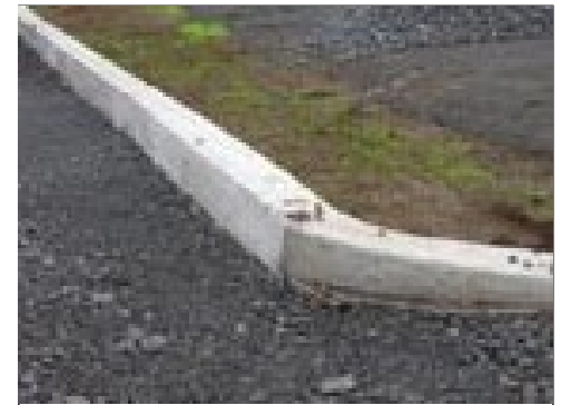
Cast in Place Curb
