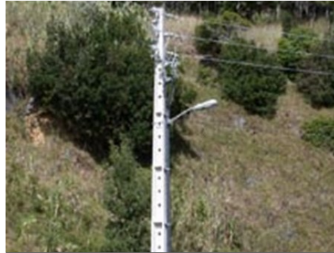
Replace Overhead Distribution
