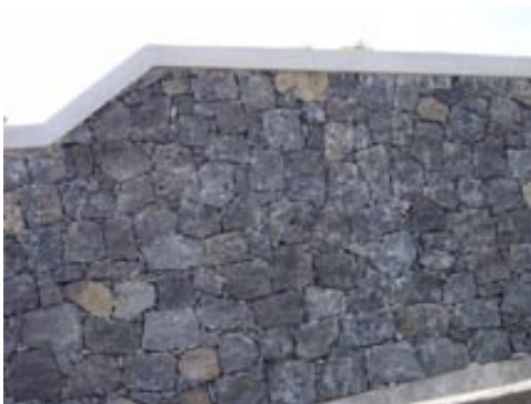
Azorean Stone Wall with Concrete Cap
