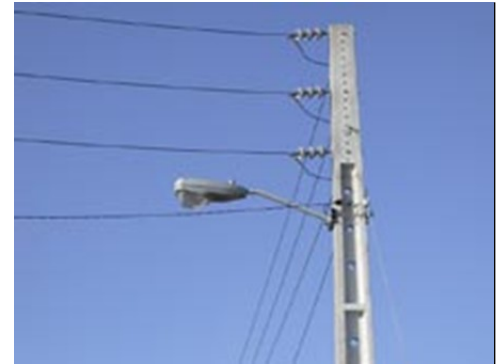
Existing Streetlight to be Replaced by LED
