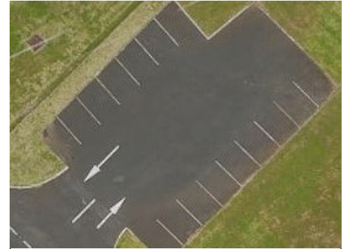
Typical Bituminous Paving
