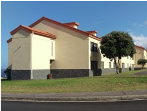
Varied Wall and Roof Lines Are Less Institutional
