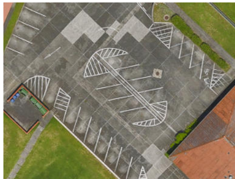
Integrated Concrete Pads
