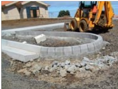
Mountable Curb and Header Curb
