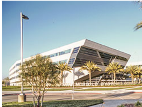
Parking Lot Fixture
