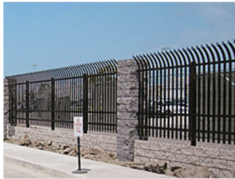
Masonry Piers and Low Wall with Metal Fence
