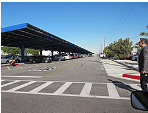
Coordinated Structure and Parking
