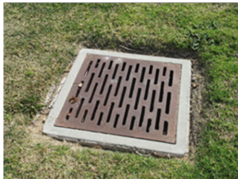
Storm Drain Inlet
