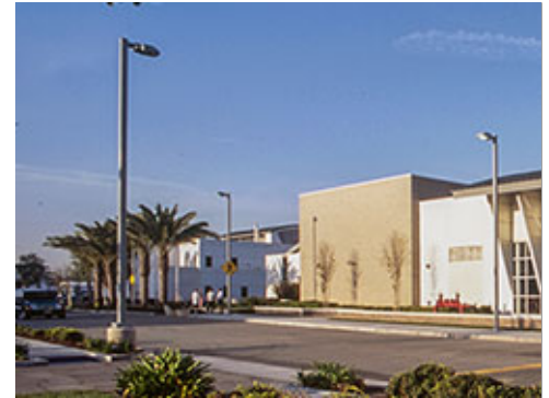
Local Street Lighting
