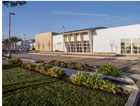
Defined Edge along Curb
