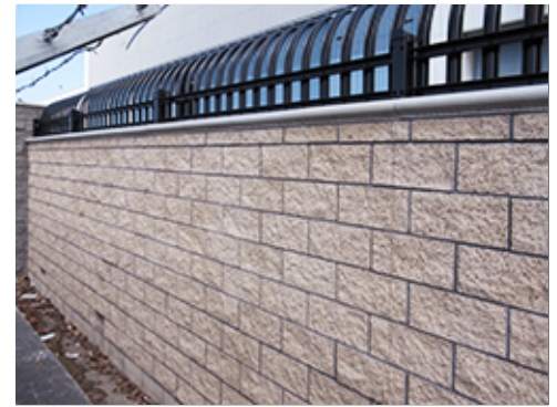
Masonry Wall with Metal Outriggers
