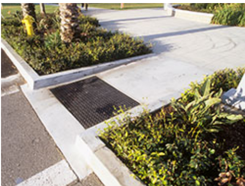
Accessible Curb Cut
