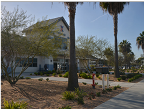
Swale in Landscape Area
