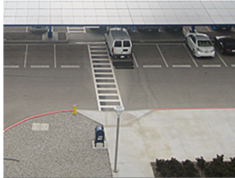
White Striping at Crosswalk
