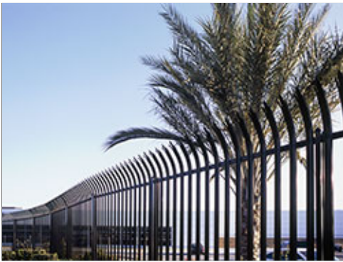
Metal Posts and Fence
