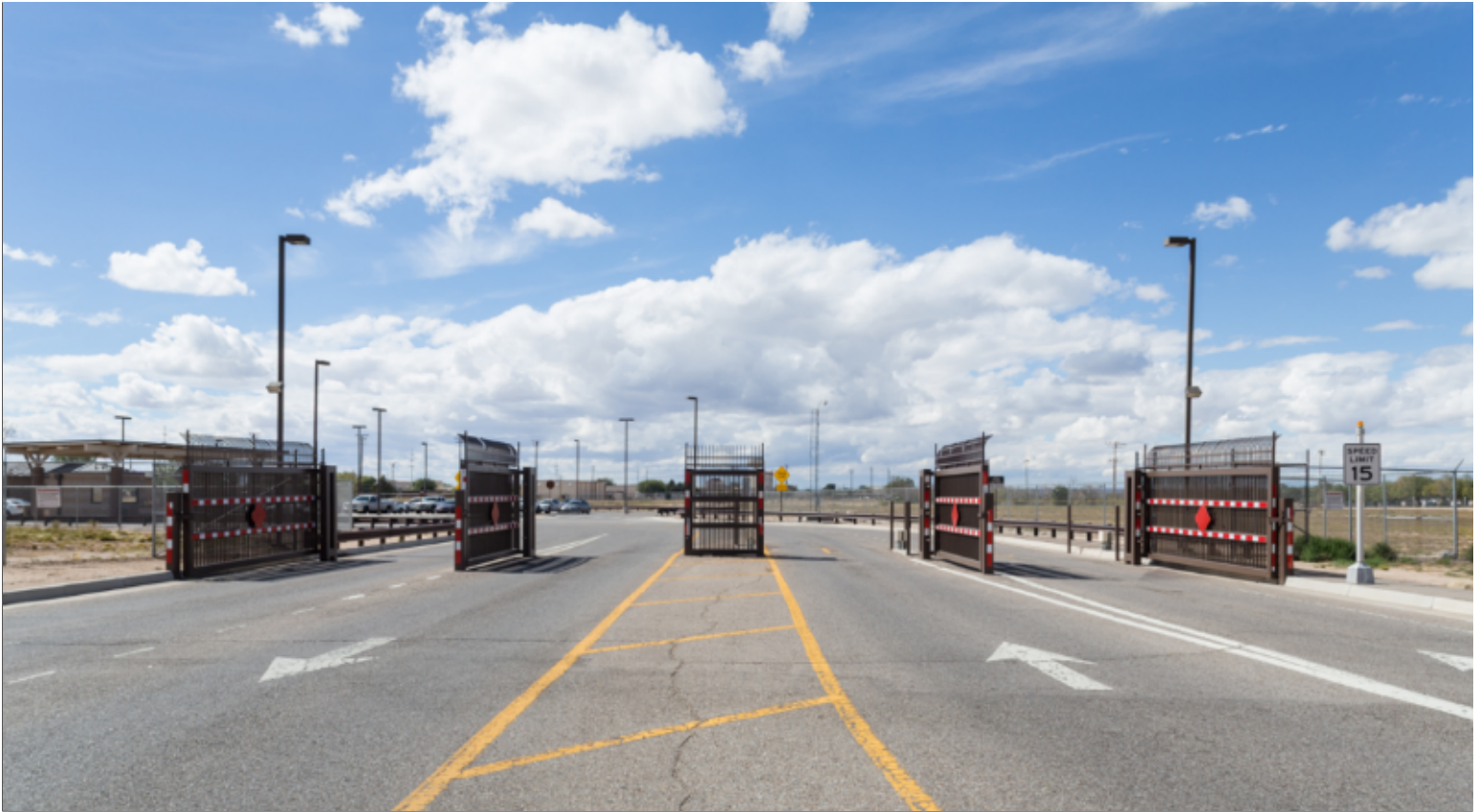
Security Gates Giving Access to and from Inspection Stations at Truman Gate
