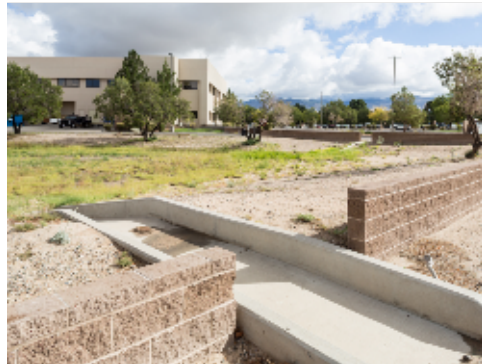
Drain to Retention Pond
