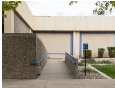
Accessible Ramp to Building Entrance
