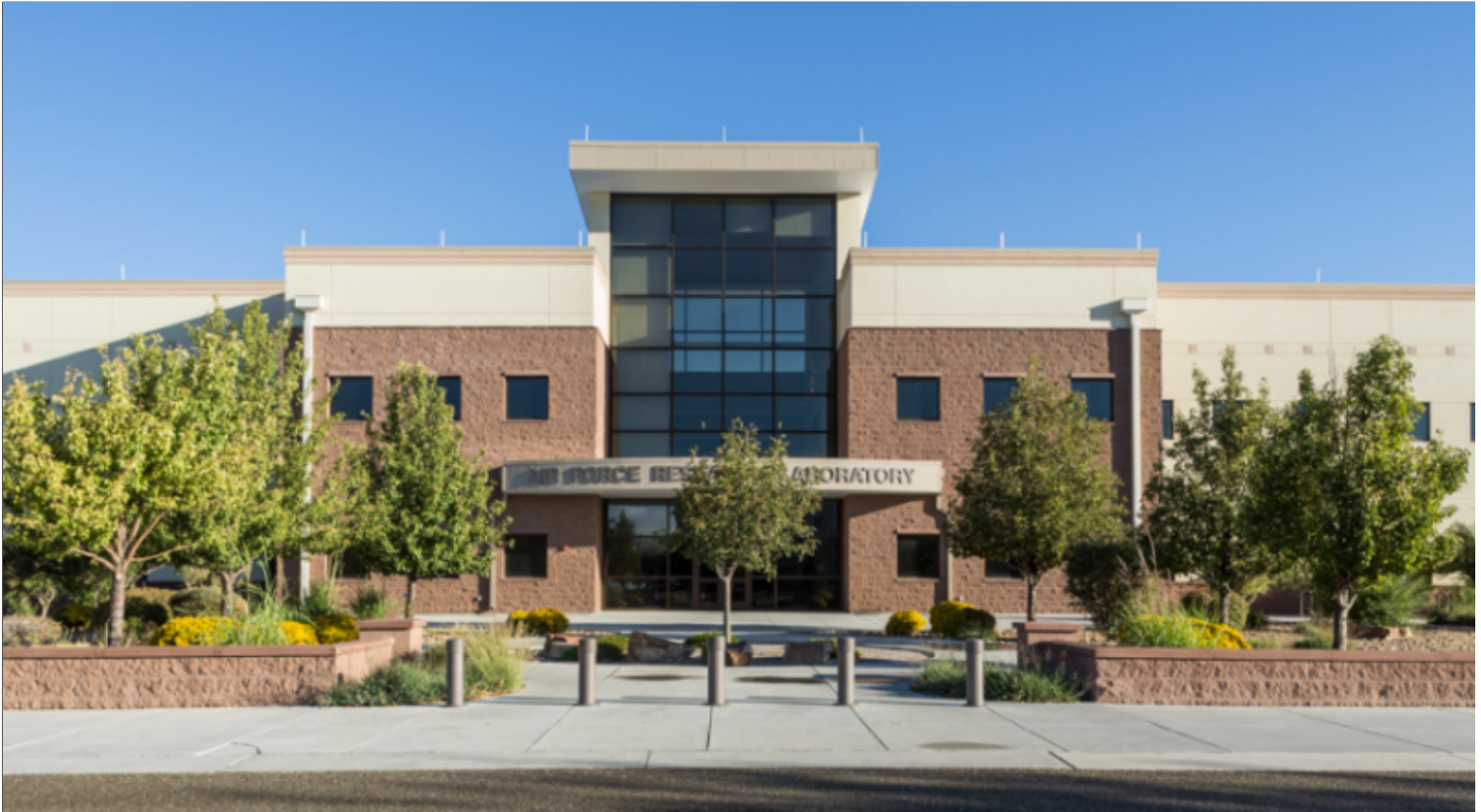
Entry Plaza Integrated with Facility Entry Facade Creating a Sense of Place and Visual Interest while Meeting AT Security Requirements
