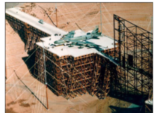
B52 on Trestle Project ca. 1980
