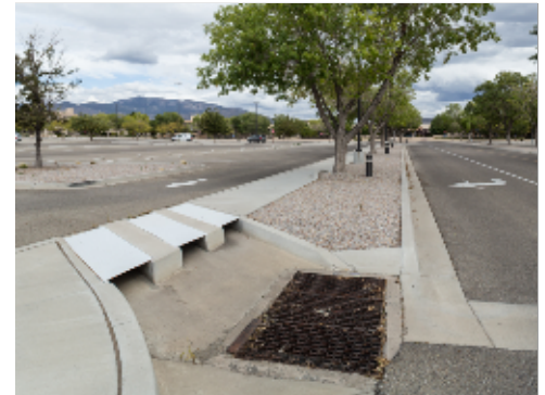
Flow Accommodation under Sidewalk
