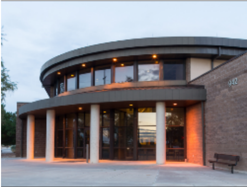
Building 942 Soffit Lighting at Entry
