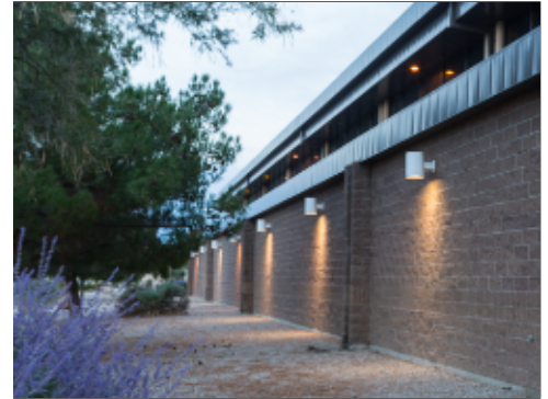
Building 942 Soffit and Sconce Lighting
