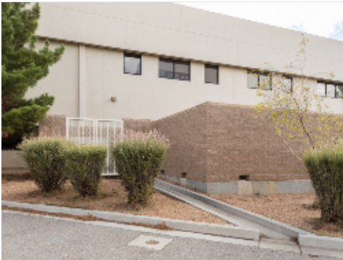
Drain to Curb from Scupper
