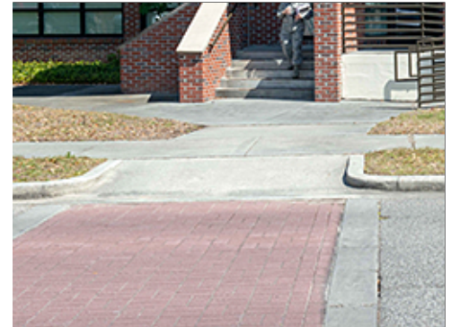
Colored Concrete Paving at Crosswalk
