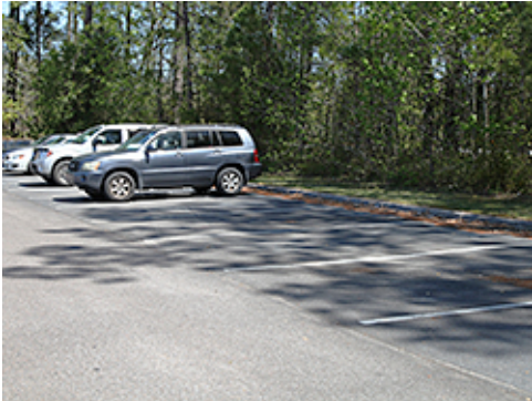
Standard Asphalt Paving and White Striping
