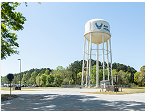
Coordinated Equipment Placement
