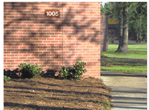
Pine Straw Mulch at Foundation Planting
