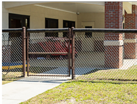
Chain Link Fencing
