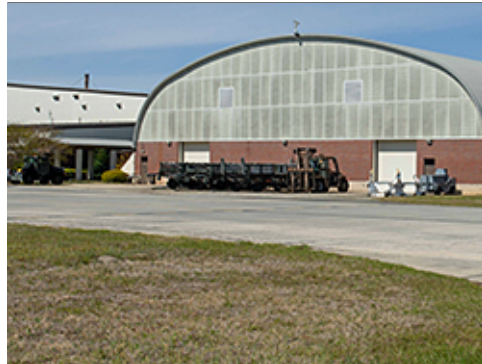
Functionally Required Concrete Paving
