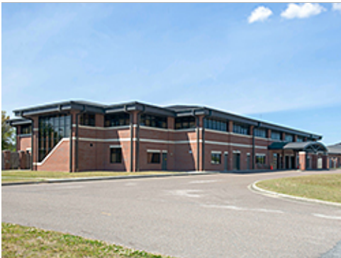
Group 2 Architectural Features
