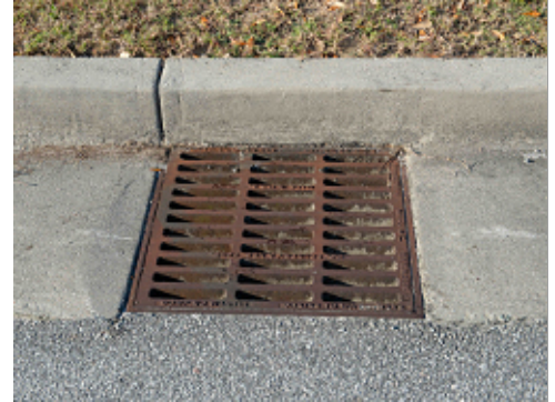
Stormwater Inlet at Curb and Gutter
