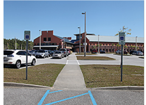
Blue Striping at Accessible Parking
