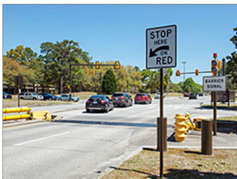
Integrated Security Elements
