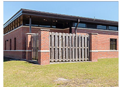
Utility Screen Walls
