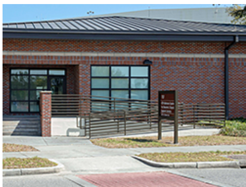
Integrated Ramp at Entrance
