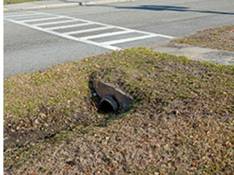
Pipe Culvert at Sidewalk
