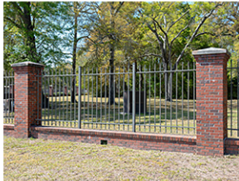
Brick and Metal Fence at Group 1
