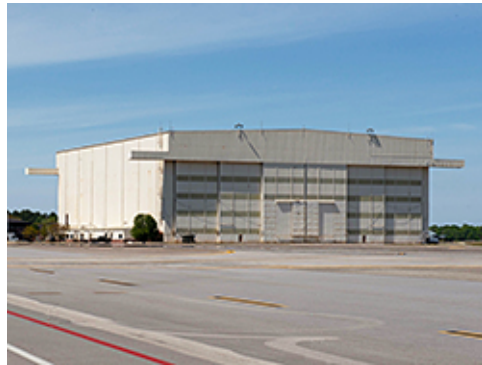
Group 3 Industrial Facility
