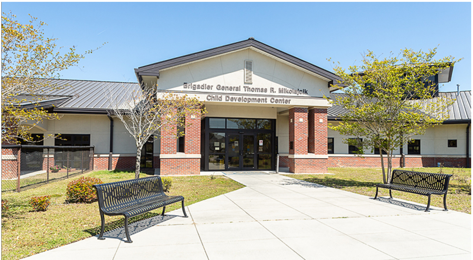
Concrete Entrance Plaza at Group 2
