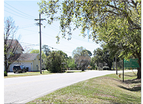
Overhead Electric Service
