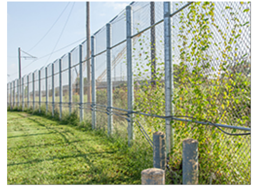
Fencing with Integrated Security Measures
