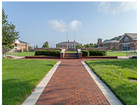
Brick Paving with Concrete Edging
