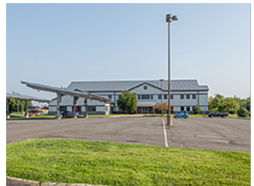
Parking Lot Lighting
