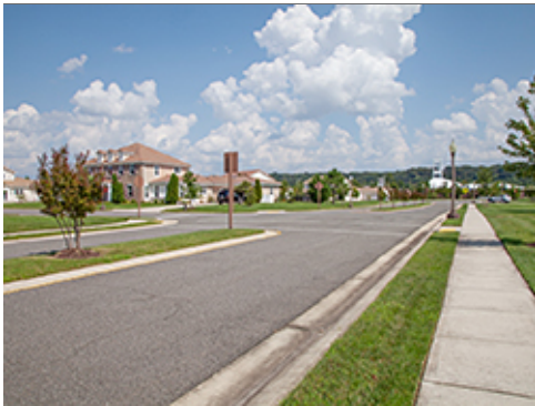
Detached Sidewalk at Group 4
