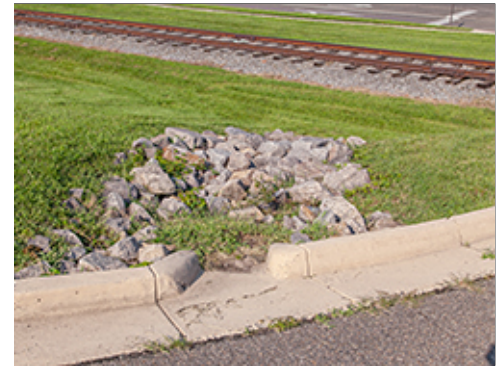
Rip Rap at Curb
