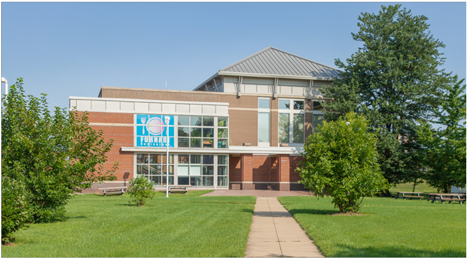
Contemporary Vernacular Architectural Features and Details
