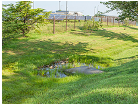
Inlet Located in Swale
