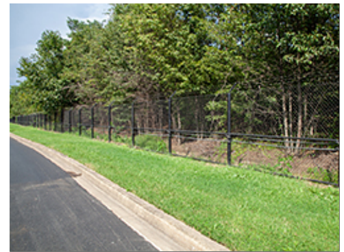
Grass Buffer at Perimeter Fence
