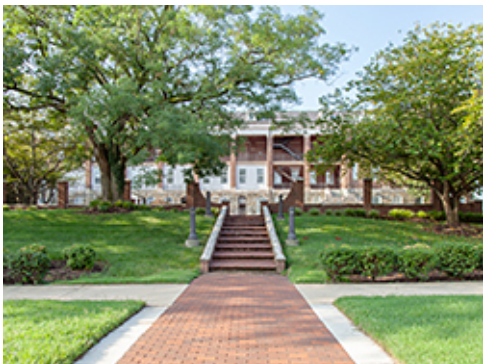
Brick Site Stair near Group 1
