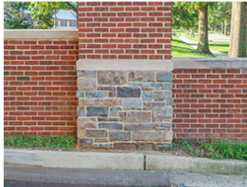
Coursed Ashlar Column Base
