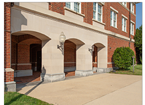
Concrete Entrance Plaza at Group 1
