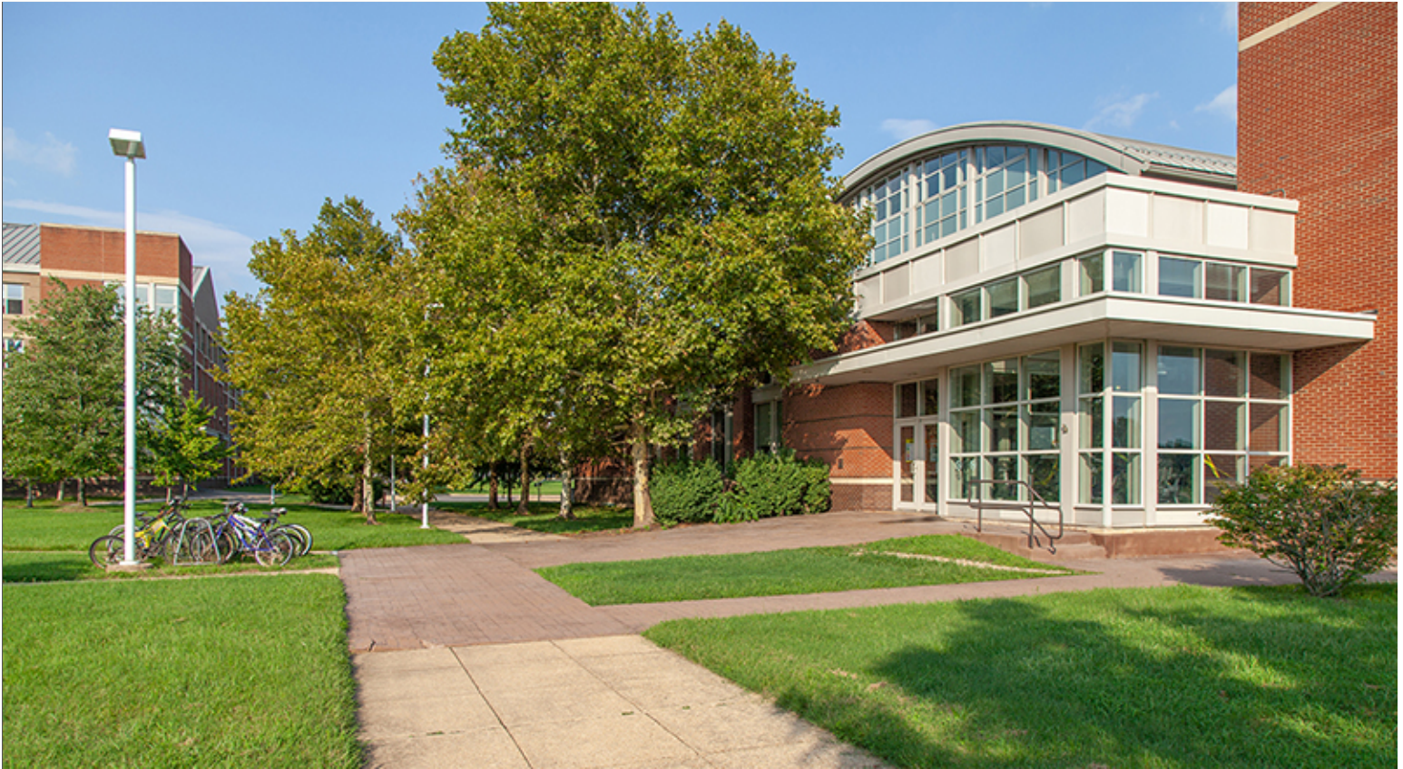
Predominant Use of Red Brick Blend with Brown Brick Accents and Neutral Metal Panels
