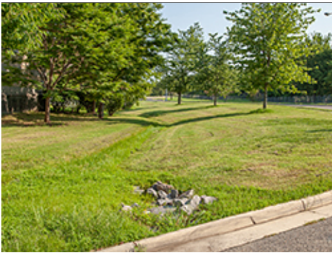
Grass Swale to Inlet
