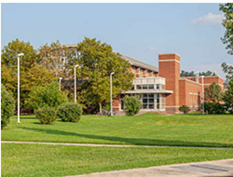
Pedestrian Scaled Lighting
