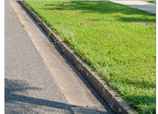
Standard Integral Curb and Gutter
