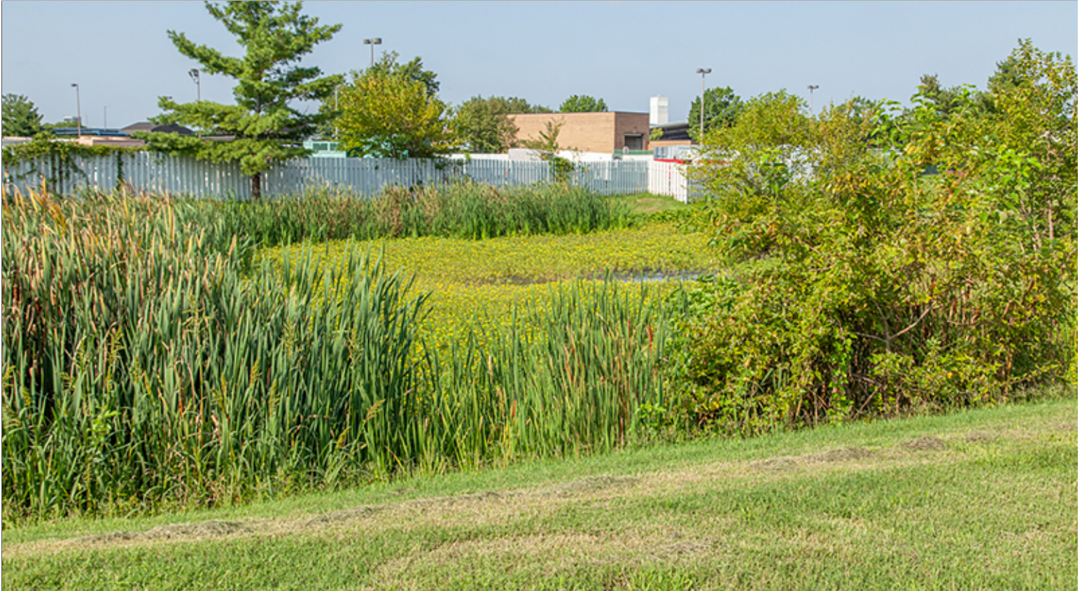
Stormwater Detention Area with Riparian Landscape
