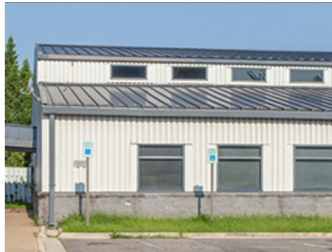
Clerestory Lighting at Group 3
