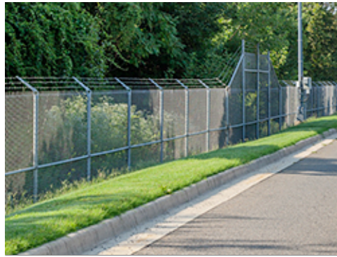
Chain Link Fencing near Group 3
