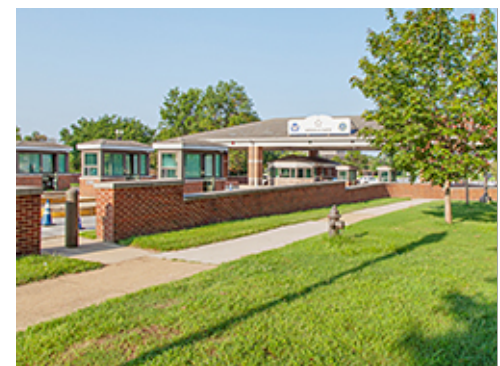
Fire Hydrant with Coordinated Access
