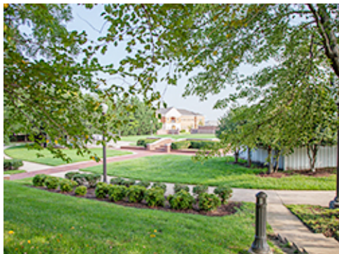
Concrete Site Stair
