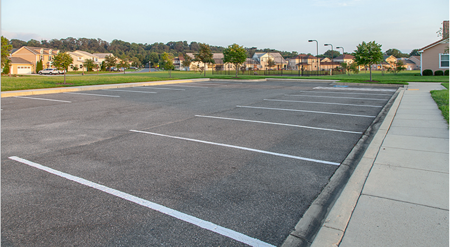
Bituminous Paving with Standard White Striping
