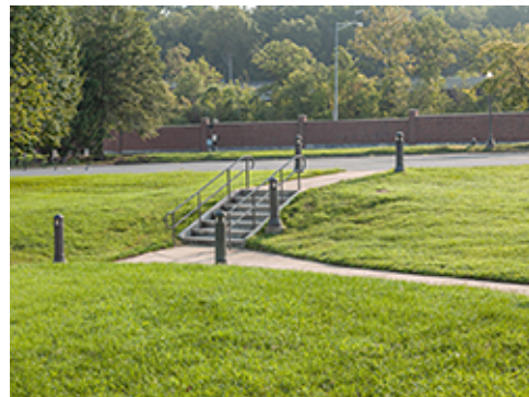
Site Stair with Railings
