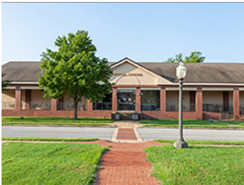
Brick Paving at Group 2
