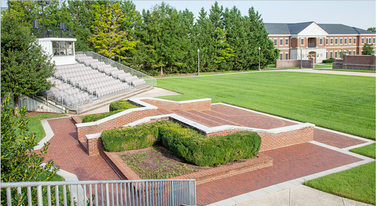
Brick Paving with Concrete Edging at Group 1
