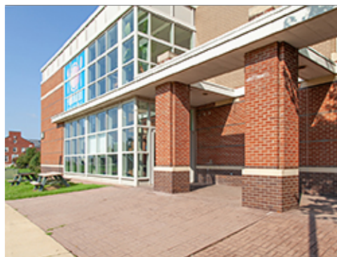
Stamped Colored Concrete at Group 2
