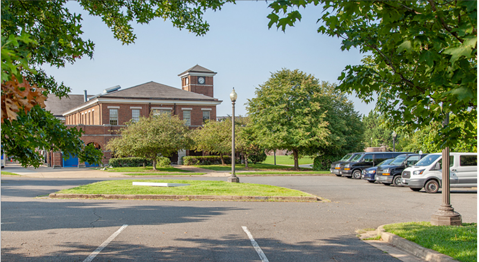
Building with Contiguous Parking Area and Connection to Secondary Entrance
