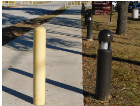
Group 2 Sidewalk Lighting
