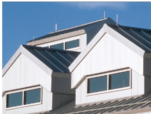
Coordinated Lightning Protection
