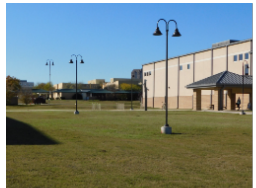
Open Space Lighting
