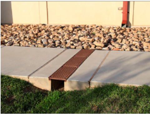
Directed Roof Drainage
