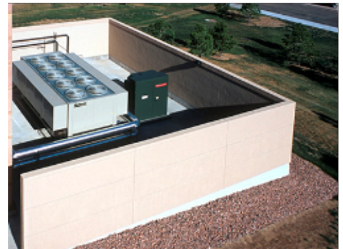
Screened Utility Yard
