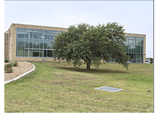
Storm Drainage Inlet
