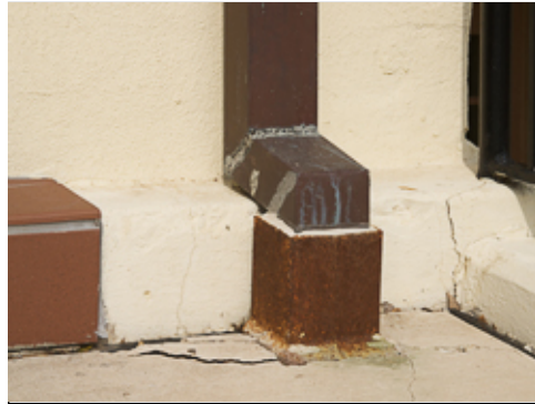
Roof Drainage Outlet
