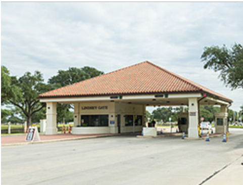
Stucco Wall Systems and Tile Roof
