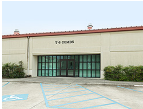
Clearly Defined Pedestrian Access
