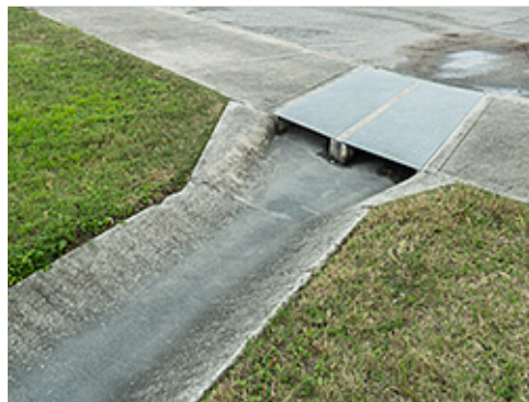
Trench Drain and Cover
