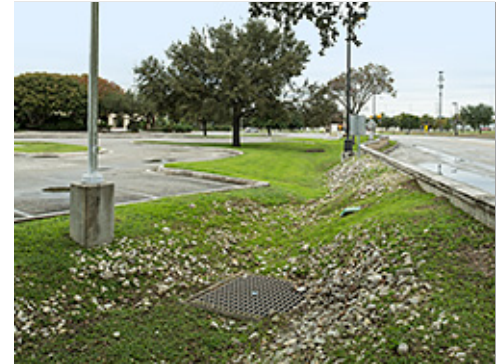
Storm Drainage Inlet
