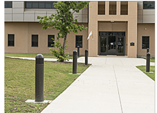
Functionally Required Lighted Bollards
