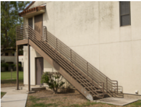
Second Story Access
