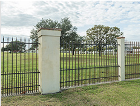
Masonry Piers with Stucco
