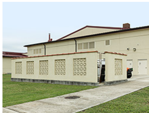
Walled Utility Yard
