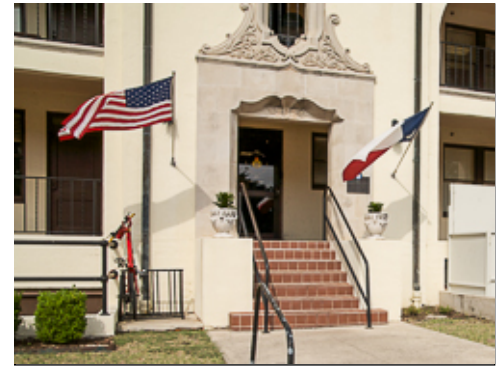
Entrance Stairs with Handrails
