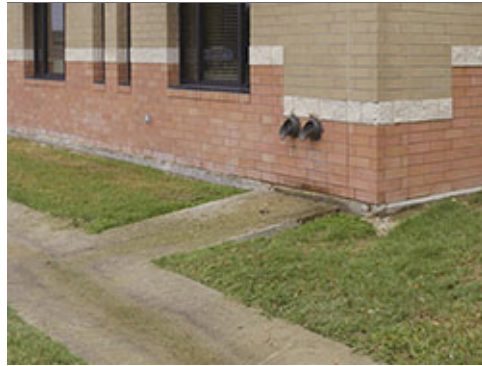
Roof Drainage Outlet
