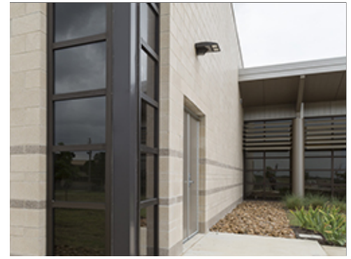
Secondary Entrance Lighting
