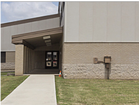
Equipment Matching Wall Color
