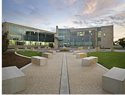
Decorative Paving at Facility Group 1
