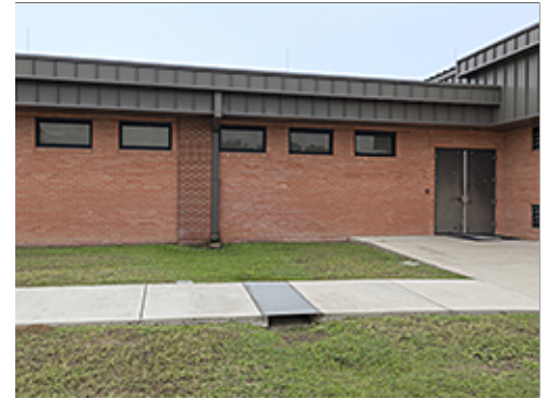
Trench Drain and Cover
