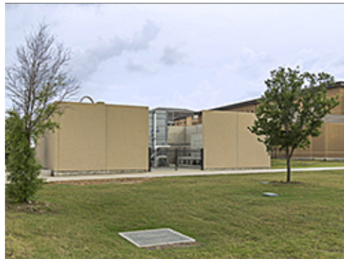
Screened Utility Yard
