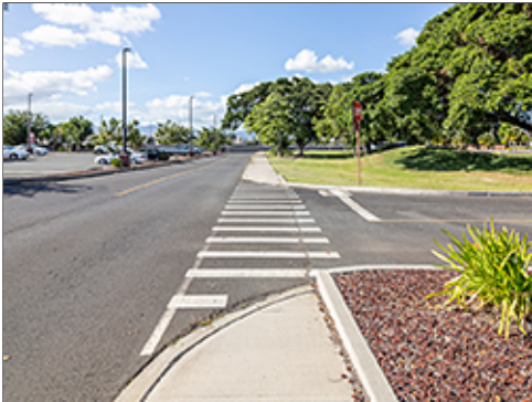
Curb Ramp and Crosswalks
