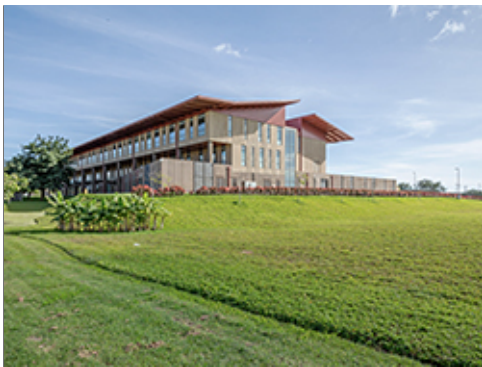
Maintained Grass Area
