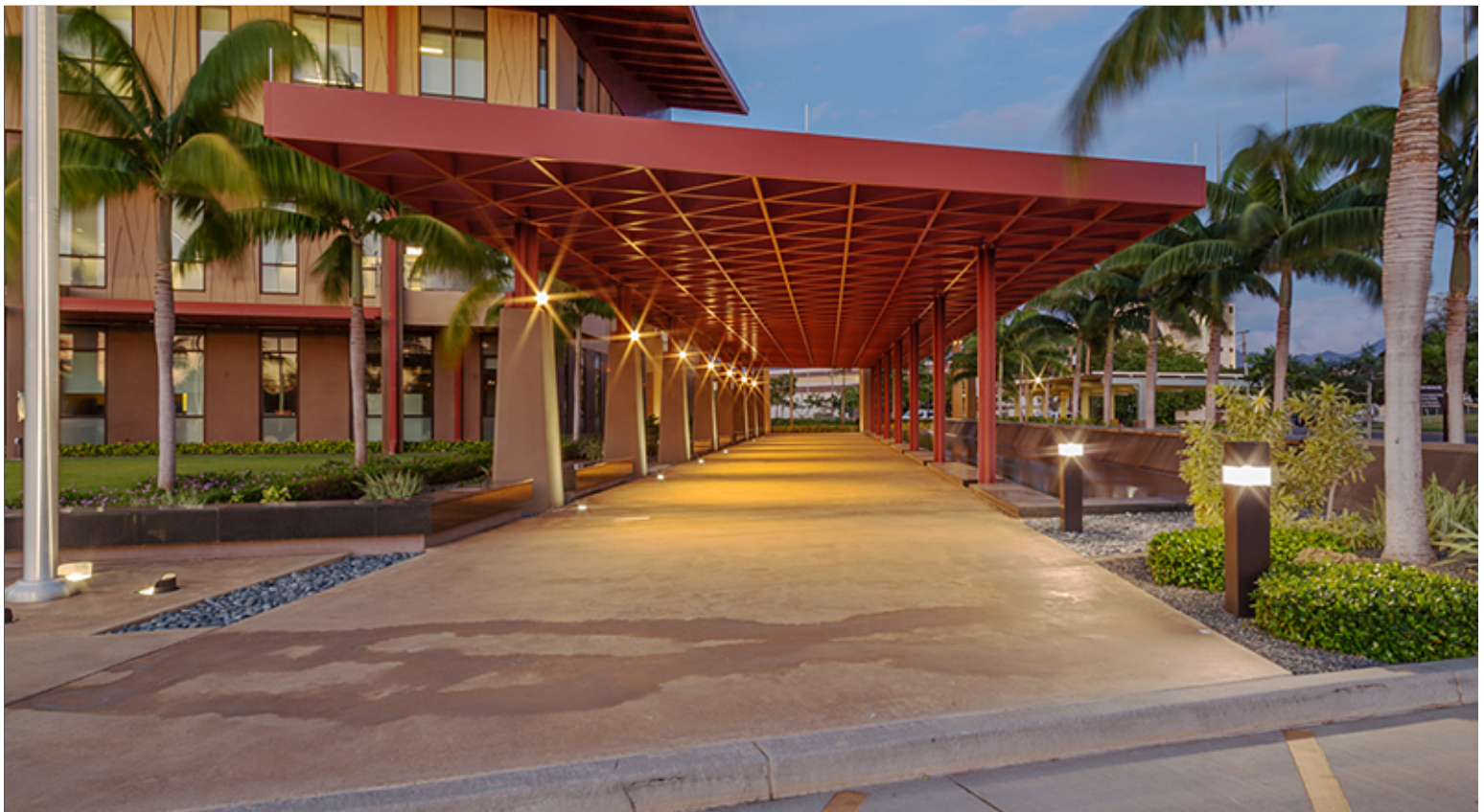
Wall Mounted Fixtures with Lighted Bollards
