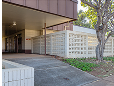
Ramp at Secondary Entrance
