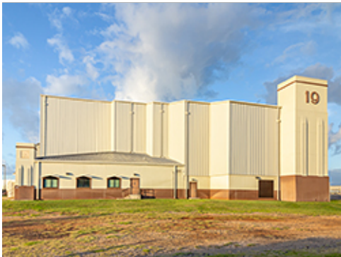
Group 3 Three-Bay Hangar
