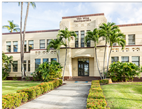
Facility Exteriors Group 1
