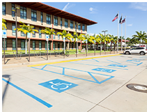
Alignment with Aisle at Accessible Spaces
