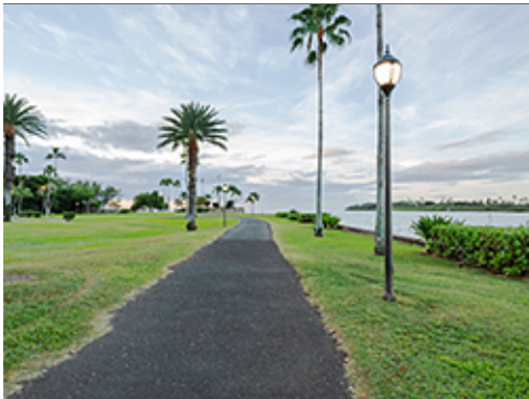
Pole Mounted Fixture along Walkway
