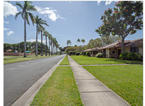
Detached Sidewalk at Group 4
