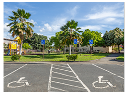
Alignment with Aisle at Accessible Spaces
