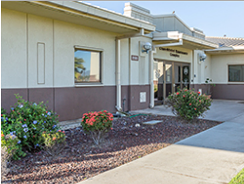
Roof Drainage Directed through Planting Bed
