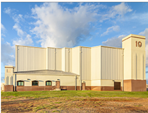
Facility Exteriors Group 3
