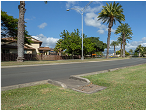
Street Run Off
