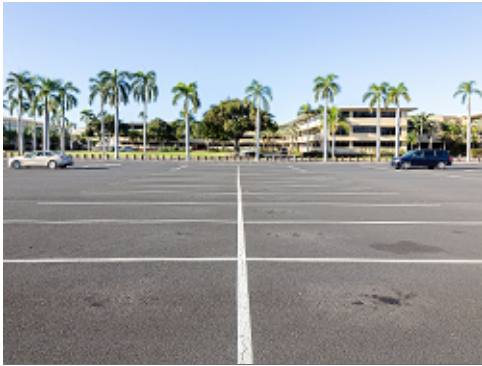
Asphaltic Concrete with White Striping
