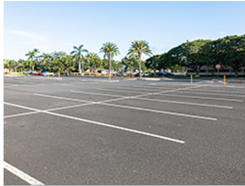
Asphaltic Concrete with White Striping
