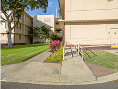
Ramp and Sidewalk at Secondary Entrance
