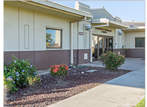
Roof Drainage Directed through Planting Bed
