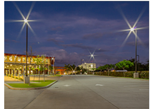
Parking Lot Lighting at Group 2
