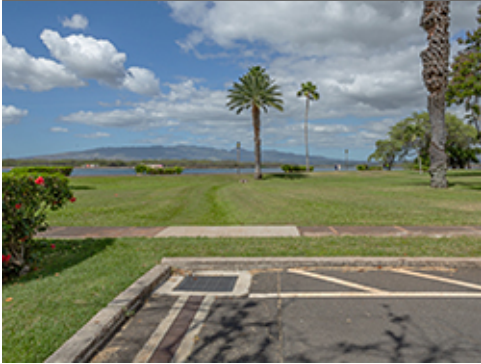
Storm Drain Inlet
