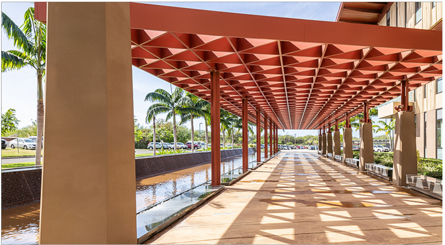
Colored Concrete Paving at Plaza with Shading Canopy
