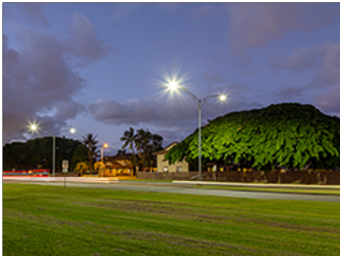
Street Lighting at Intersection
