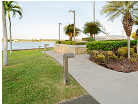
Lighted Bollards and Pole Mounted Fixtures
