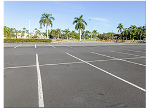
Asphaltic Concrete with White Striping
