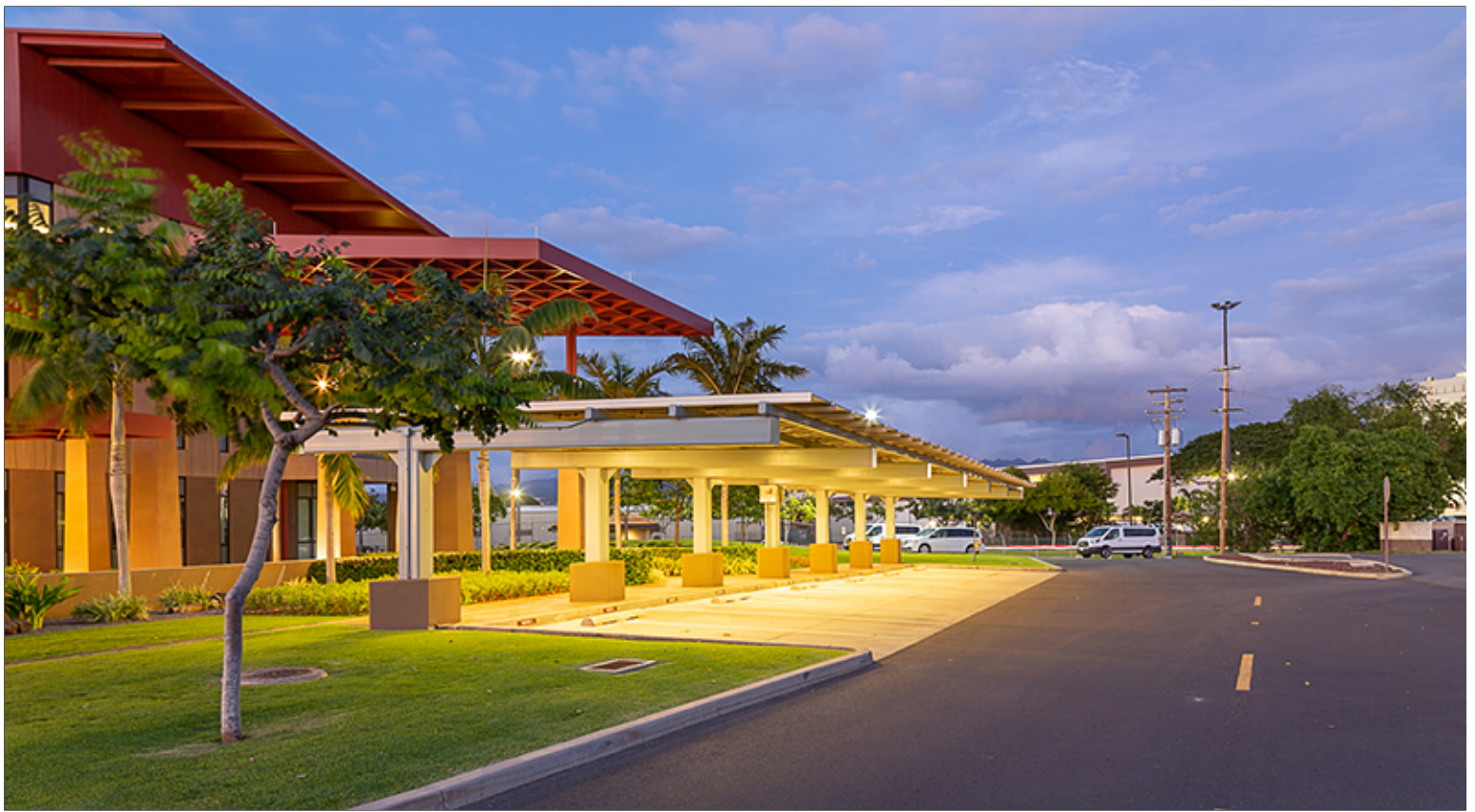
Consolidated Sidewalk Lighting and Parking Lighting
