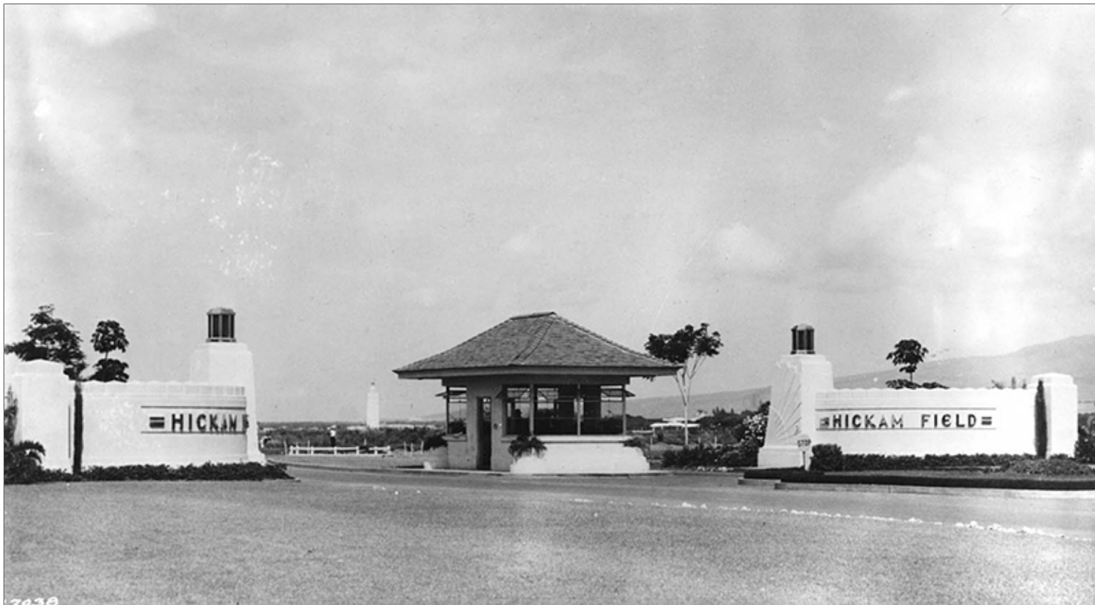
Main Gate at Hickam Field
