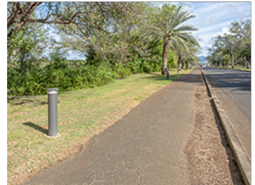
Lighted Bollards Defining Sidewalk
