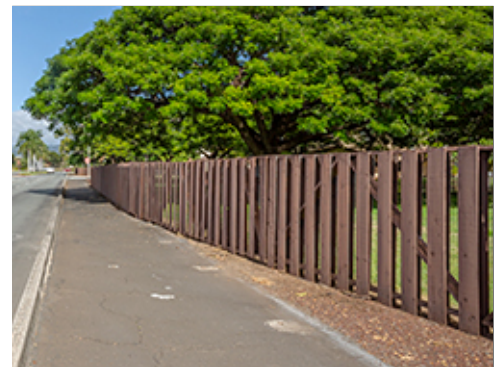
Perimeter Fencing along Group 4
