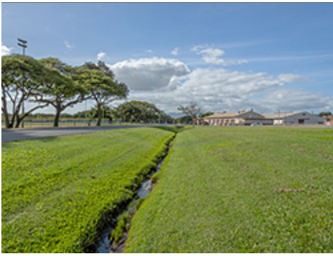
Landscaped Stormwater Swale
