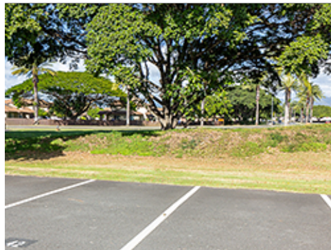
Groundcover at Slope
