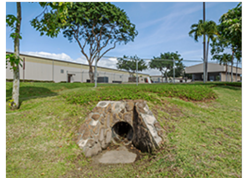
Stormwater Pipe at Street
