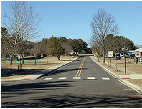
Collector Street in Facility Group 4
