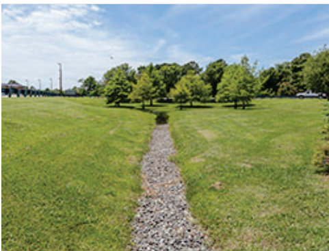
Stabilized Drainage Surface
