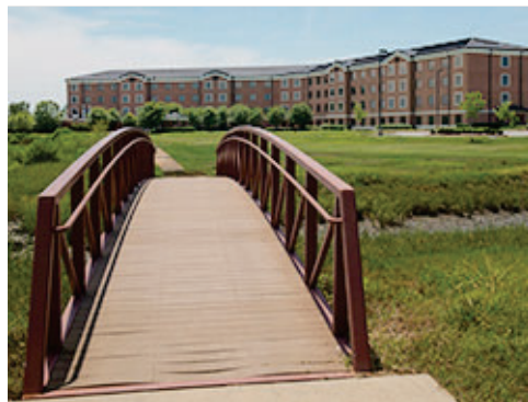
Bridge as an Amenity
