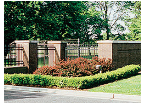
Brick Piers and Metal Fencing
