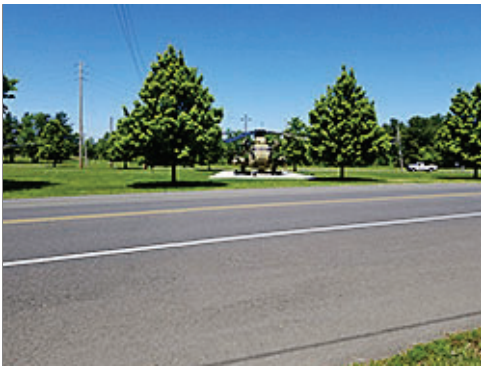
Typical Asphaltic Concrete Paving
