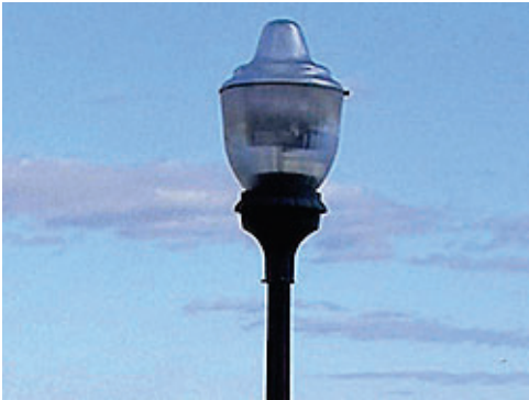
Street Light Pole and Fixture
