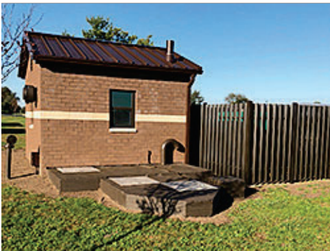
Compatible Sewage Lift Station
