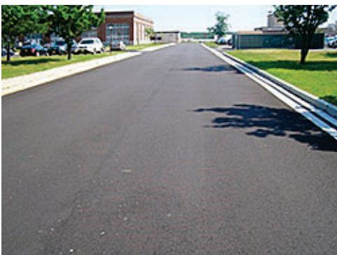
Asphaltic Concrete Paving
