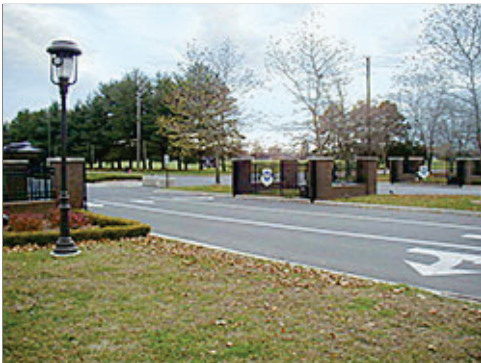
Perimeter Fence at Gate
