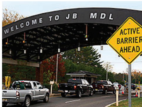
Main Gate and Canopy
