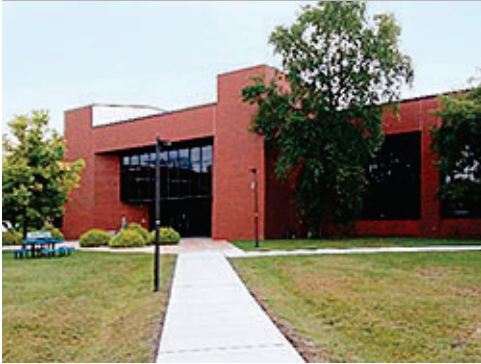
Group 2 Sidewalk with Concrete Paving
