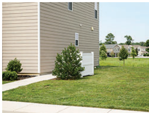
Screening at Utilities
