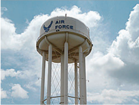
Elevated Water Storage
