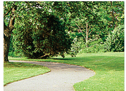
Asphaltic Concrete Trail Paving
