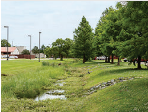
Drainage Area with Grasses
