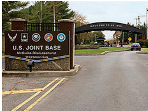
Integrated Fencing at Gate
