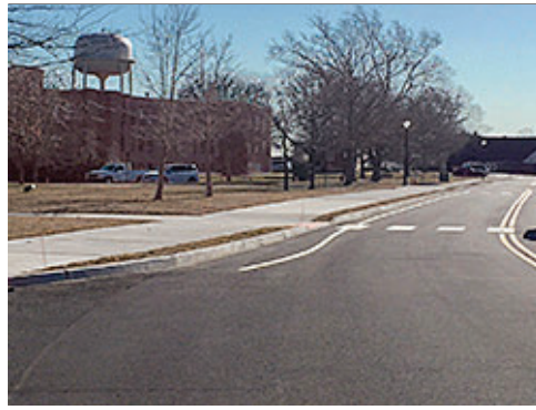
Collector Adjacent to Facility Group 2
