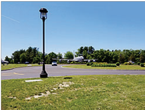
Standard Street Light Fixture
