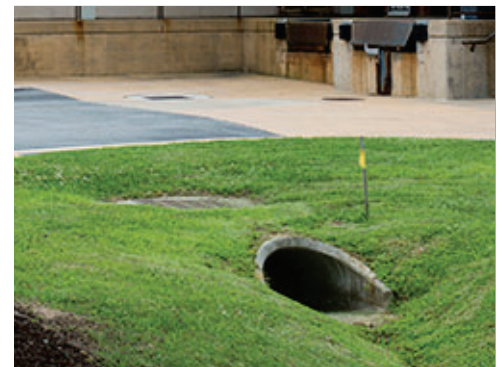
Storm Inlet and Culvert
