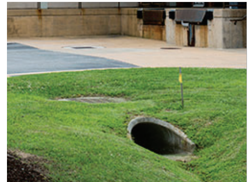
Storm Inlet and Culvert
