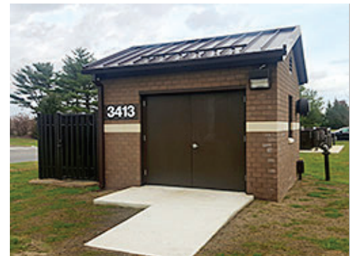
Compatible Utility Structure
