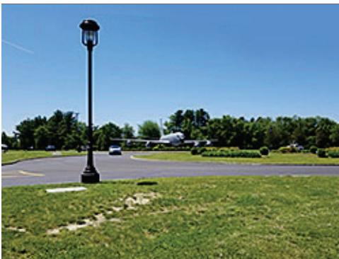
Street Light Pole and Fixture
