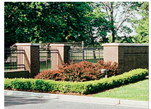
Brick Piers and Metal Fencing
