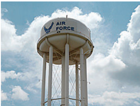
Elevated Water Storage
