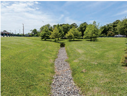
Stabilized Drainage Surface
