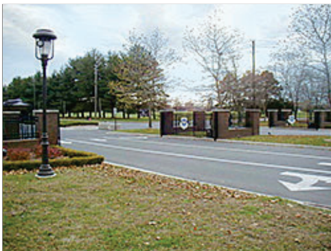
Perimeter Fence at Gate
