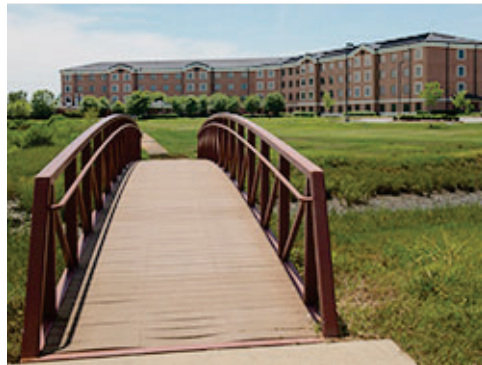
Bridge as an Amenity
