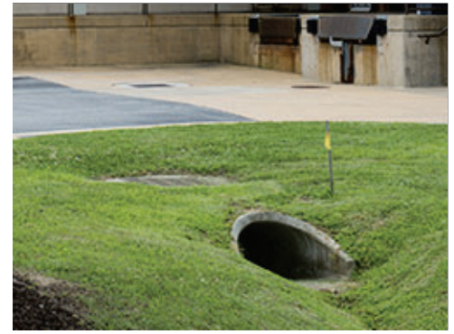
Storm Inlet and Culvert
