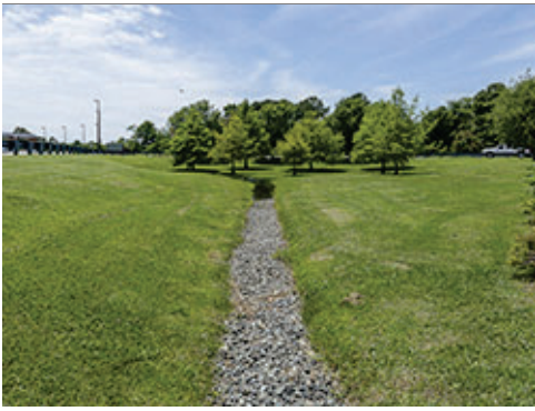
Stabilized Drainage Surface
