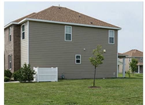
Residential Utilities Screening
