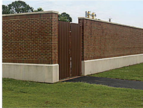
Screen Wall and Gate
