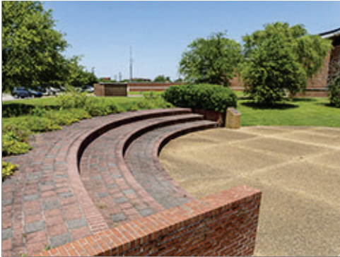
Brick and Concrete Paving
