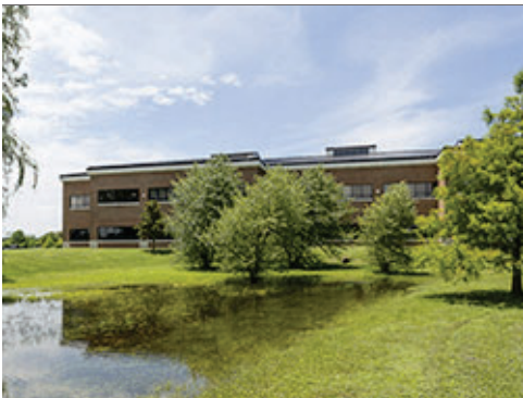
On-site Hydrologic Control
