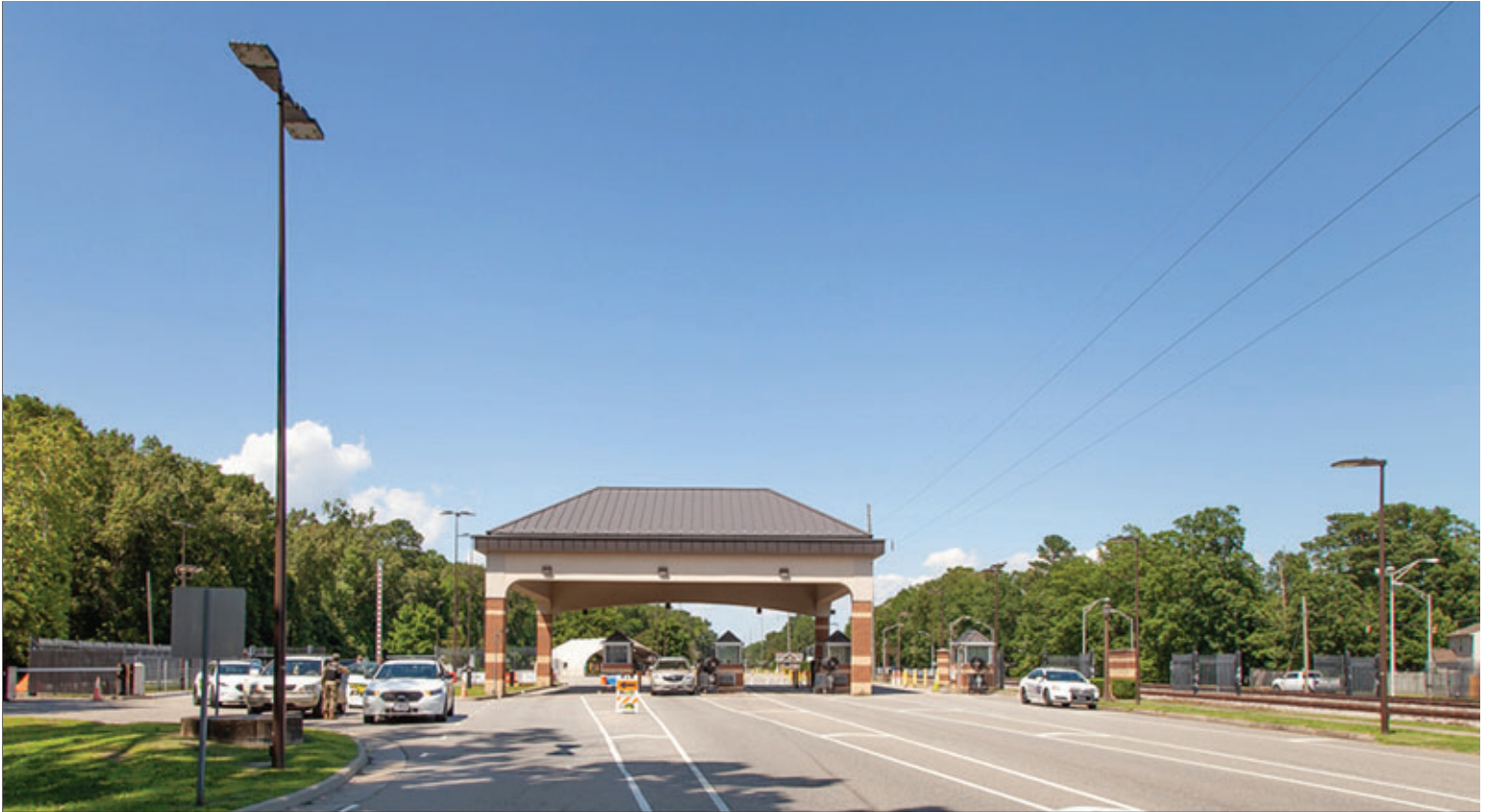
High Efficiency Downlighting at Main Gate
