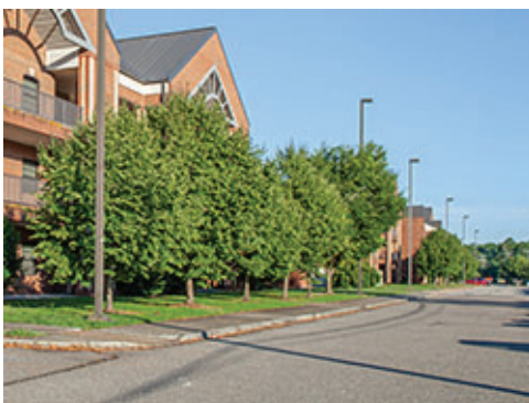
Buried Utilities at Group 2
