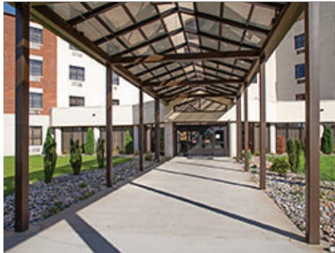
Concrete Paving at Covered Entrance
