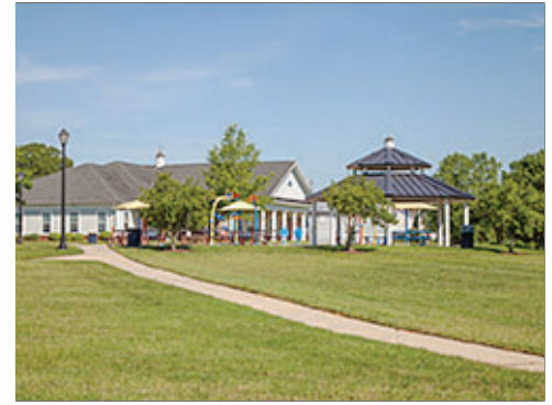
Playground and Pavilion
