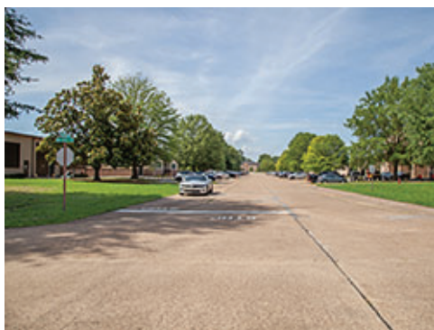
Intersection Adjacent to Group 3
