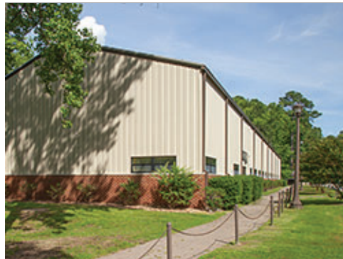
Metal Panels at Group 3
