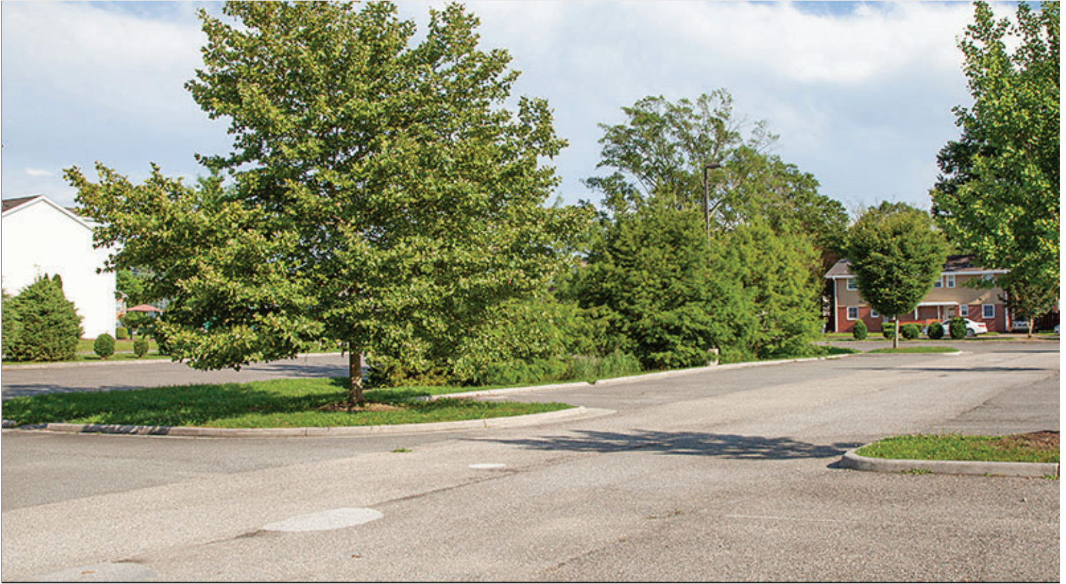
Parking Lot Graded to Drain to Central Bioswale
