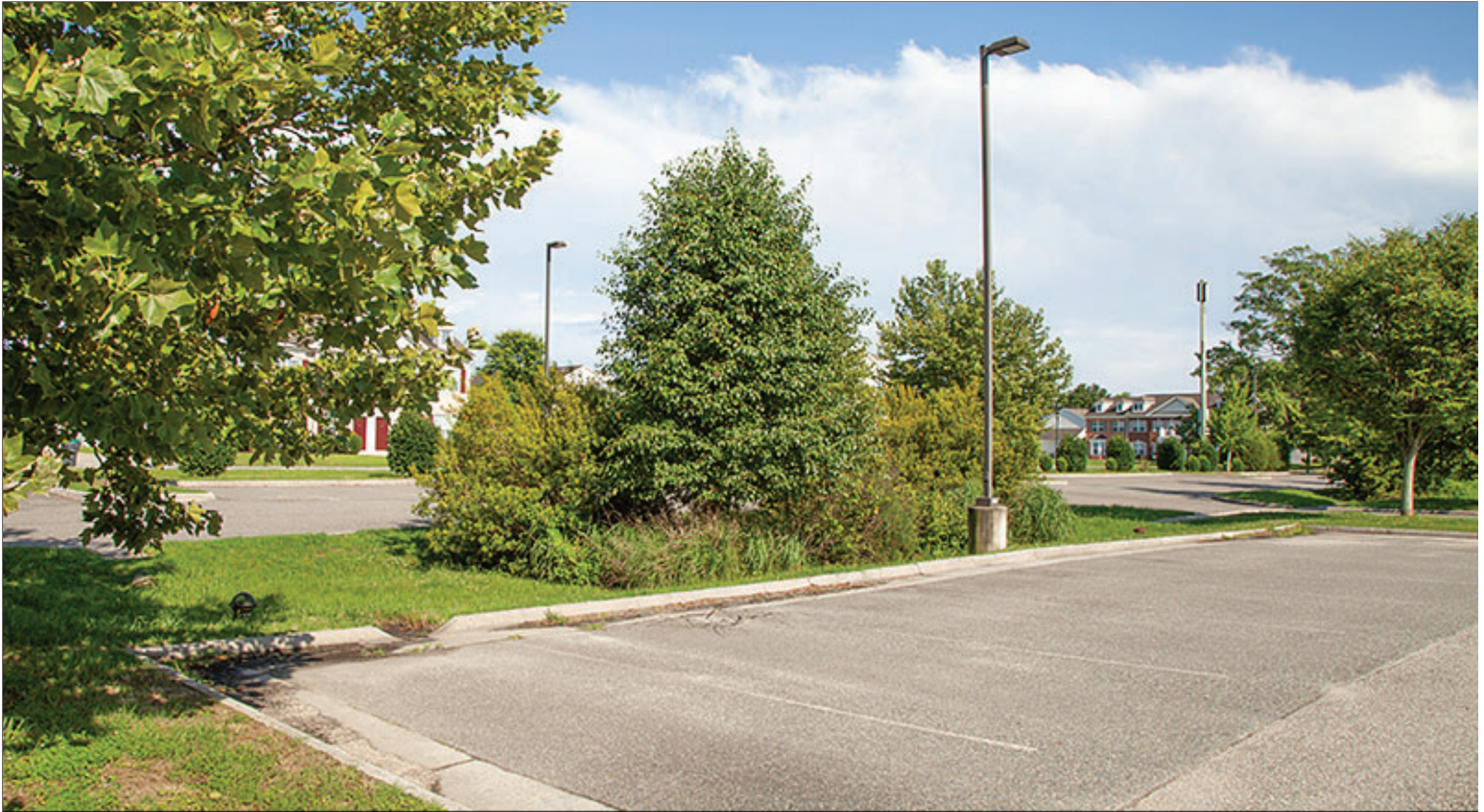
Bioswale Integrated with Median
