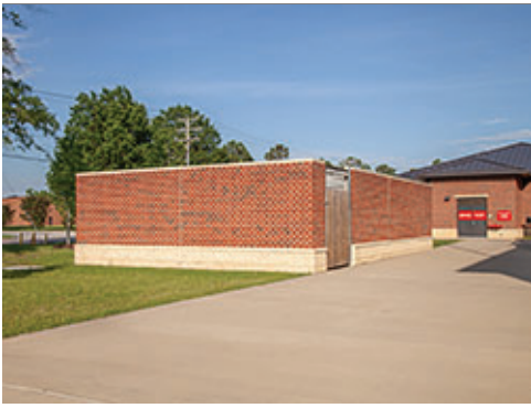
Underground Services to Mechanical Yard
