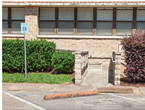
Ramp at Group 2
