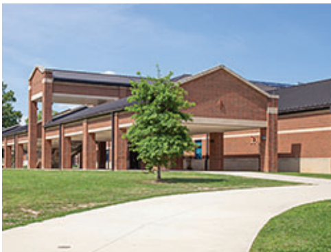
Grade Accommodating Slope
