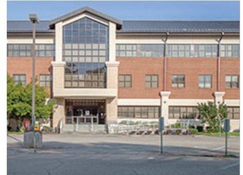
Designated Accessible Parking
