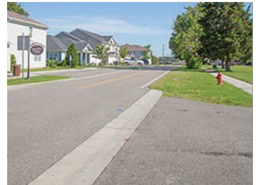
Integrated Concrete Drain Pan
