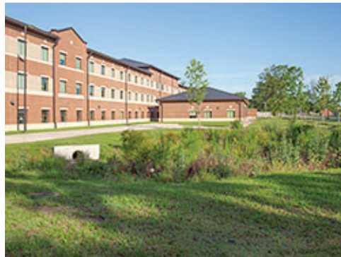
Roof Drainage to Bioswale
