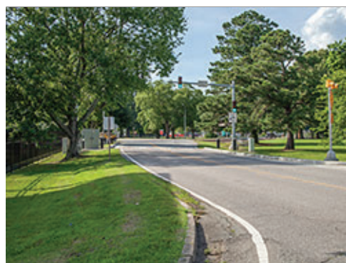
Barrier Signal along Special Route
