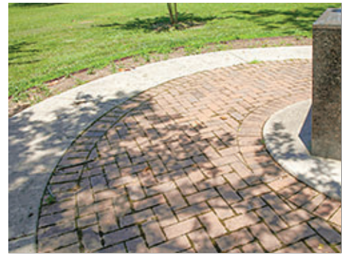
Brick Pavers and Concrete Edging
