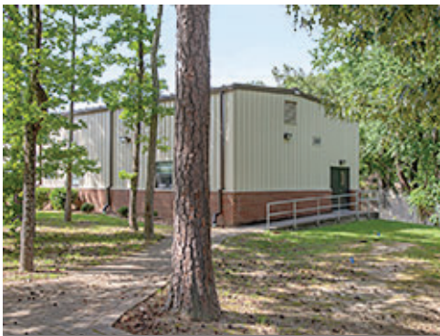
Ramp at Group 3
