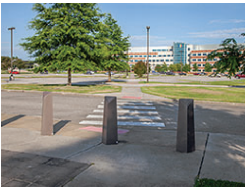
Central Sidewalk Linking Facilities
