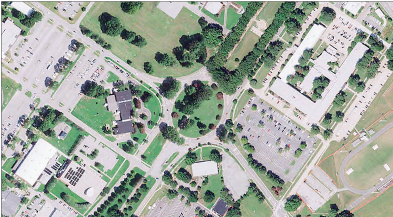
Major Intersection of Arterials with Traffic Circle and Green Space as a Focal Point
