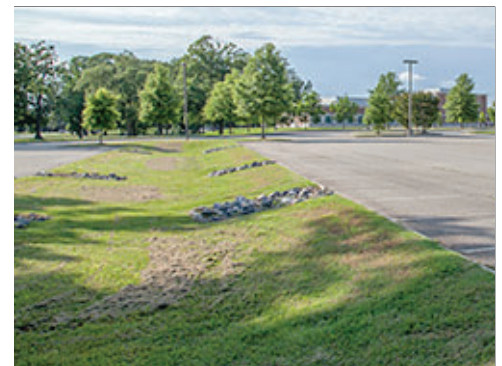
Median with Rip Rap for Stormwater
