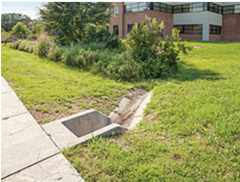
Parking Lot Drainage to Bioswale
