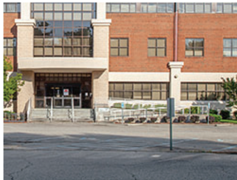
Stair and Ramp at Group 1
