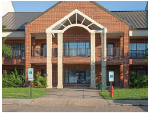
Concrete Entrance Plaza
