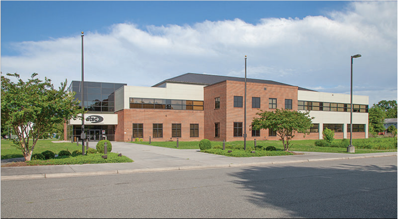
Group 2 Materials Palette: Predominant Use of Brick and Secondary Use of Metal Panel as an Accent
