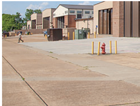
Functionally Required Concrete Paving
