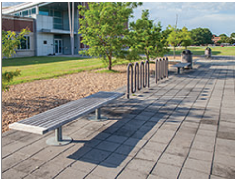
Concrete Pavers at Group 2
