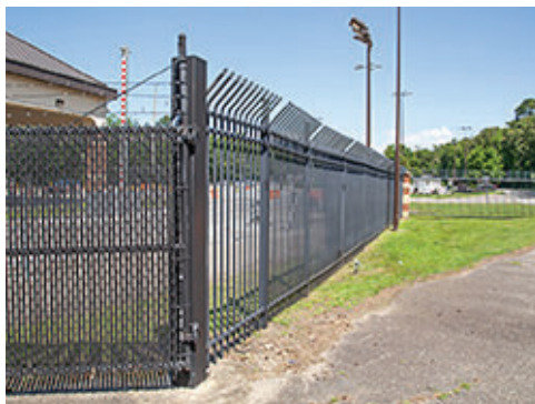
Metal Fence with Outriggers
