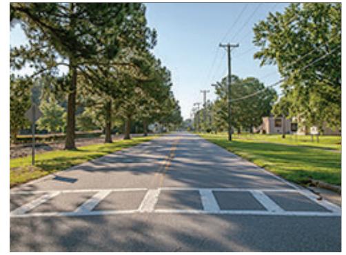
Overhead Electric Service Lines
