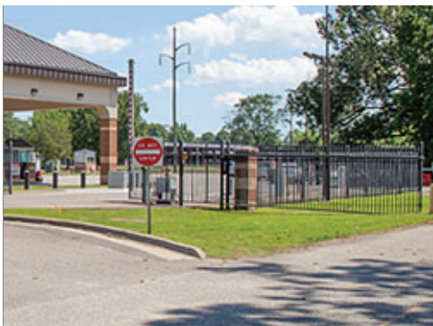
Masonry Piers and Metal Fence at Group 1
