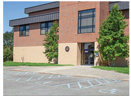
Curb Ramp at Accessible Parking
