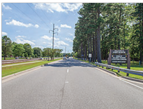
Divided Arterial near Main Gate
