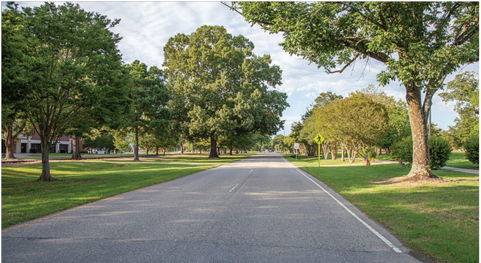
Washington Boulevard near Marshall Street: A Divided Arterial with an Expansive Landscaped Median
