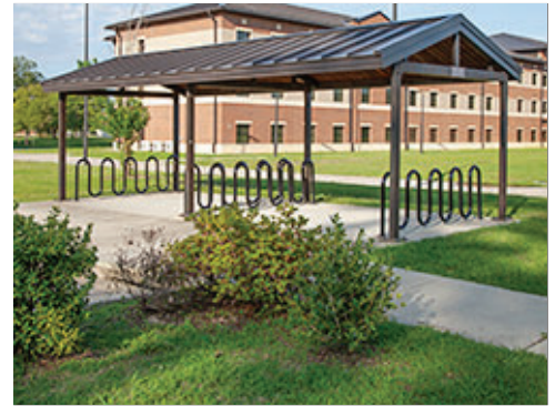
Concrete Paving at Pavilion
