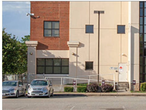
Parking Lot and Sidewalk lighting
