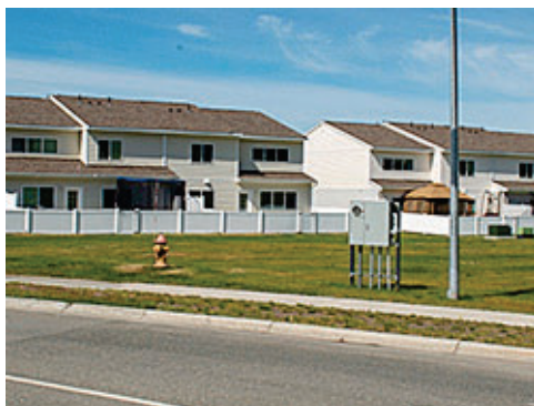
Fire Hydrant and Electrical Cabinet
