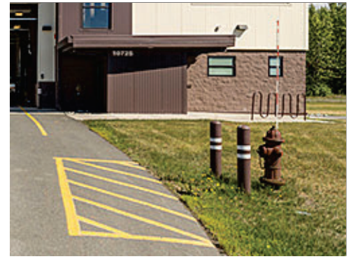
Fire Hydrant with Vertical Flag
