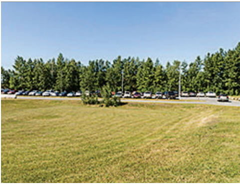
Large Detention Basin
