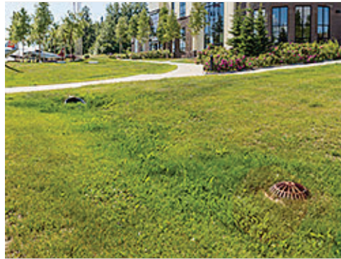
Culvert, Swale and Inlet
