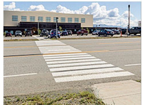
Base Standard Crosswalk Striping
