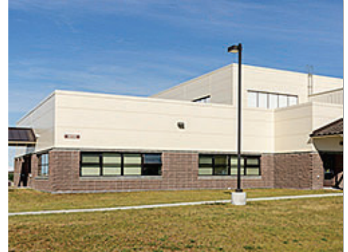
Group 3 Ground Mounted Fixtures
