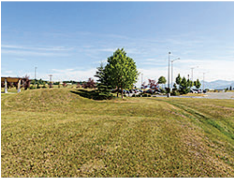
Berm and Swale to Direct Stormwater
