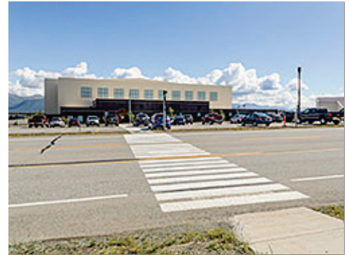
Base Standard Crosswalk Striping
