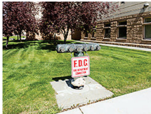
Standpipe Connection
