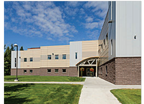
CMU and Insulated Metal Panels
