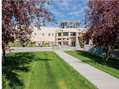
Connection to Main Entrance
