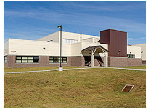
Stormwater Outlet to Detention Area
