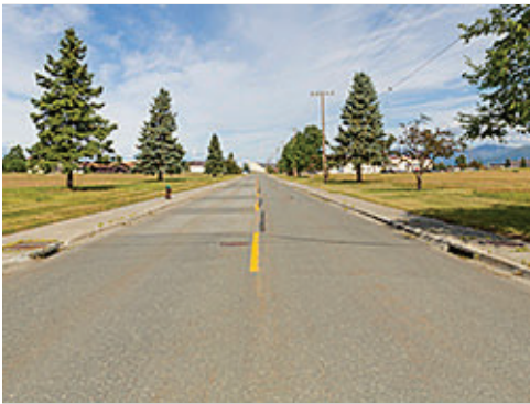
Storm Sewer Inlets at Gutter
