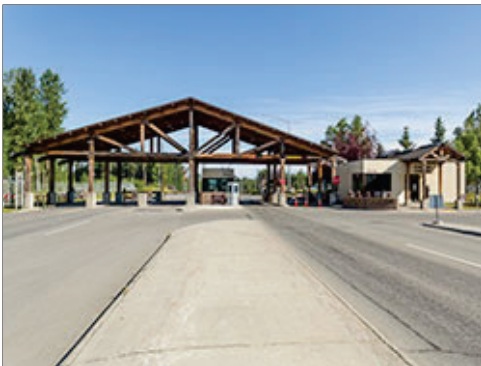
Divided Arterial at Gate
