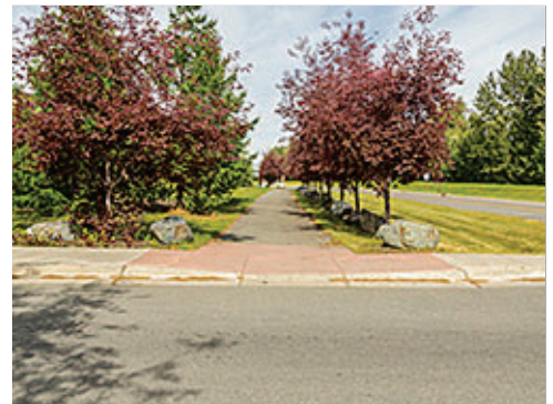
Asphalt Paving at Trail
