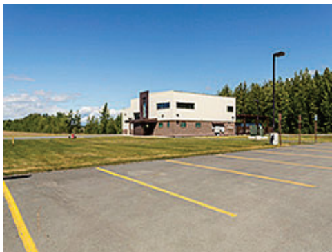
Standard 4-Inch Striping
