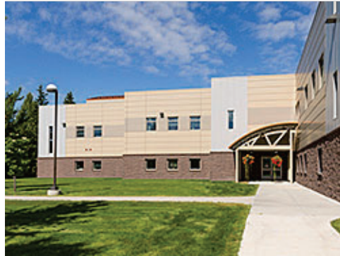
Ground-Mounted and Wall-Mounted Fixtures
