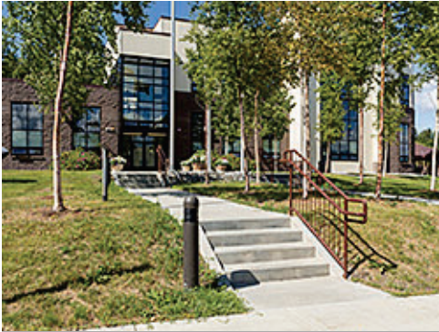
Site Stair and Railing
