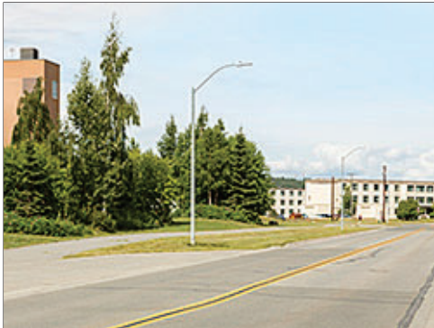
Base Standard Street Lighting
