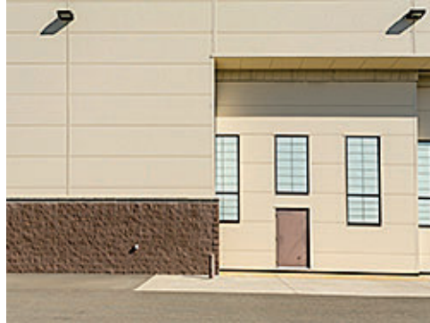
Group 3 Wall Mounted Fixtures
