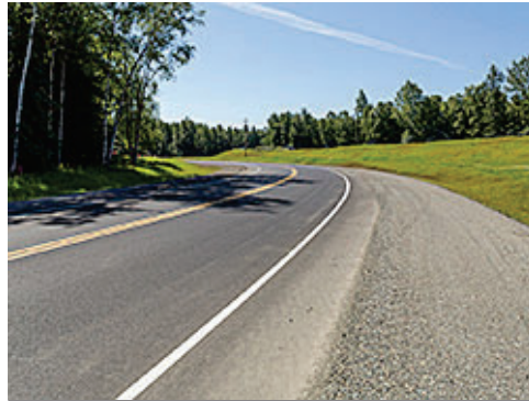
Rock Paving at Shoulder
