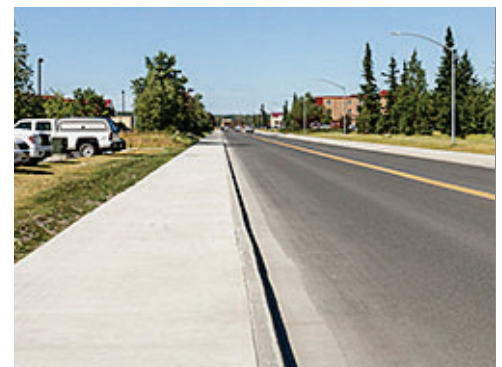
Barrier Curb with Attached Sidewalk
