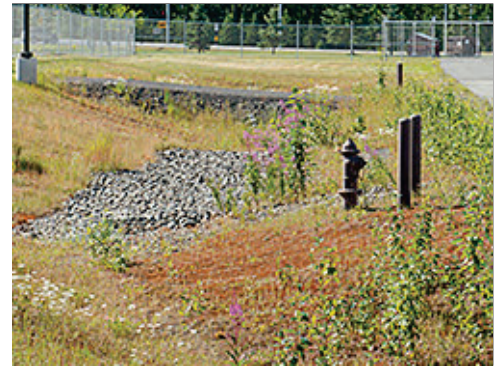
Rip Rap at Swale
