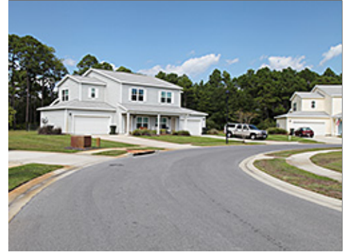
Asphaltic Paving in Group 4
