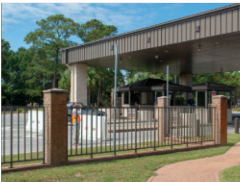
Fencing at Group 1 Facility
