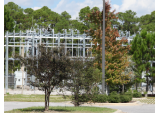
Landscape Screening at Utility Structure
