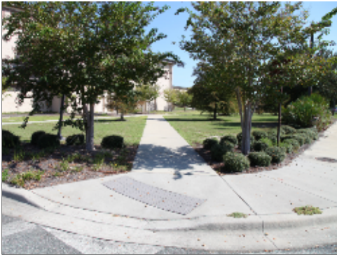
Accessible Curb Ramp
