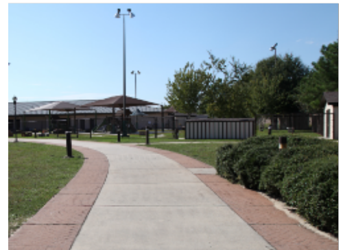
Concrete with Decorative Edging
