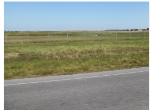
Paving on Remote Road without Curb
