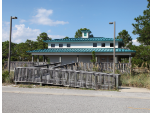
Lumber Framing at Recreational Area
