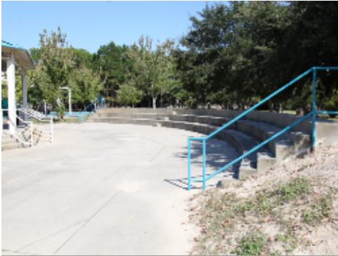
Site Stair with Pipe Railing
