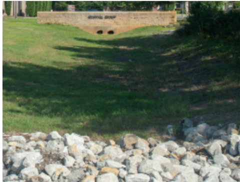
Swale with Rip-Rap
