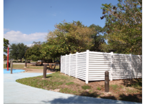
Screen Wall at Utility Elements
