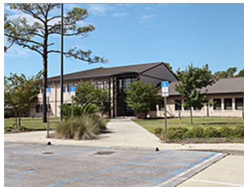
Adjacent Accessible Parking
