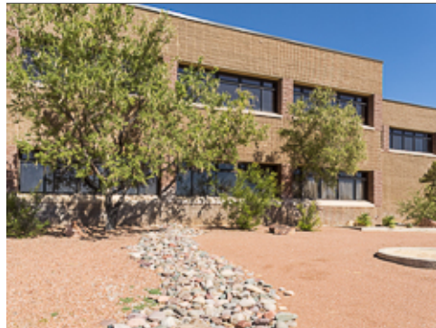
Landscaping surrounding WG HQ
