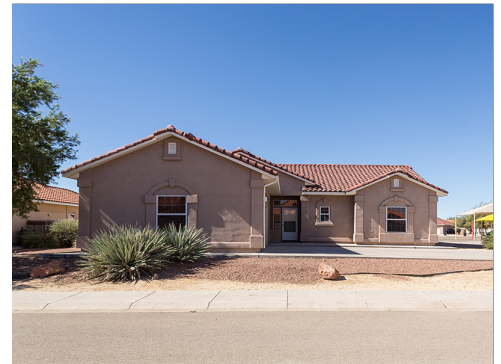
Group 4 Single Family Structure
