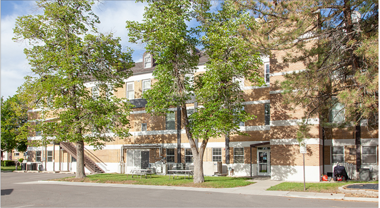
Trees Shading Facade
