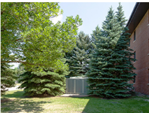
Visual Screening of Mechanical Equipment
