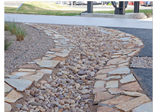
Stone Rip-Rap and River Rock Basin
