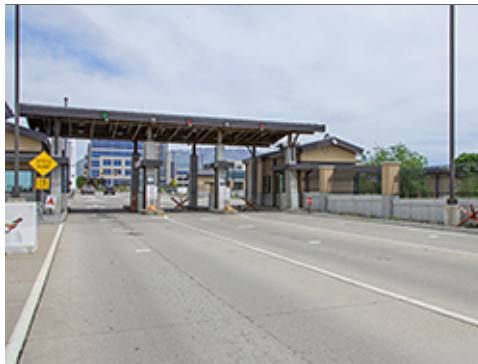
M Avenue Arterial at Gate
