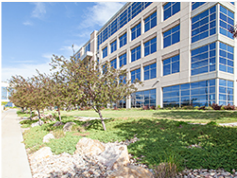
Site Sloped to Drain toward Planting Area
