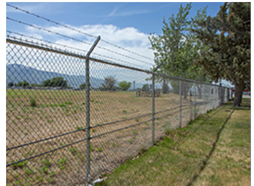
Chain Link with Outriggers at Group 3
