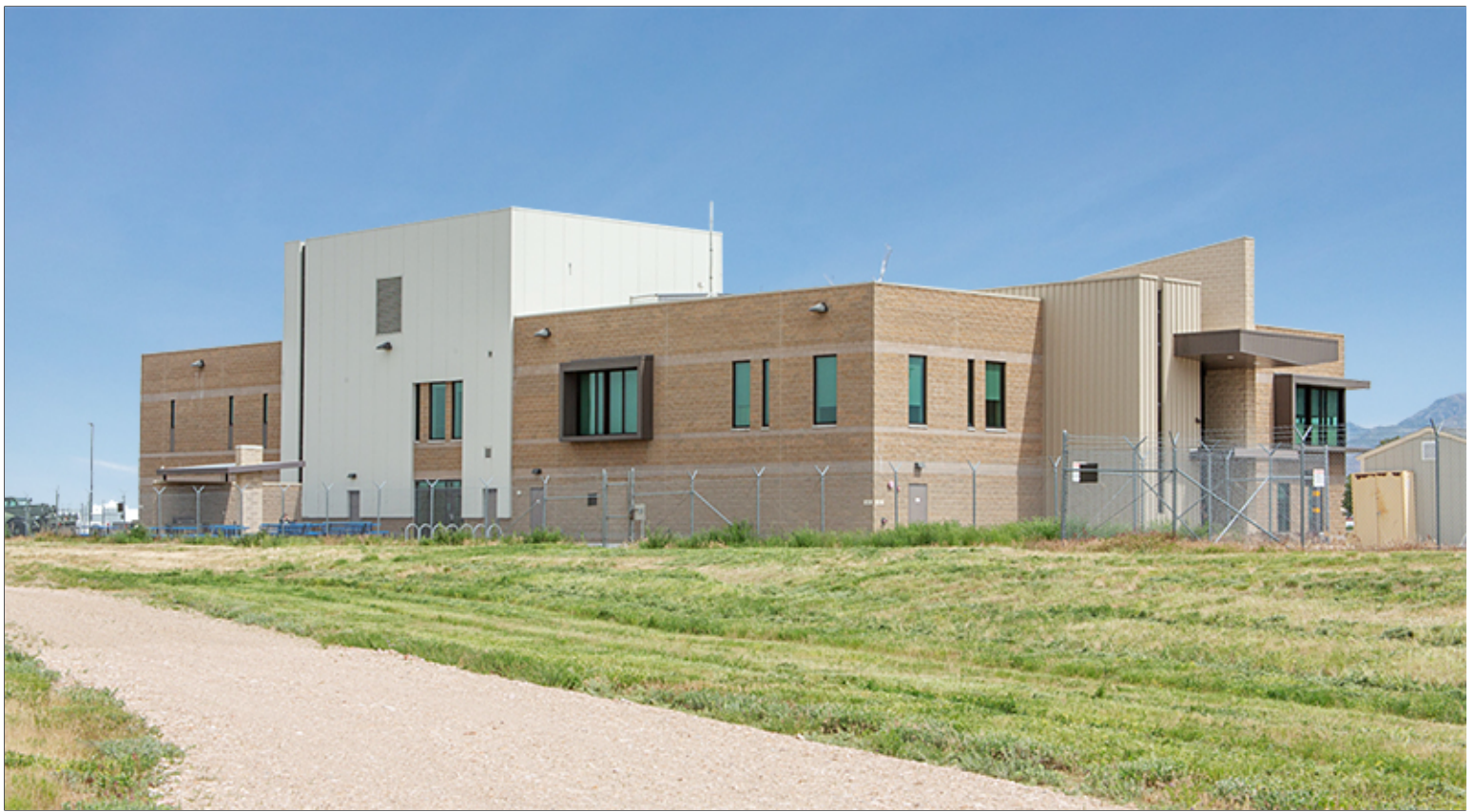
Example of Contemporary Architectural Theme with Functional Shading
