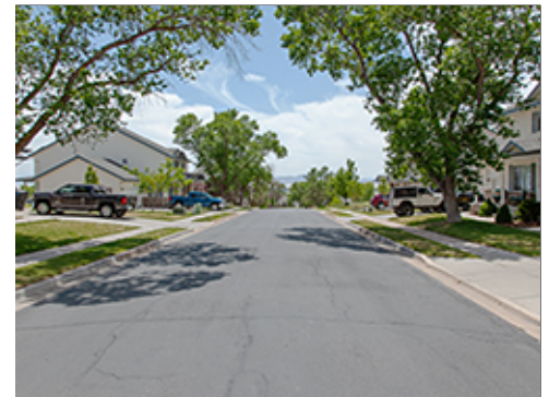
Local Street at Group 4
