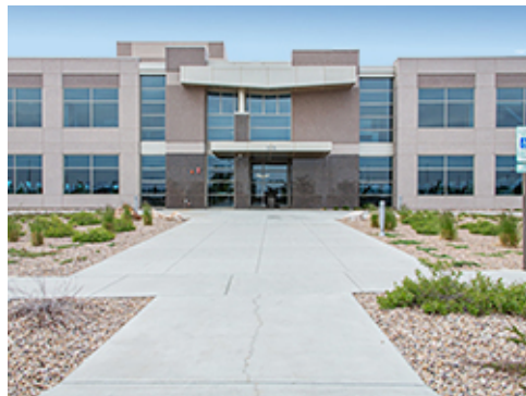
Concrete Entrance Plaza
