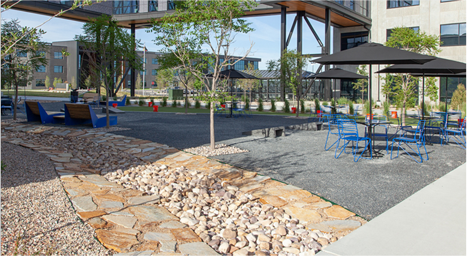
Stormwater Swale Designed as an Amenity
