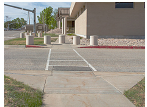
Curb Ramp at Intersection
