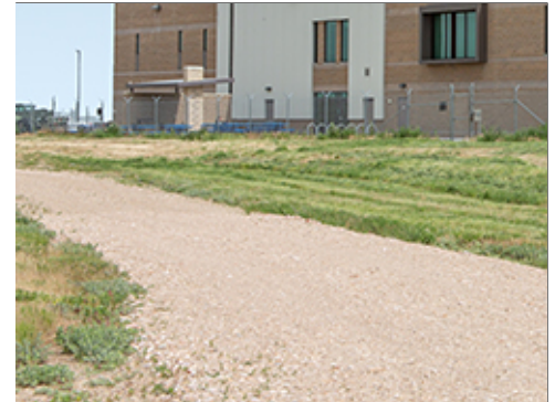
Gravel Paving at Limited Access Area
