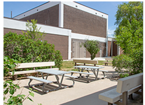
Group 2 Gathering Area with Concrete Paving
