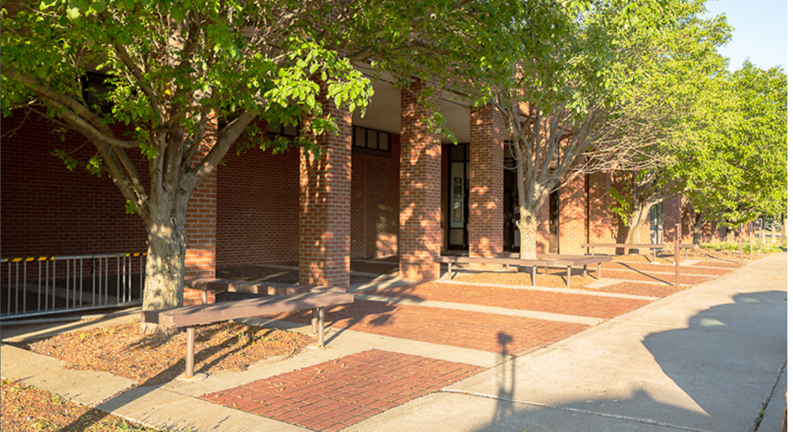
Concrete Paving with Inset Brick Pavers at Group 2
