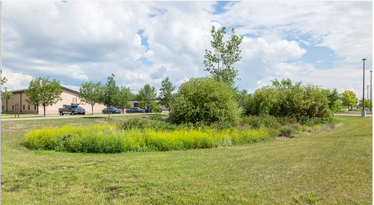
Vegetated Detention Basin
