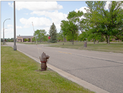
Hydrant with Locator Mast
