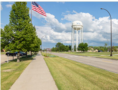
Concrete Paving along Special Route
