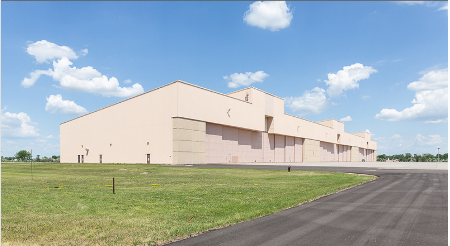
Facility Group 3 Hangar
