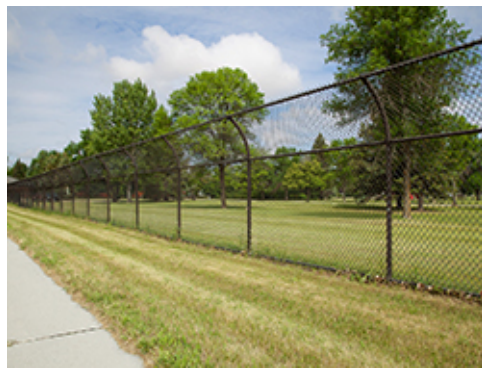
Chain Link Fencing at Group 3
