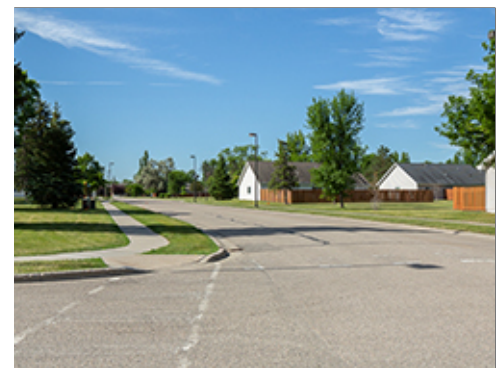
Typical Local Street at Group 4
