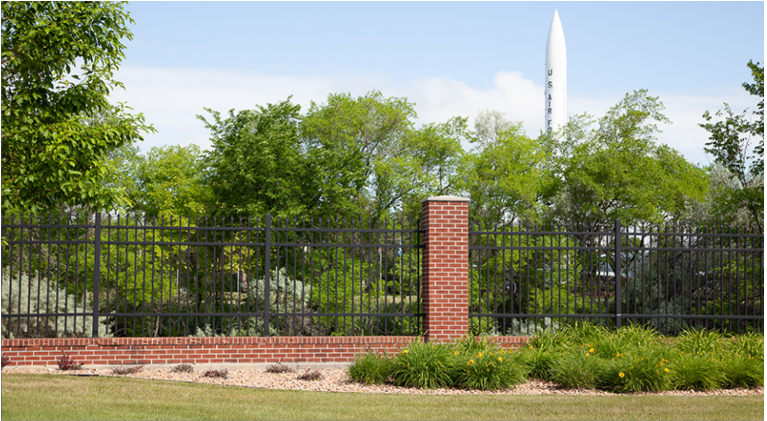
Masonry Piers and Metal Post, Rail and Picket Fencing at Group 1
