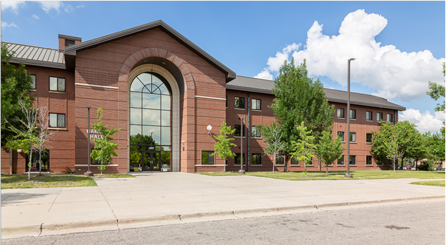
Pedestrian Scaled Fixtures near Entrance Parking Scaled Fixture near Access Drive
