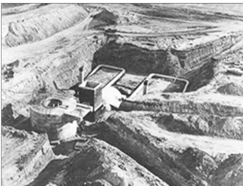
Launch Facility Grand Forks AFB c. 1965
