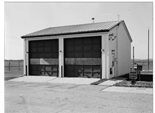
Grand Forks AFB Missile Alert Storage Facility
