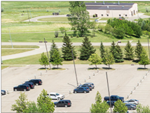
Access to Parking
