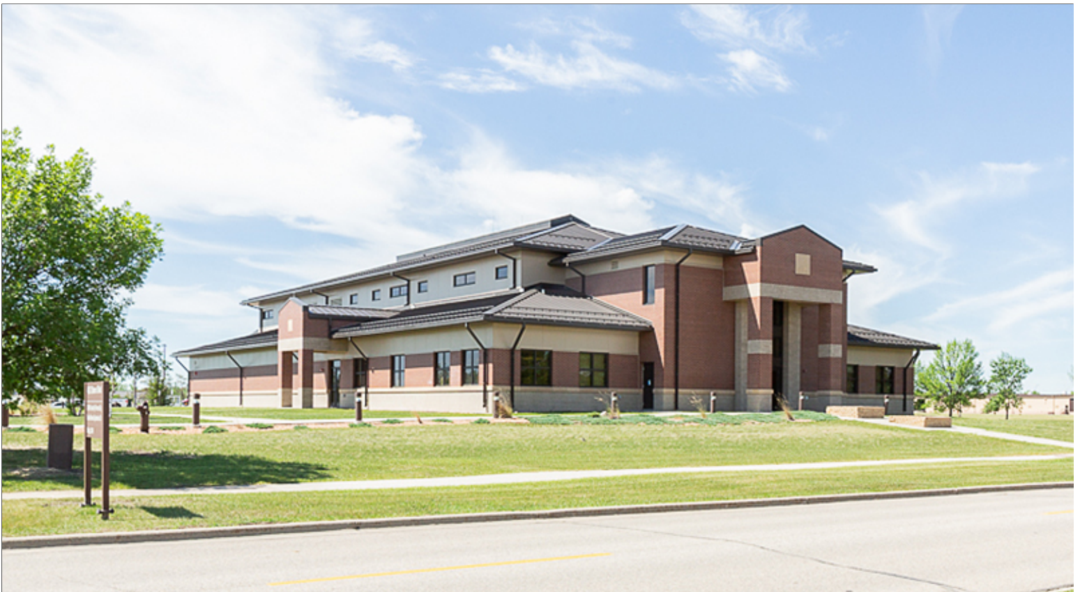
Overhangs Providing Shading near Summer
