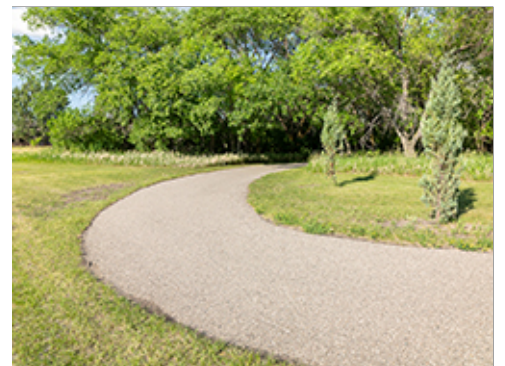
Bituminous Paving at Trail
