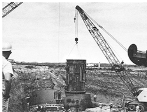
Equipment Room Liner Installation
