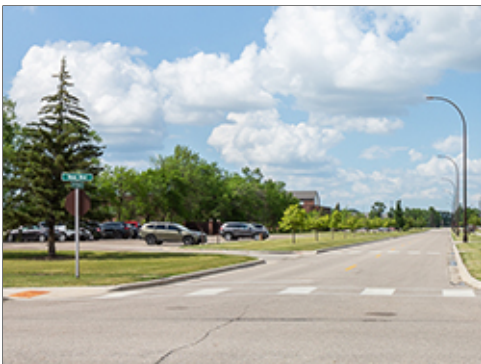
Intersection at Group 2
