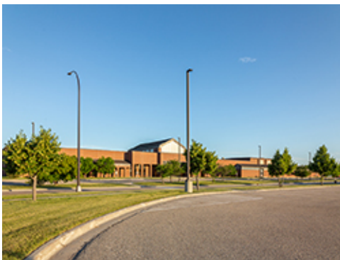
Underground Utility Service Lines
