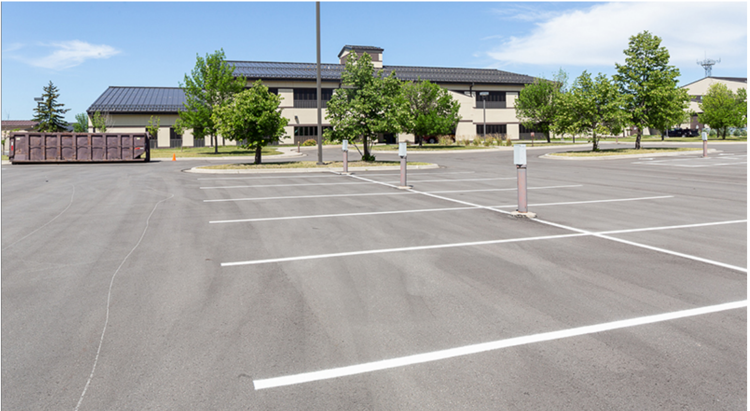
Bituminous Paving with Standard White Striping
