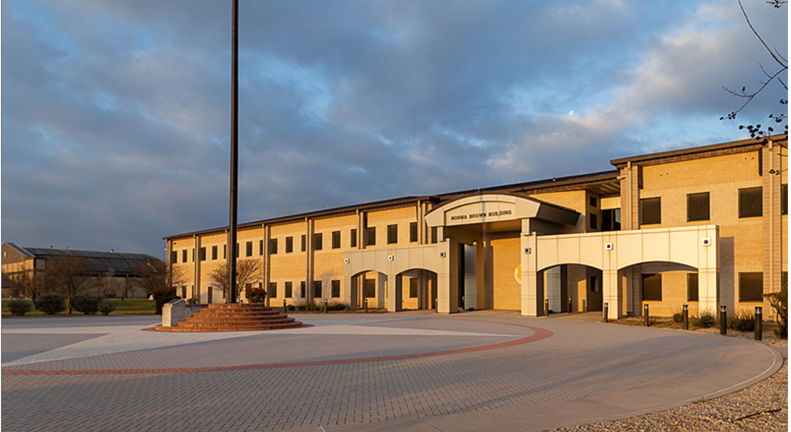
Decorative Patterns with Unit Pavers at Group 1
