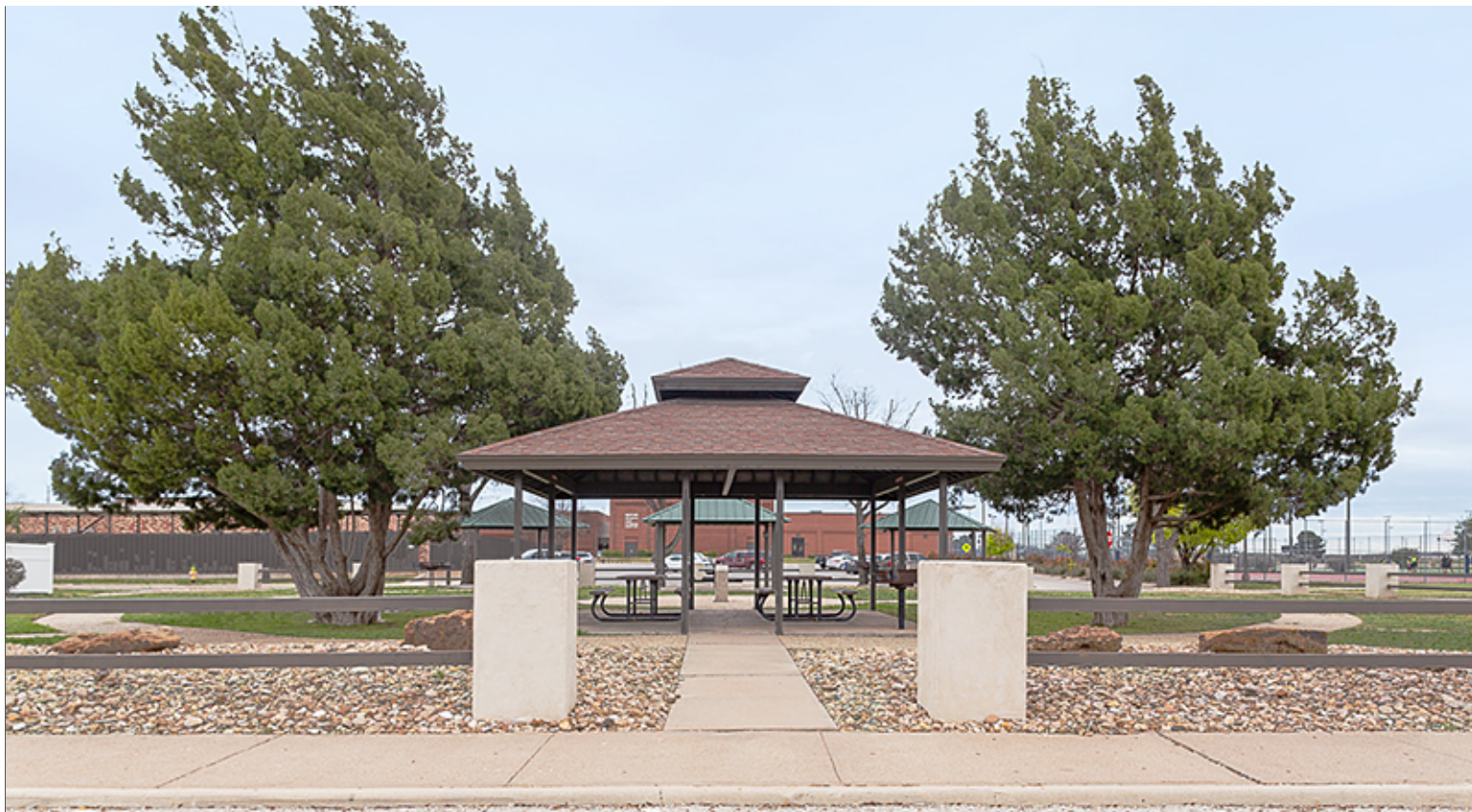
Piers and Fence Defining space and Entrance
