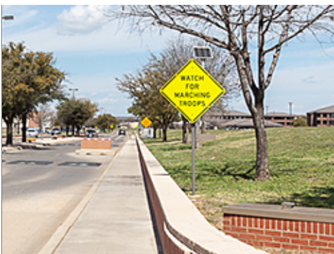
UFC Compliant Sign
