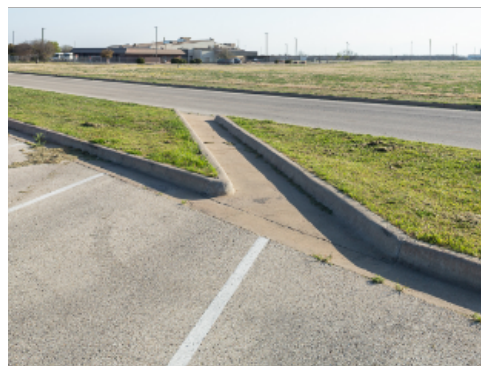
Channel for Stormwater
