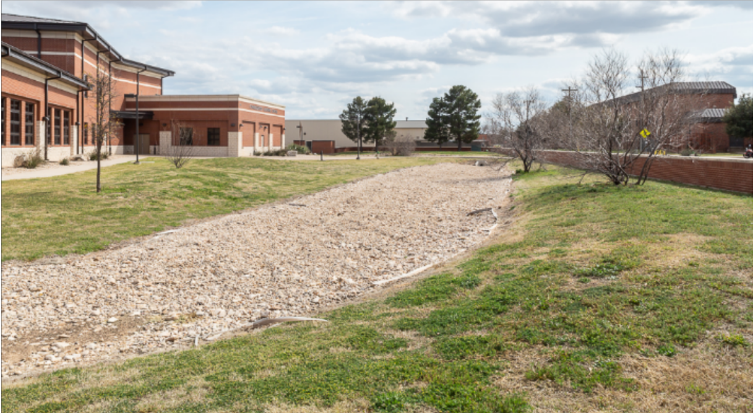
Integrated On-Site Drainage and Percolation Feature
