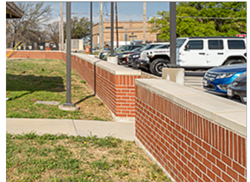
Screen Wall Defining Access
