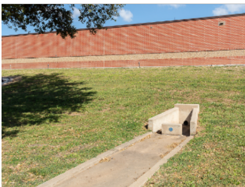
Outlet to Paved Basin
