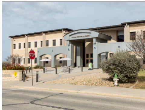
Lightd Bollards along Sidewalk
