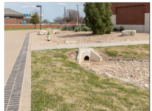
Outlet to Rip-Rap Basin
