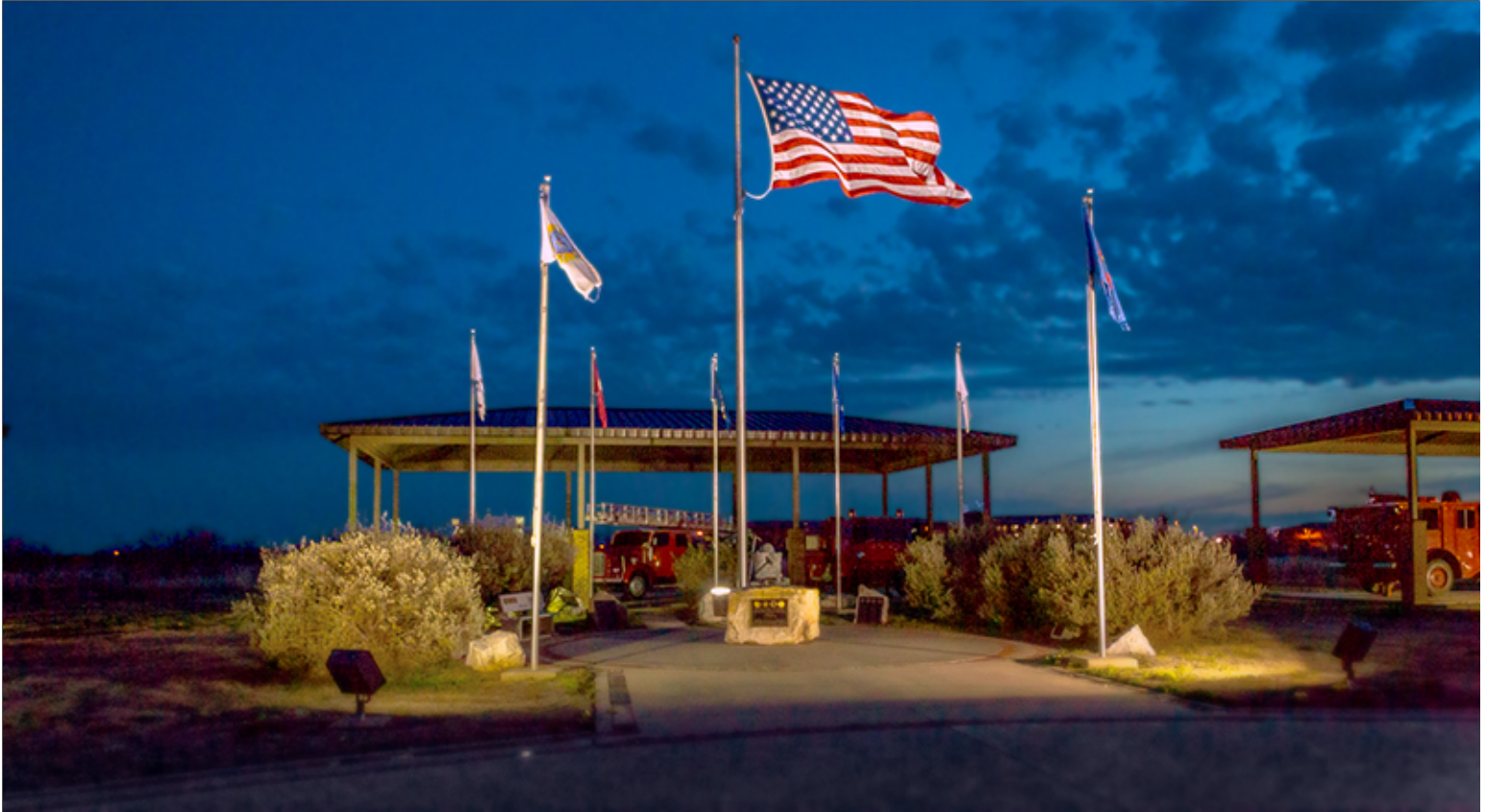
Indirect Lighting for Sidewalks and Plaza
