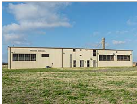
Group 3 Industrial Facility
