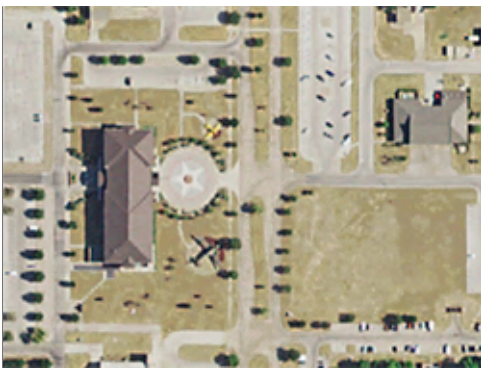
Intersection at Group 1 Plaza
