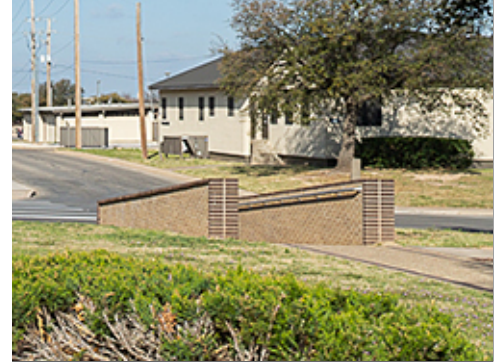
Masonry Walls at Site Ramp
