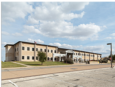
Special Paving along Group 1
