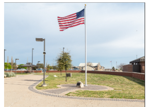
Exposed Aggregate Concrete and Pavers
