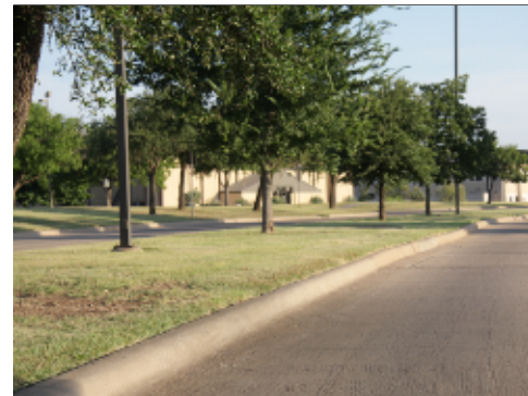
Integral Curb and Gutter at Median
