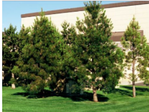
Utility components hidden by vegetation
