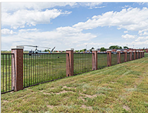
Brick and Metal Fence
