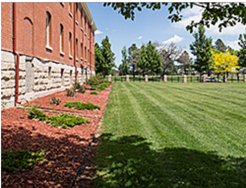
Minimizing Water at Foundations
