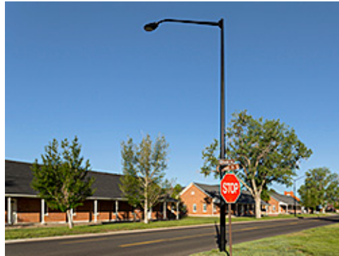
Standard Street Light Fixture
