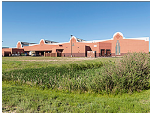
On-Site Stormwater Detention Area
