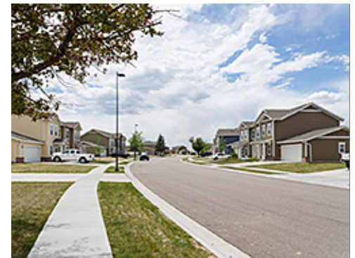
Local Street with Detached Sidewalk
