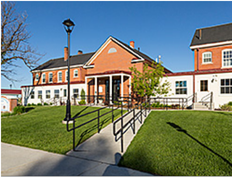
Ramp along Accessible Route
