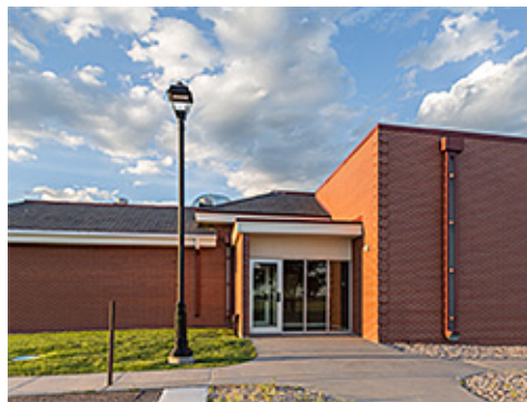
Pedestrian Lighting at Entrance
