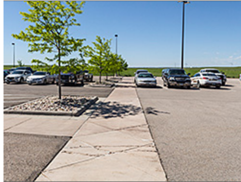
Contrasting Pavement Defining Path
