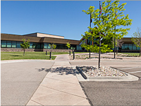
Link to Main Entrance
