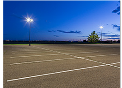
Parking Lot Lighting
