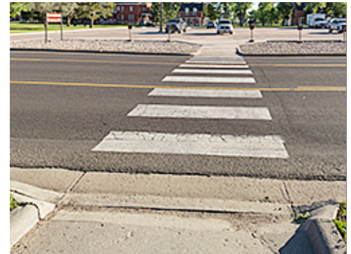
Integrated Curb Ramp
