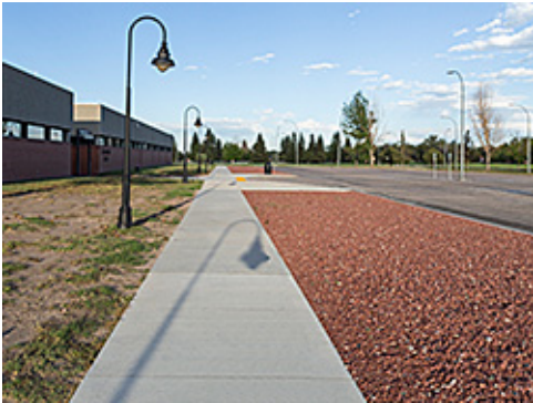
Pedestrian Scale Light Fixture
