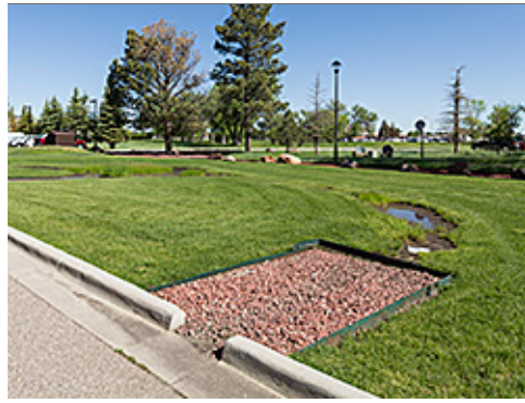
Rock Filtration Area
