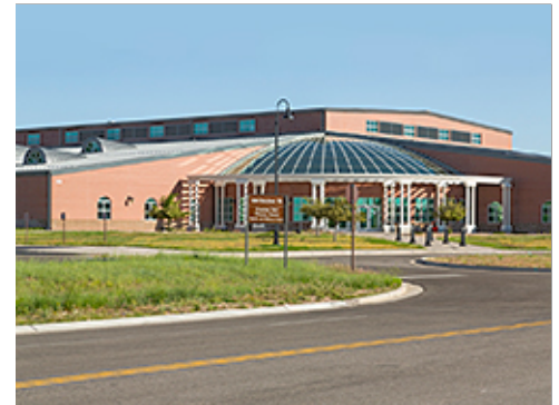
Contrasting Color at Main Entrance
