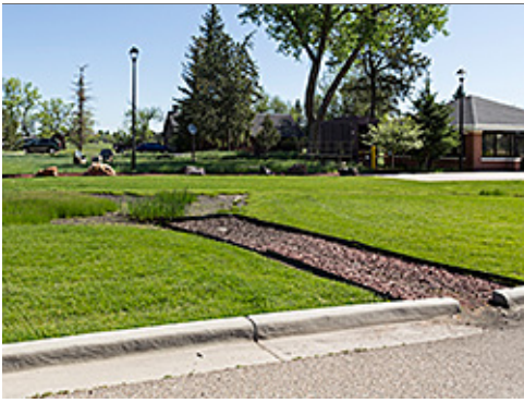
Parking Lot Stormwater Discharge Inlet
