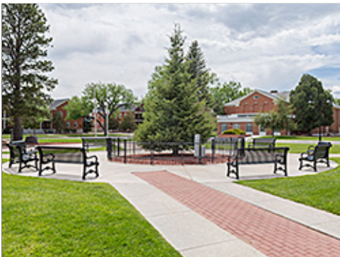
Concrete with Brick Accent Pavers
