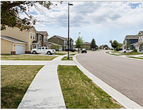
Detached Sidewalk in Group 4
