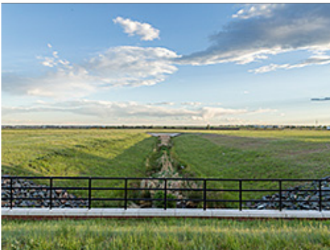
Base-wide Scale Stormwater Feature
