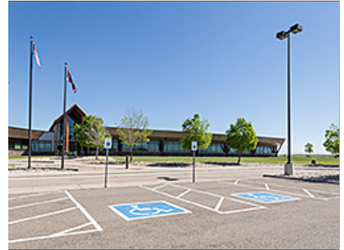
Adjacent Accessible Parking
