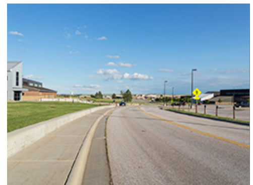
Integrated Sidewalk and Retaining Wall
