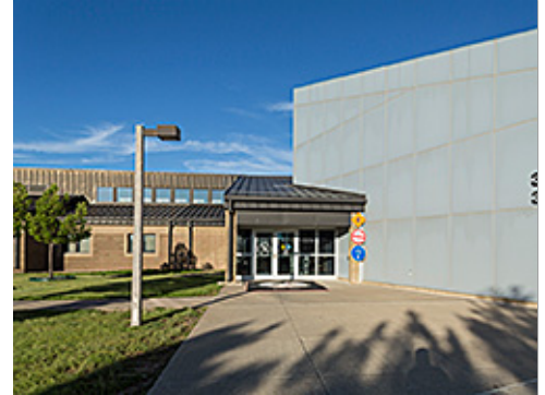
Pedestrian Circulation Lighting
