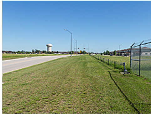
Remote Area Chain Link and Cable Fencing
