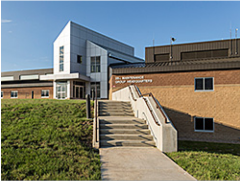
Main Entrance Stair
