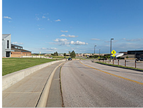
Attached Sidewalk and Retaining Wall
