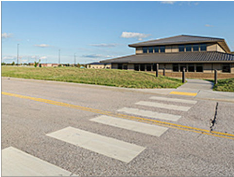
Standard Crosswalk Striping
