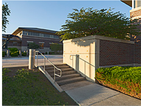
Site Stair at Group 1
