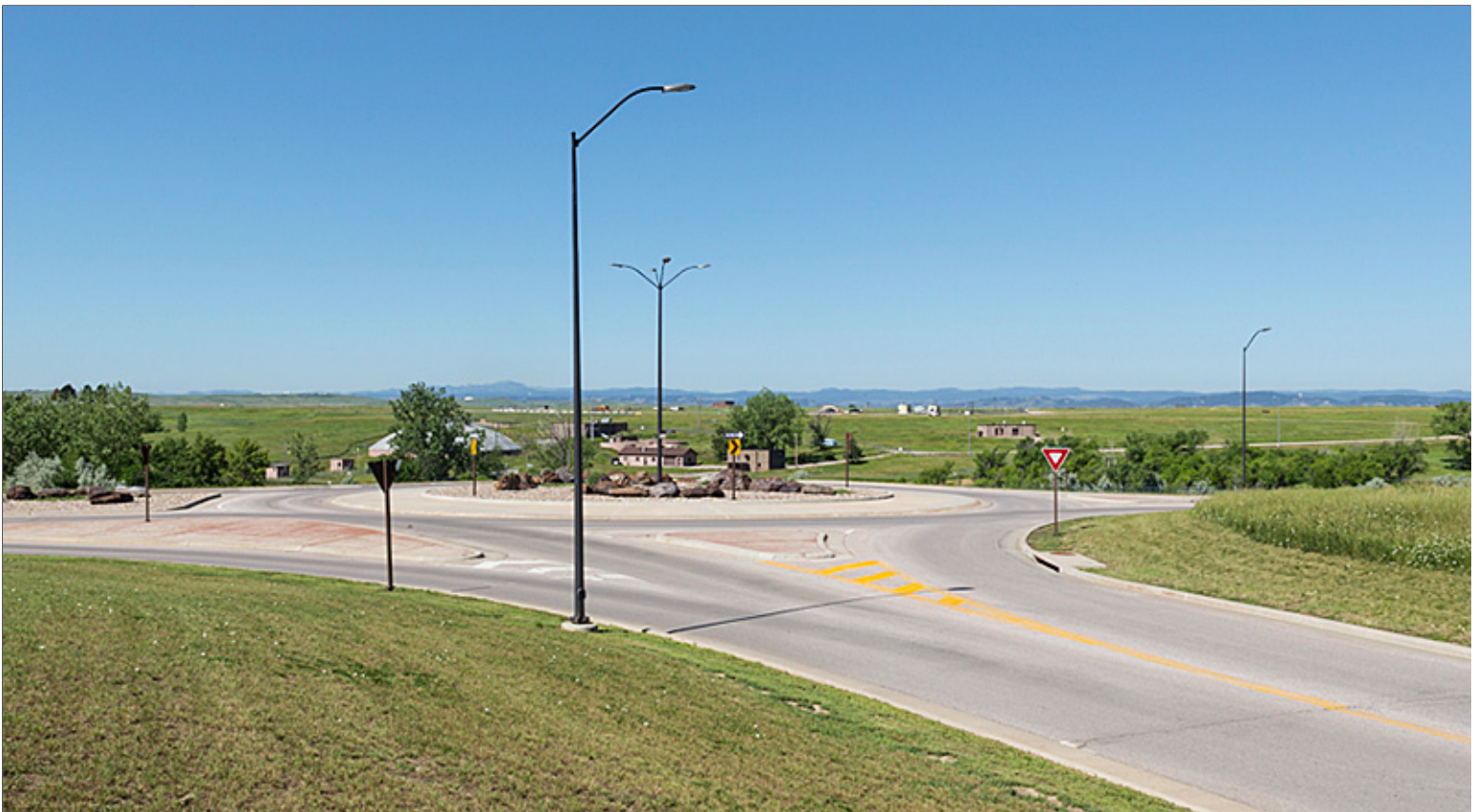
Passive Systems: Traffic Circle with Low Maintenance Xeric Landscape Features
