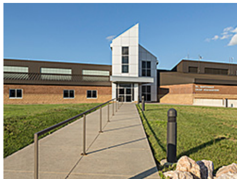
Bollards and Railings at Entrance
