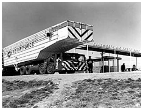
Transporter Erector at Ellsworth AFB, c. 1963
