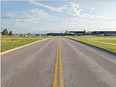
Asphaltic Concrete Paving
