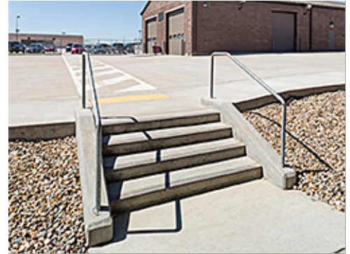
Site Stair at Group 3
