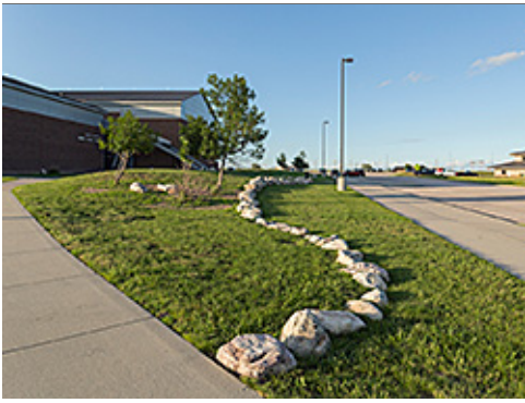
Rock Retaining Wall
