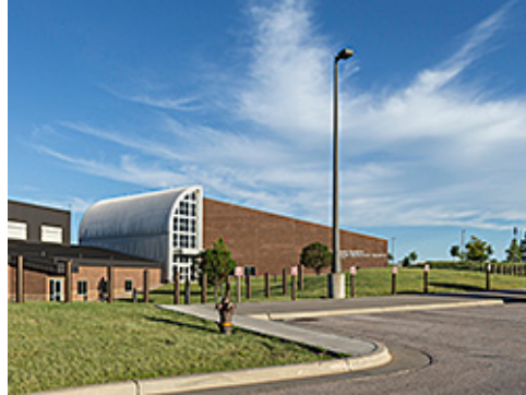
Parking Lot Lighting
