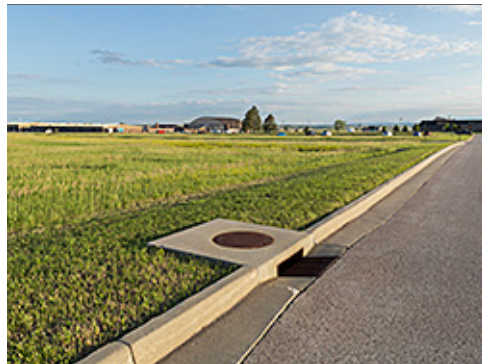
Roadway Catch Basin
