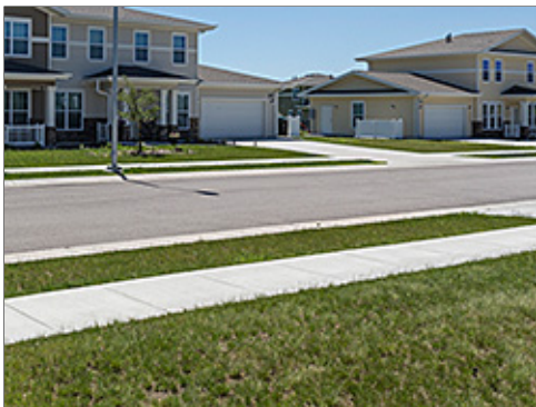
Residential Scale and Detailing
