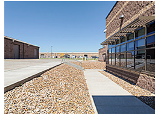
Rock Mulch at Group 3
