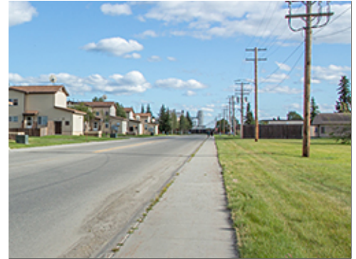
Above Grade Utility Service
