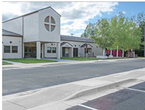
Asphalt Paving at Group 2
