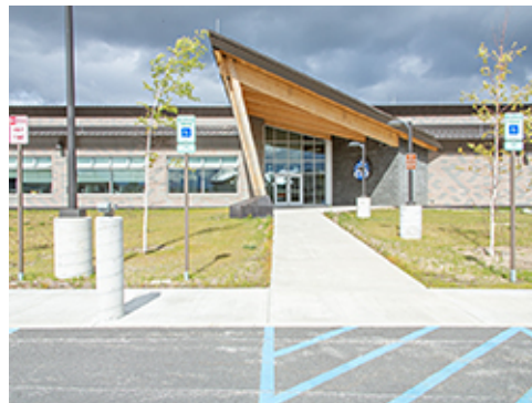
Zero Curb with Grade to Accommodate Slope
