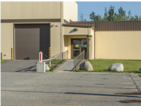
Site Ramp at Entrance
