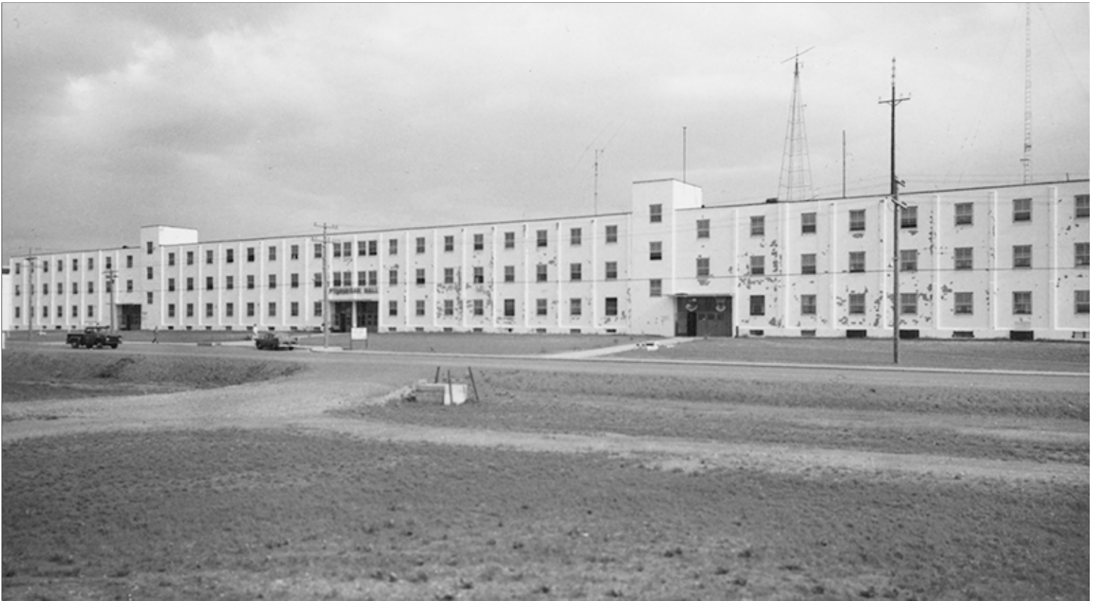
Ptarmigan Hall, c. 1962, Airmen Dormitory Converted to Wing Headquarters in 1972
