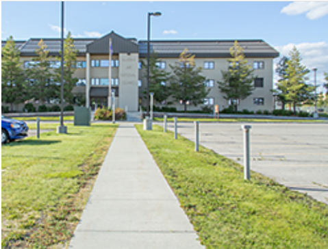
Axial Approach to Main Entrance
