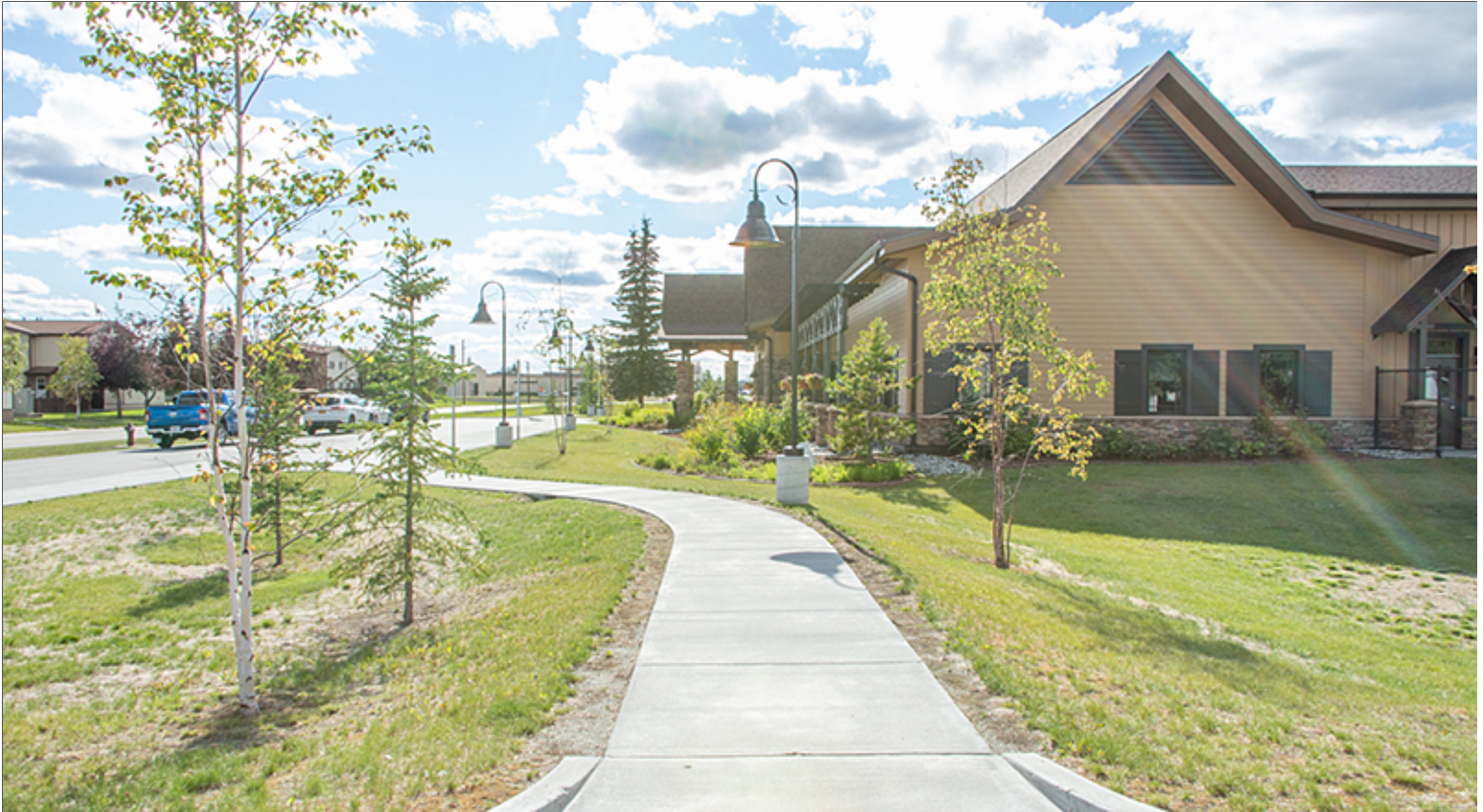
Concrete Sidewalk at Group 2
