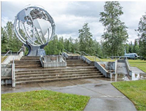
Concrete Paving at Plaza, Stairs and Ramps
