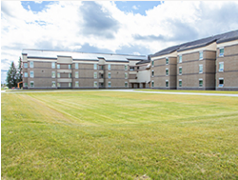
Detention Basin as an Amenity
