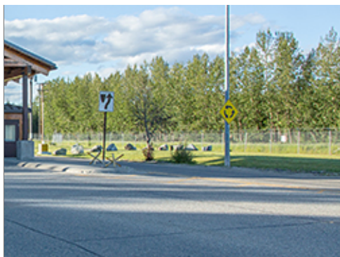
Perimeter Fencing Adjacent to Main Gate
