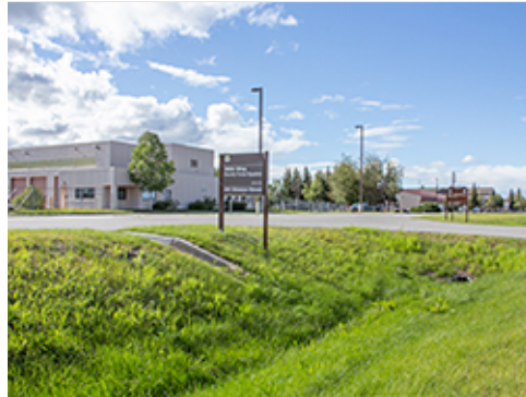
Vegetated Swale along Street
