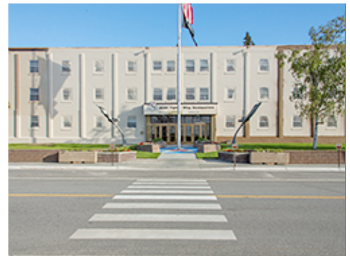
Decorative Paving at Group 1 Entrance Plaza
