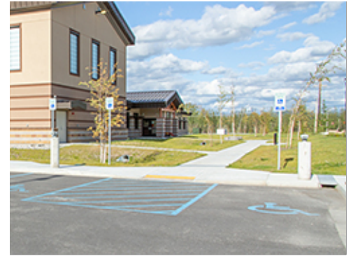
Link from Parking to Main Entrance
