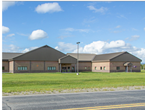
Gabled Roof with Metal Clad Endwall
