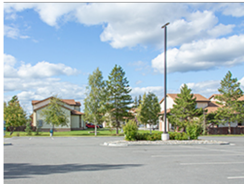
Coordinated Placement of Light Fixture
