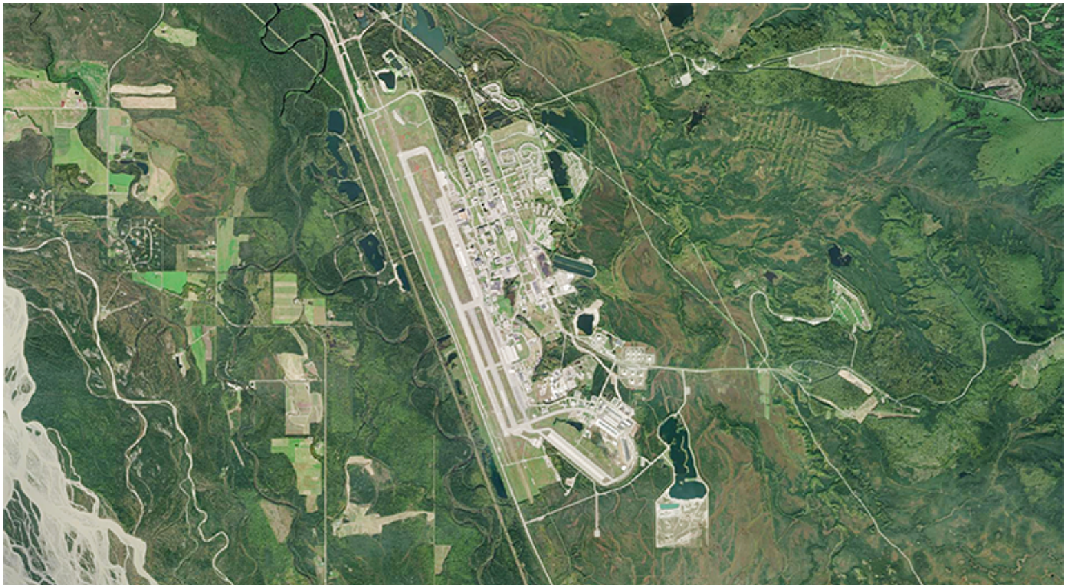
Aerial Image of Eielson AFB
