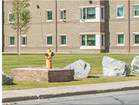
Hydrant with Protective Plinth
