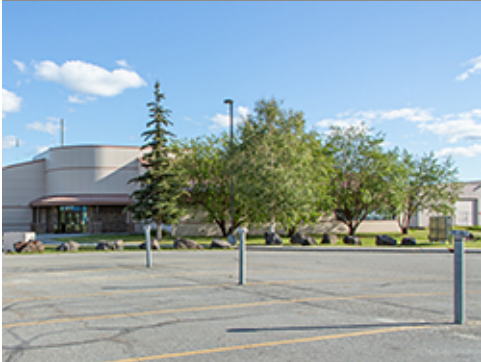
Planting at Perimeter of Parking Lot
