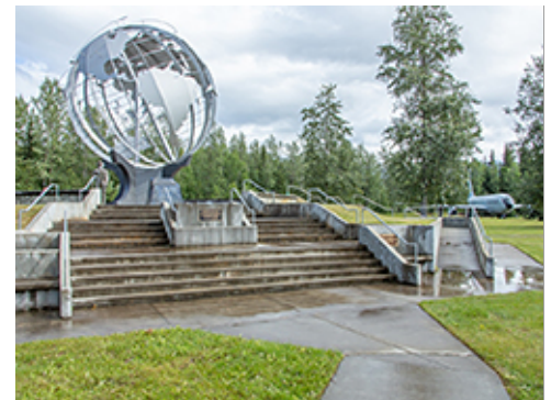
Stair with Integrated Ramp
