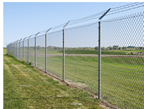
Typical Chain Link Fencing
