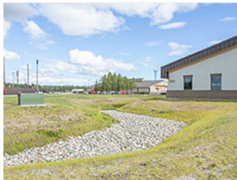
Swale with Rip Rap
