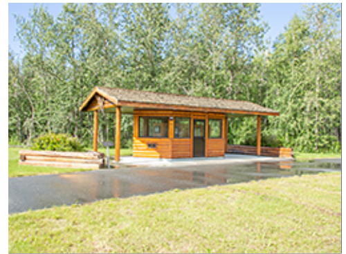
Concrete Paving at Pavilion
