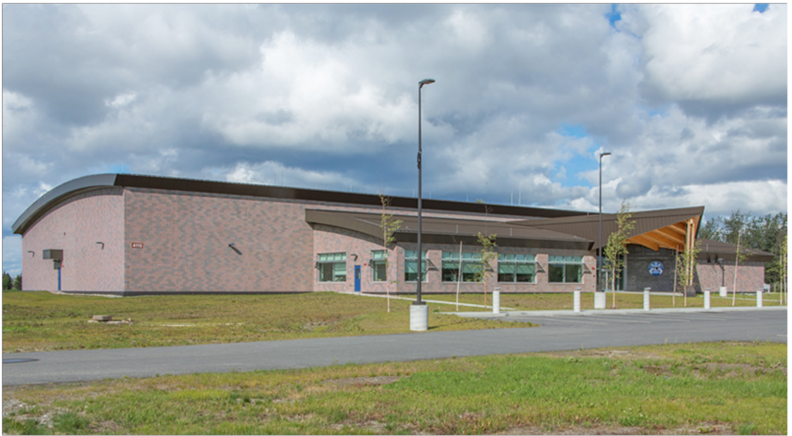
Predominant Use of Concrete Masonry Units (CMU) at Group 2 Facility
