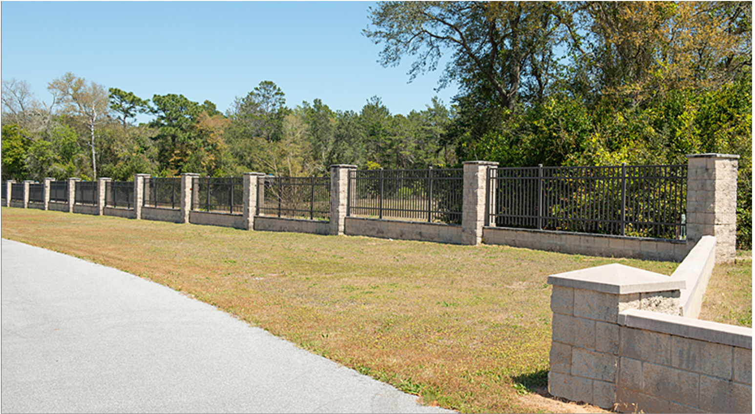
Group 1, Main Gate Fence: Metal Railing Supported by CMU Piers and Low Walls with Architectural Precast Caps and Coping
