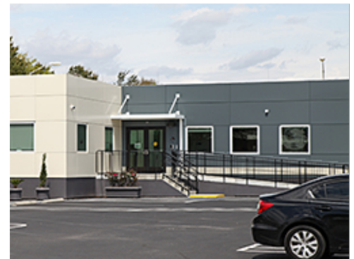
Building Stair and Ramp
