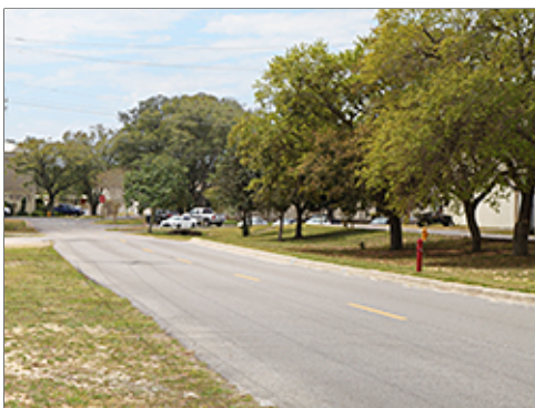
Local Street in Group 3
