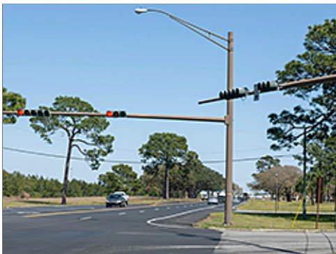
Street Lighting Combined with Signal Pole
