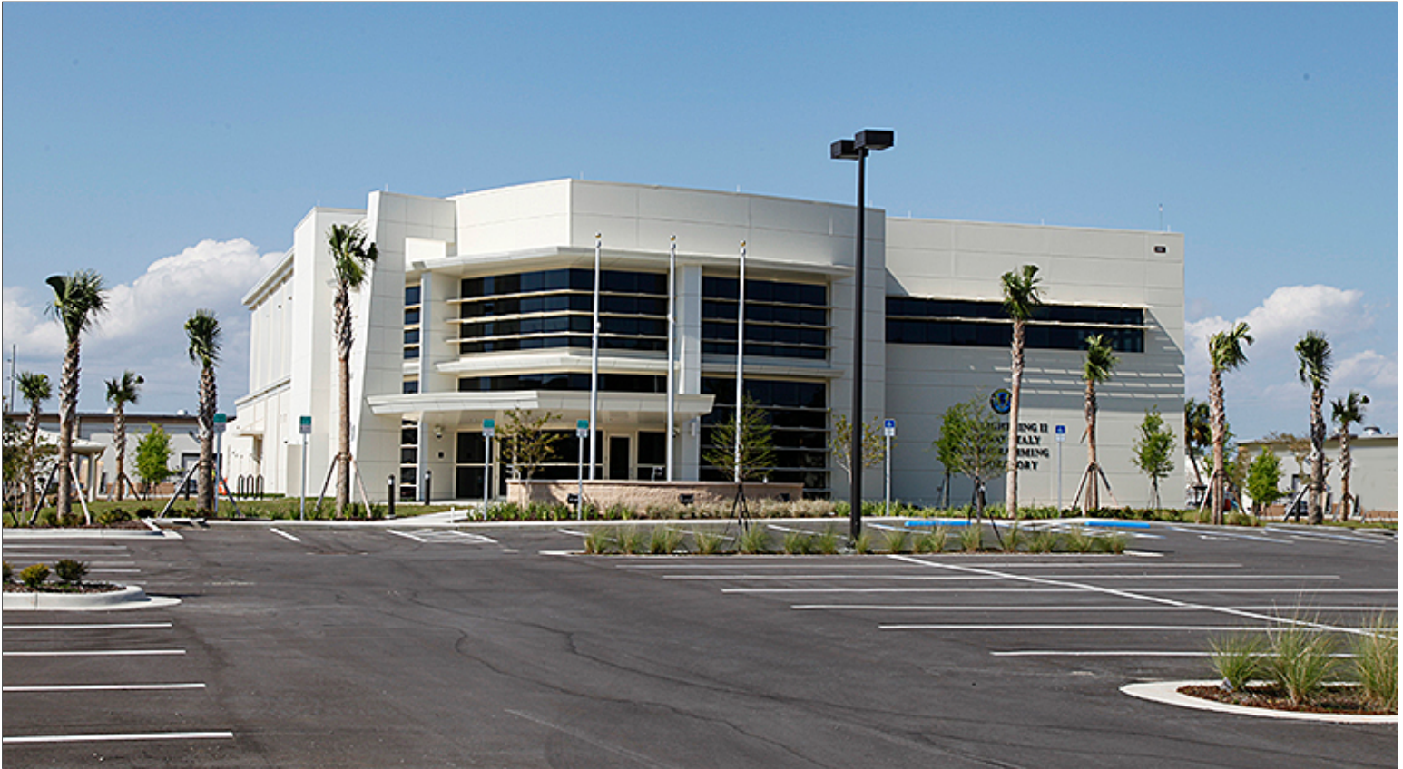
South Facing Exposure with Fixed Shading Devices to Reduce Solar Heat Gain
