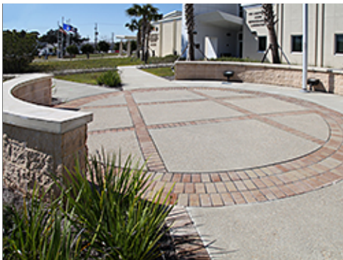
Decorative Paving at Group 2
