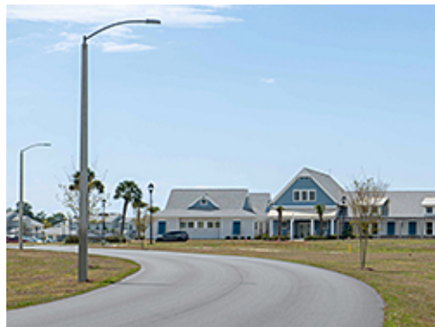
Collector Lighting in Group 4
