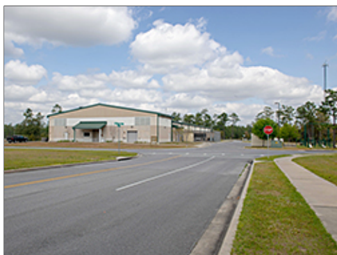
Intersection at Group 3
