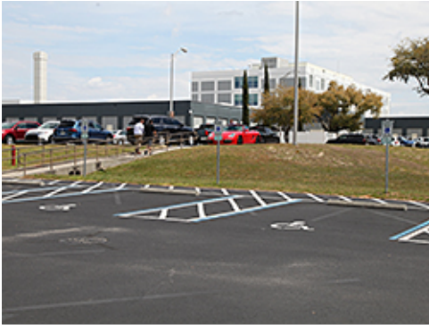
White with Blue Striping at Accessible Spaces
