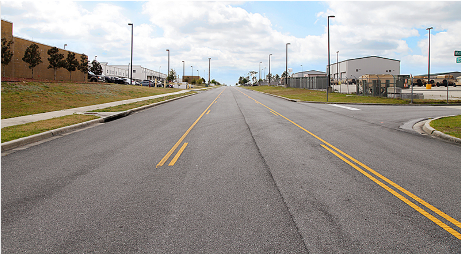
Striped Center Turn Lane at T Intersection
