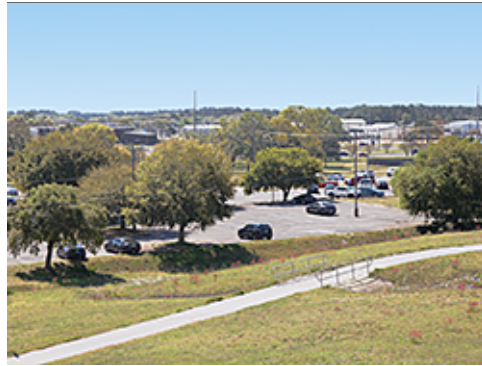
On-Site Stormwater Swale and Detention
