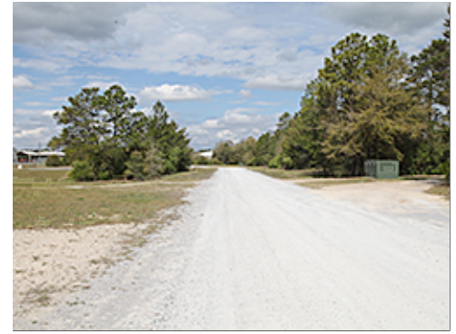
Gravel Paving in Utility Area
