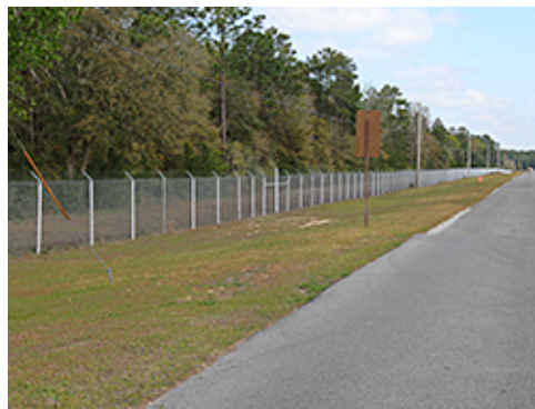
Remote Site Chain Link Fencing
