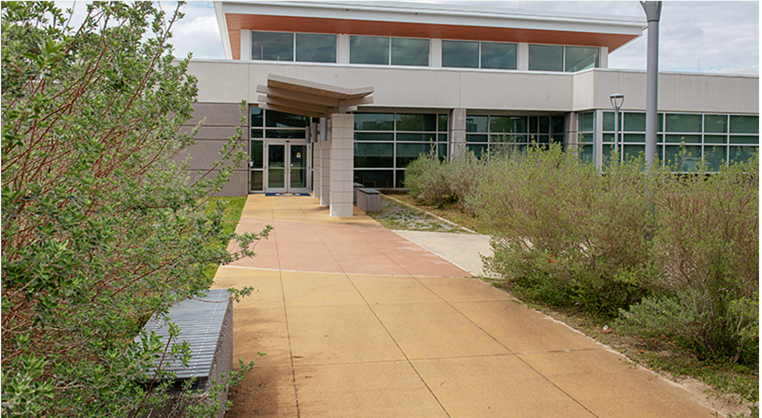
Integrally Colored Concrete Sidewalk at Entrance to Group 1 Facility
