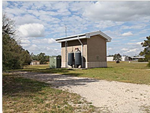
Compatible Utility Structure
