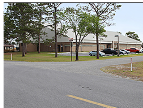
Intersection at Local Street
