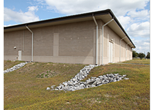
Rip Rap at Downspout Outflow Area
