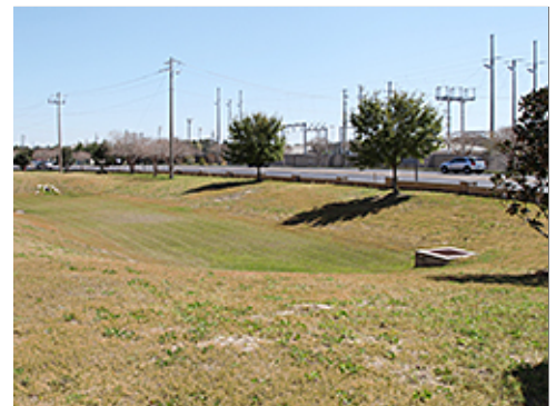
Storm Drainage Basin Adjacent to Street
