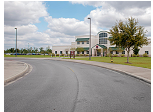
Street Adjacent to Group 1 Facility
