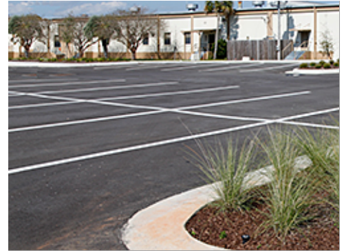
Typical Asphaltic Concrete Paving
