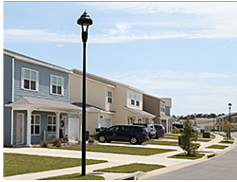
Street Lighting in Group 4
