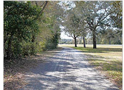
Rock Paving on Remote Access Road
