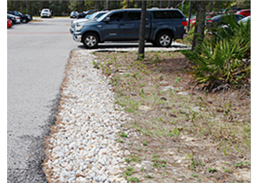
Compacted Rock Mulch as Header Curbing
