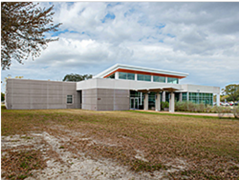
Group 1 Clerestory Lighting as a Feature
