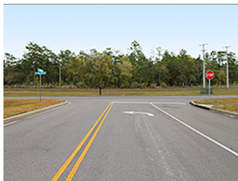
T Intersection with Center Turn lane
