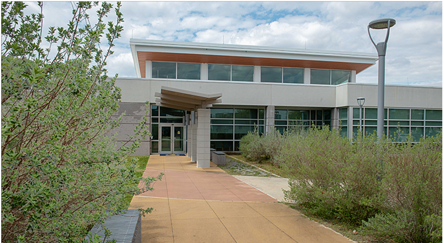
Indirect Lighting Fixture at Group 1
