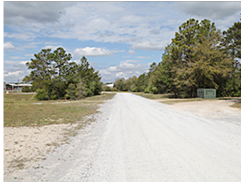
Gravel Paving on Utility Road
