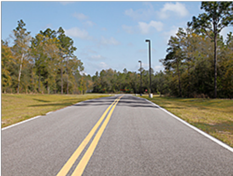
Typical Asphaltic Concrete Paving
